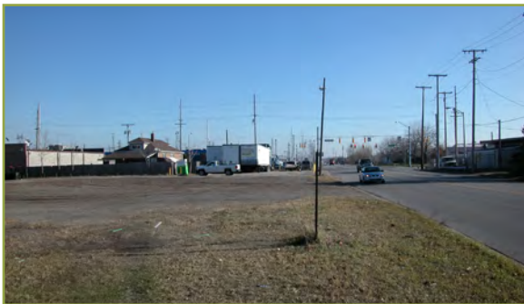
INCOMPLETE SIDEWALK NETWORK ON MICHIGAN STREET
