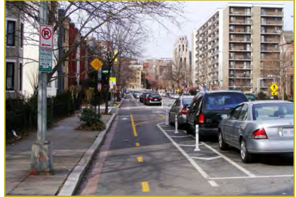
CYCLE TRACK, SEPERATING PEDESTRIANS AND BICYCLES FROM TRAFFIC
