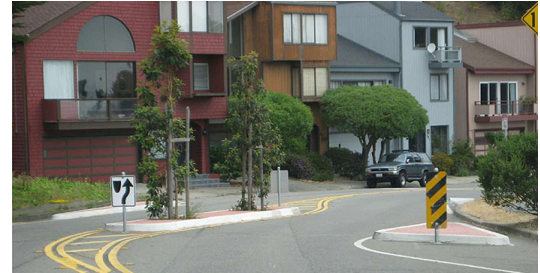
Chicane in a residential area.
