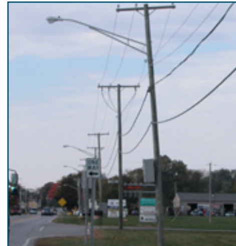
TYPICAL STREET LIGHTS
