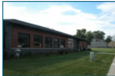
NEWER COMMERCIAL BUILDING
