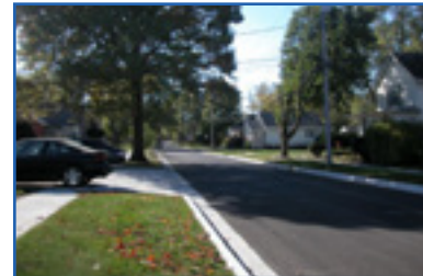
NEWER STREETS INCLUDE CURB AND GUTTER FOR STORM WATER DRAINAGE
