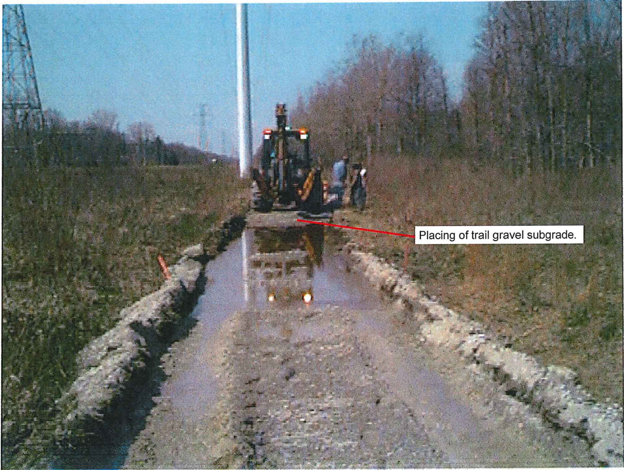
April 10, 2002 Construction Photo
