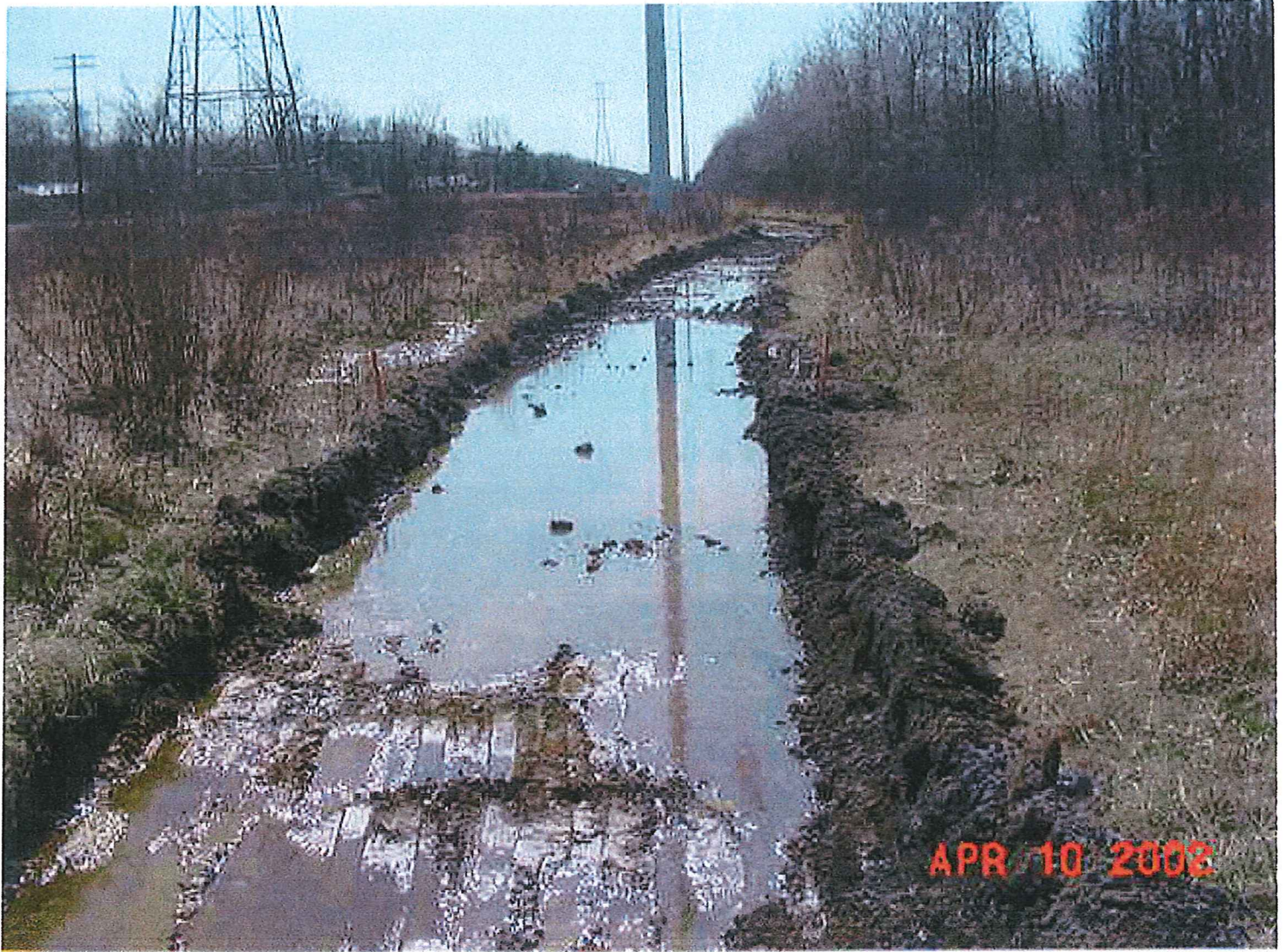
April 10, 2002 Construction Photo
