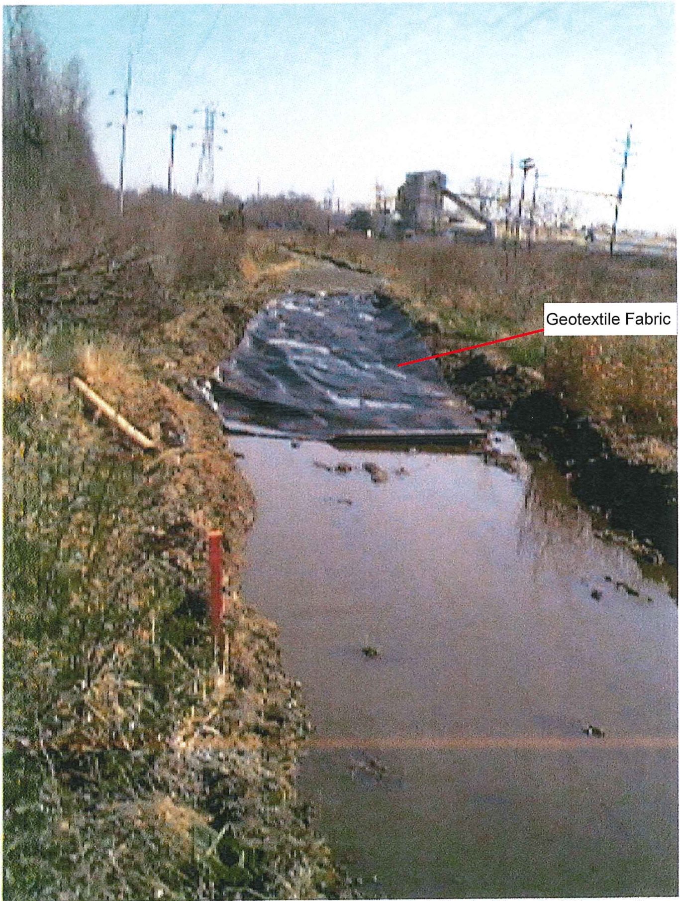
April 10, 2002 Construction Photo
