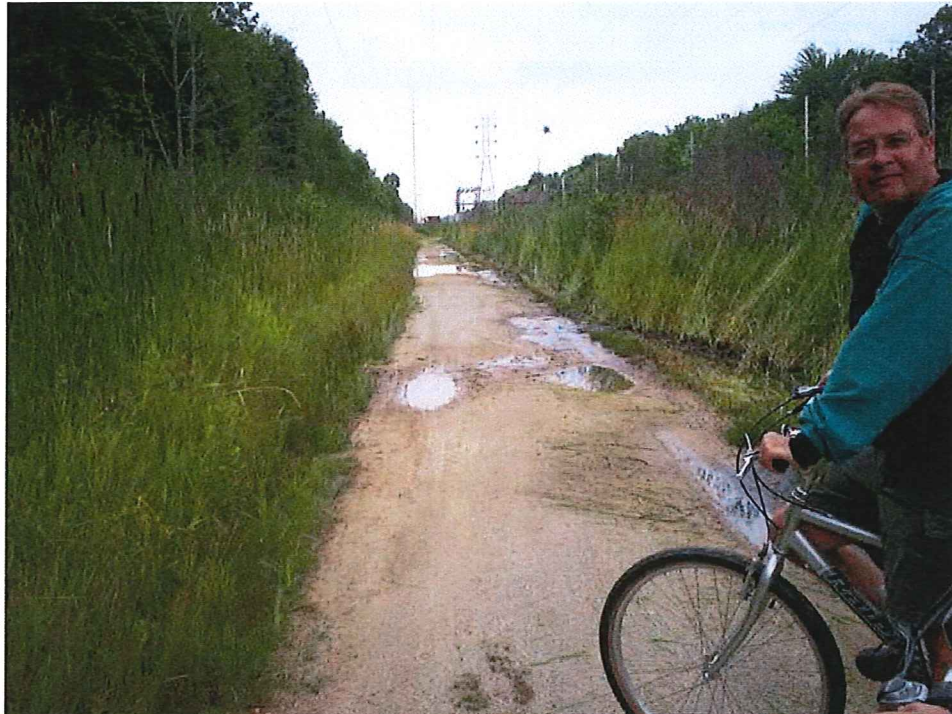
Photo 3 Existing trail is nearly impassable in low lying areas. (Photo July 8, 2009)
