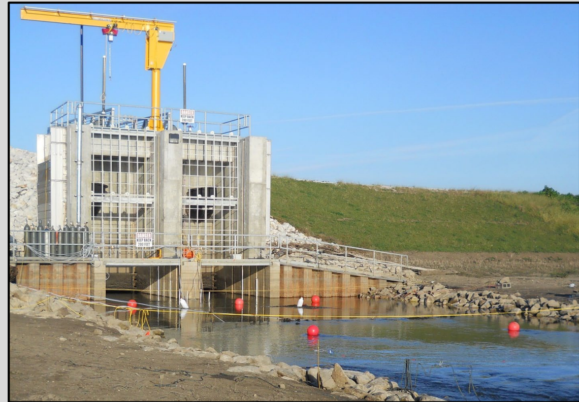
Carbon dioxide treatments at a water control structure on the Illinois River (Lewistown, IL)
