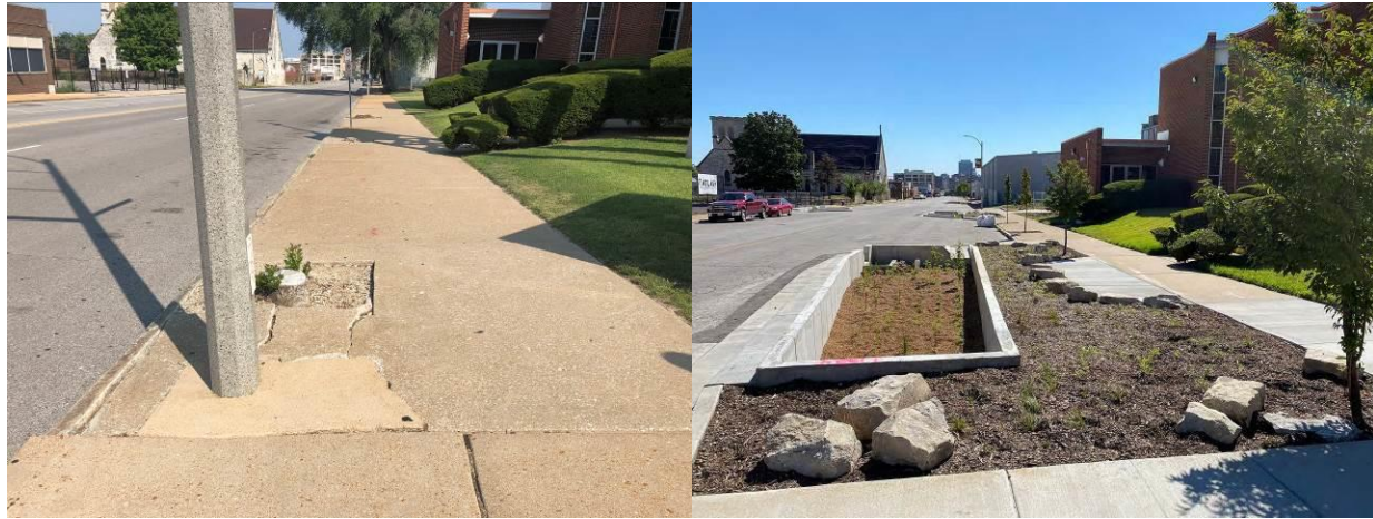
Before (picture on the left) and after (picture on the right) comparison of bioinfiltration being installed as traffic control, reducing a four-lane road down to a two-lane road – Principal and Minor Arterial Roads.
