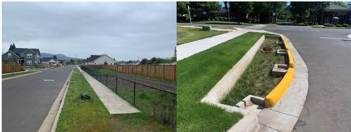
Examples of bioinfiltration facilities installed along roadways (Collector and Local Roads) as either a larger stormwater management feature (picture on the left) or a smaller, distributed stormwater management features (picture on the right).
