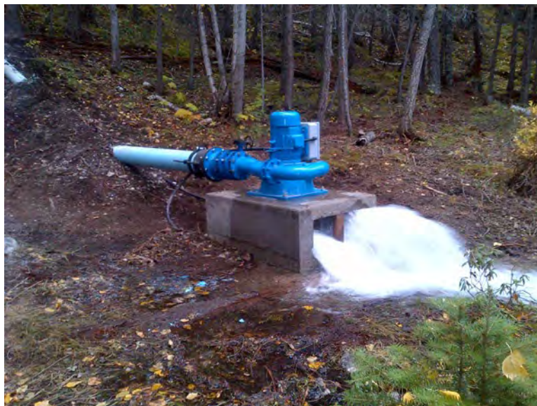
Figure 7-4: Micro hydropower facility (Source: Suneco Green Energy [8])
