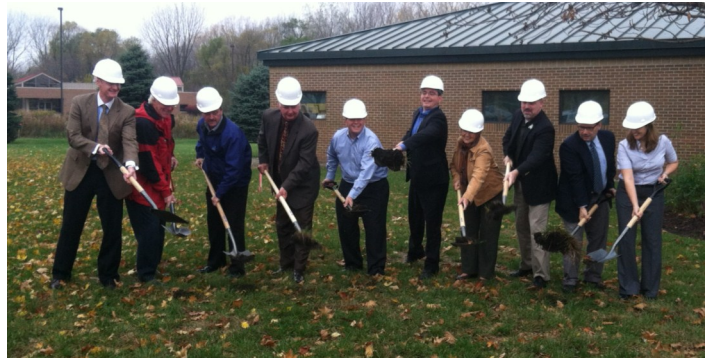
The first shovelfuls of dirt are thrown at the groundbreaking for the Northside Trail at NIRPC on October 23, 2012.
