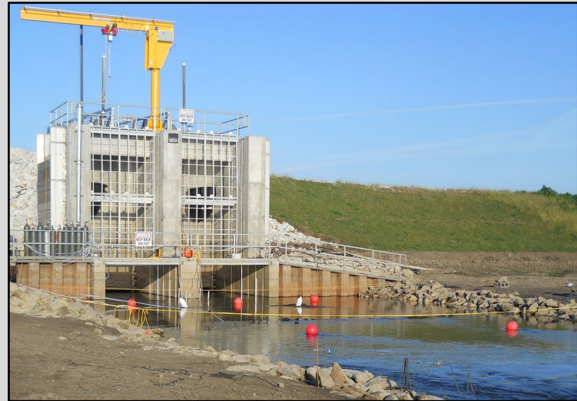
Carbon dioxide treatments at a water control structure on the Illinois River (Lewistown, IL)
