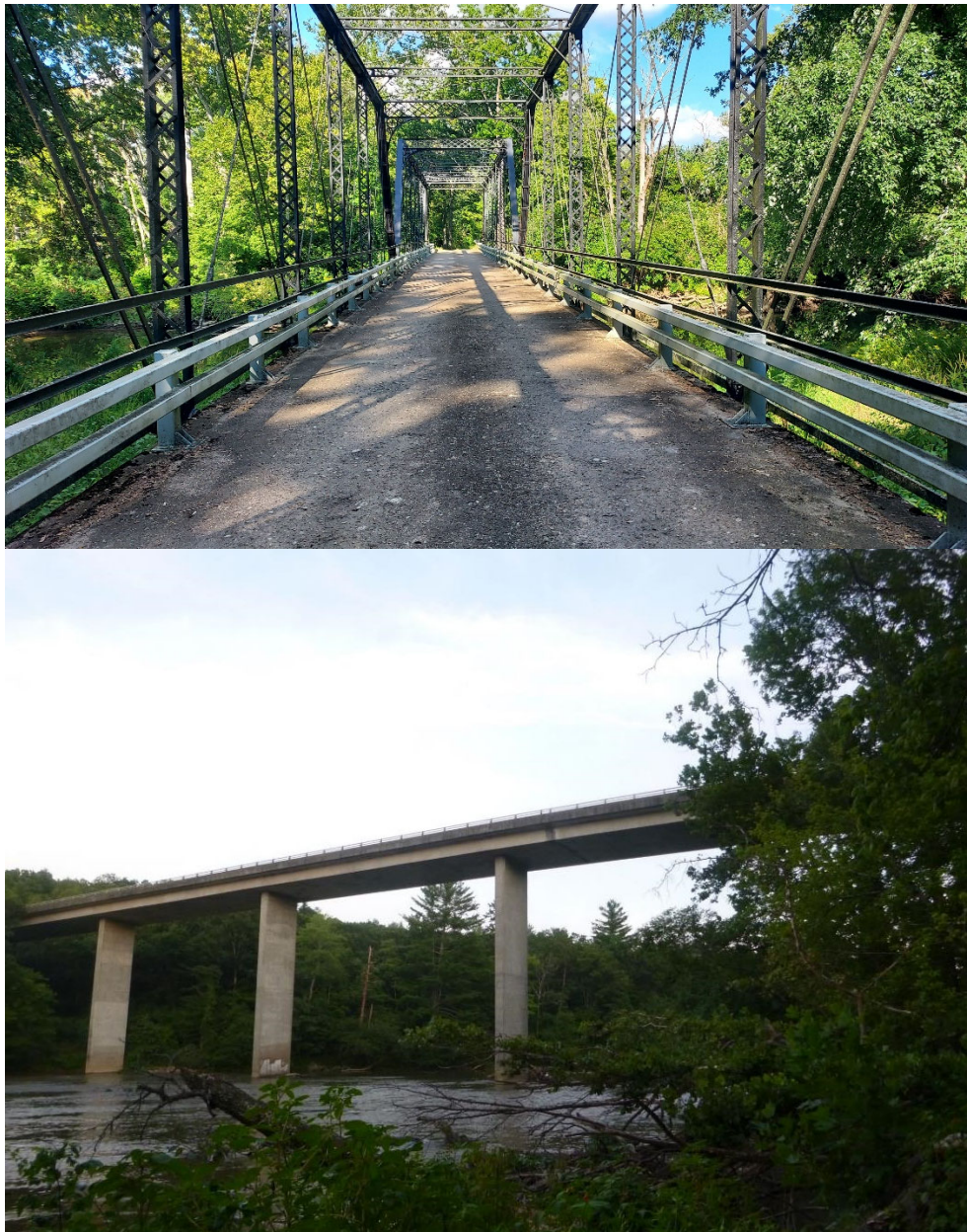
FIGURE 9. Representative bridges with documented bat use, including a bridge with metal struts in Indiana (top; photo provided by Indiana Department of Transportation) and a concrete bridge in North Carolina (bottom; photo provided by North Carolina Wildlife Resources Commission).
