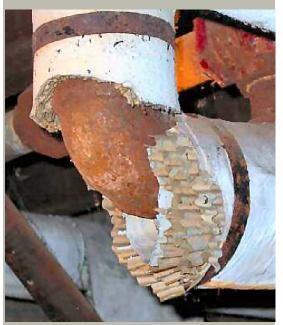
Damaged asbestos pipe insulation.
