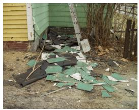
Improperly removed asbestos from home renovation project.
