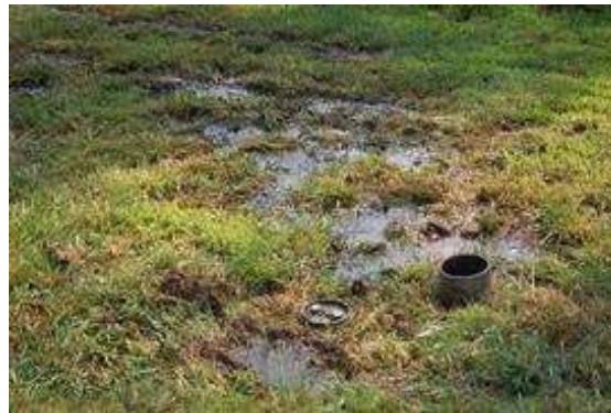
Over-saturated drain field (Photo from www.DennisDiffley.com )
