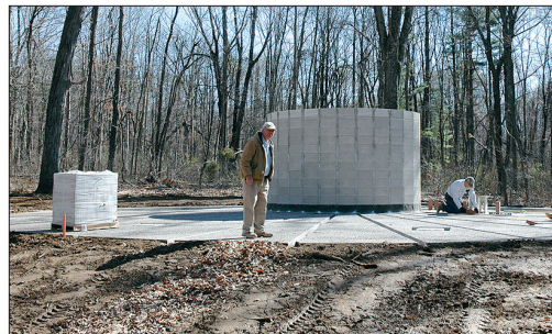
The Plaza early in the construction process.
