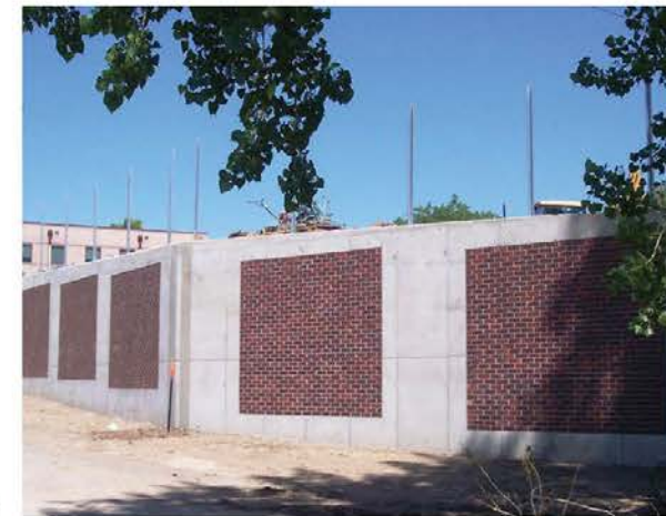
Snap brick retaining wall ▶
