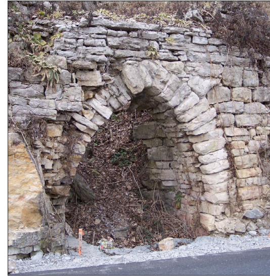
Detail of stone arch
