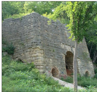
Carlson's Lime Kiln at Barn Bluff Park
