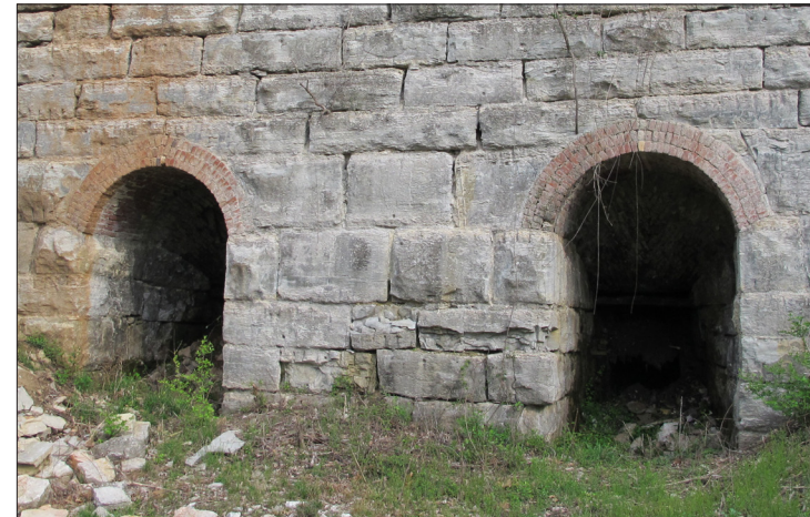
Perpetual Kiln 48003 arched openings
