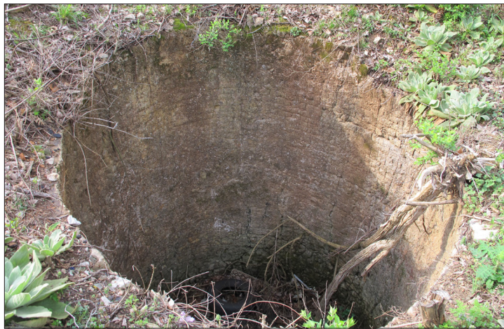
Original shaft opening at Kiln 48003
