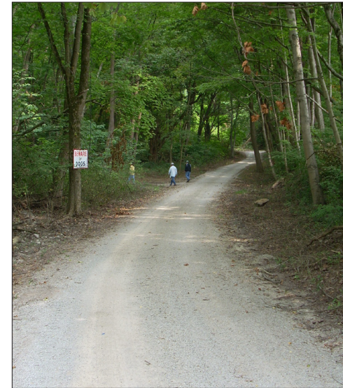
Construction / access road near Kiln 48003
