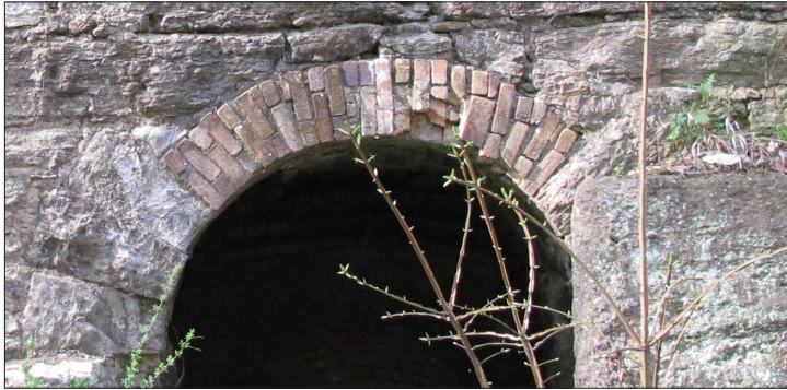
Brick repairs at arch
