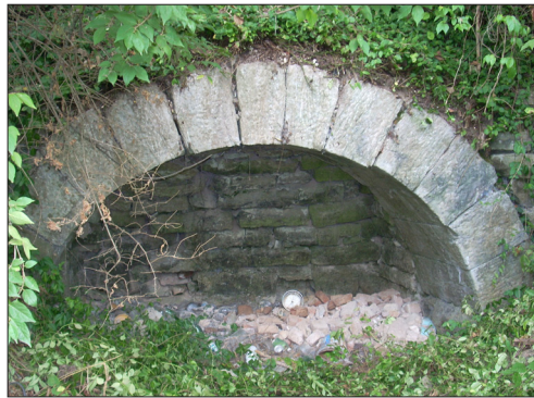
Stone arch opening at Kiln 48001
