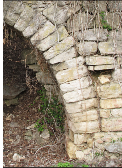
Detail of stone arch
