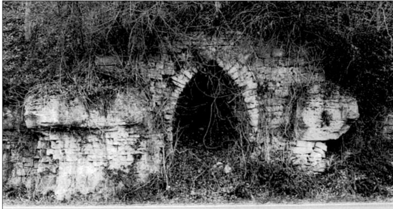
Condition of Kiln prior to roadway construction (photo ca. 1995)
