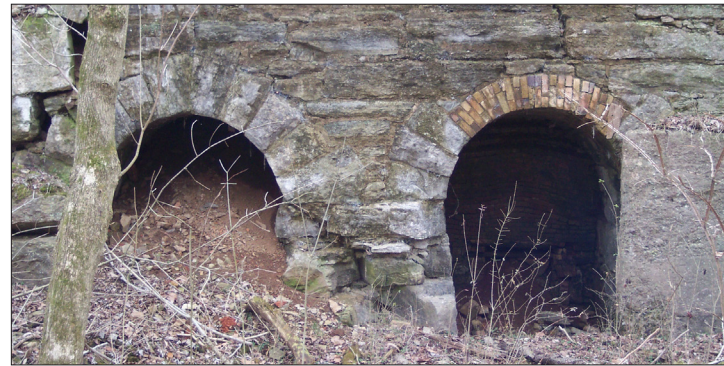
Arched openings at Kiln 48002
