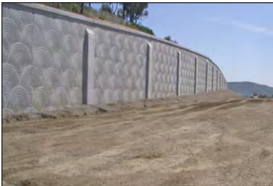
Formwork Used to Create Pattern Repetition in Retaining Wall
