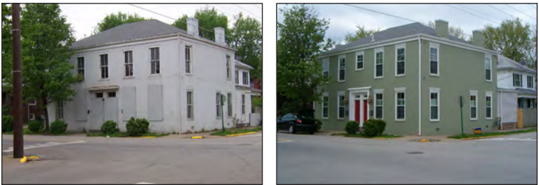
The Indiana House at Pearl and Maple Streets represents the proper rehabilitation of a historic structure. The original window (openings) were retained, and an appropriate color scheme was chosen to highlight the simple architectural details and brighten this formerly run-down eyesore.
