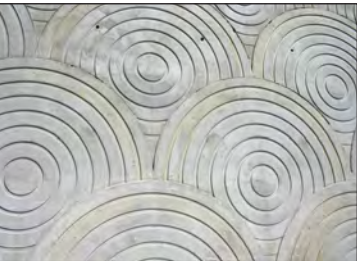
Formwork Used to Create Pattern Repetition in Retaining Wall
