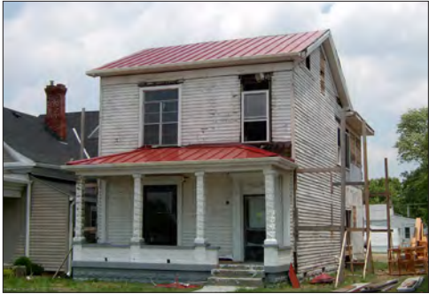
An example of a rehab project with inappropriate replacement windows. The expansion of the local historic district and subsequent rehabilitation guidelines would educate building owners on proper rehabilitation methods.
