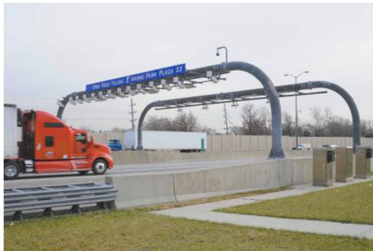
Traffic passes under gantry and does not stop
