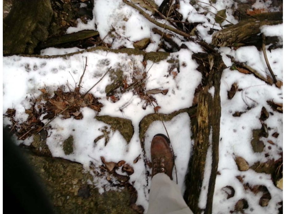
Photo 2: A-01, Joints in creek bed at 160-170 degrees with a secondary joint at 80 degrees
