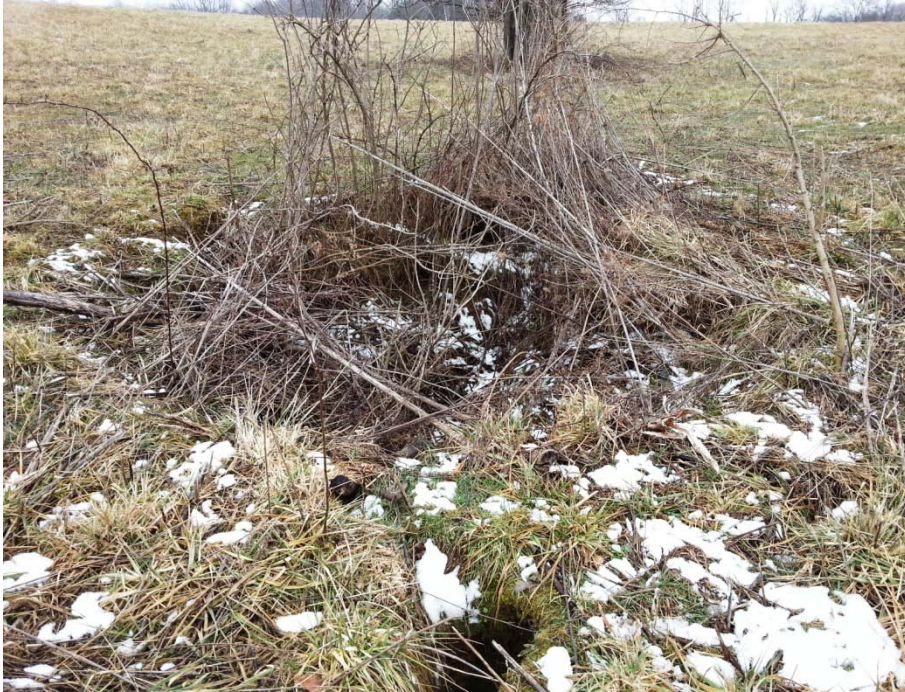
Photo 55: C-07, Distinct sinkhole approximately 10' x 15' x 4' deep.
