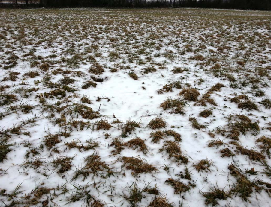
Photo 63: D-02 & D-03, Area surrounding 3" diameter open holes with no significant depression.
