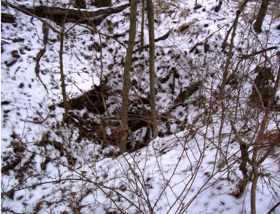
Photo 73: D-09, Set of 3 sinkholes approximately 10' diameter 7' deep with large swallow holes.
