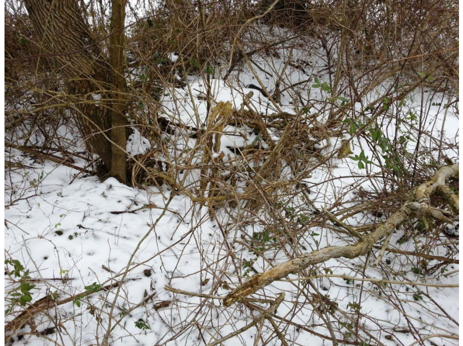
Photo 136: E-25, Two small sinkholes, both at base of trees, no visible swallow holes.
