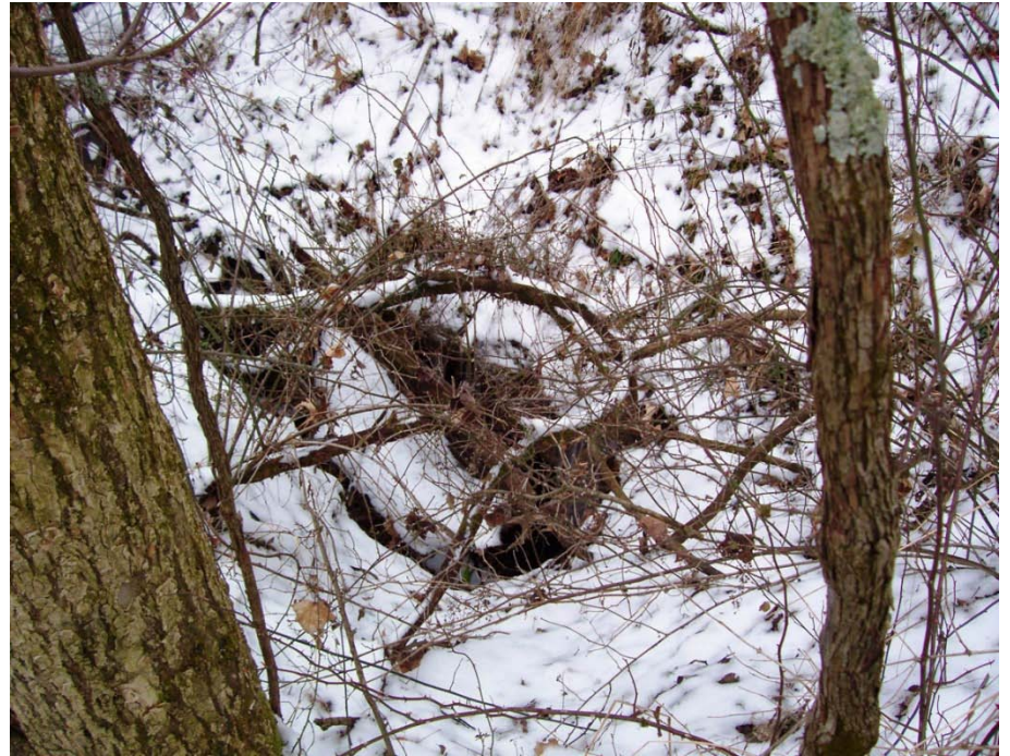
Photo 86: E-04, 15' x 25' sinkhole, approximately 5' deep. Corrugated (tin) roofing panels embedded in bottom.
