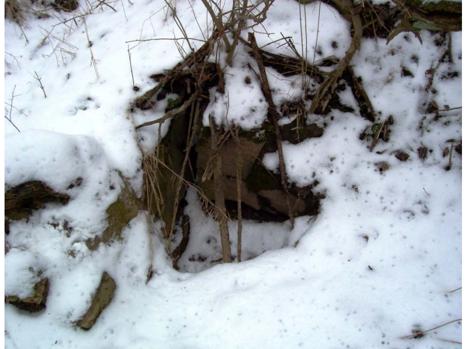
Photo 96: E-07, Swallow hole in a single sinkhole approximately 25' diameter approximately 5' deep.
