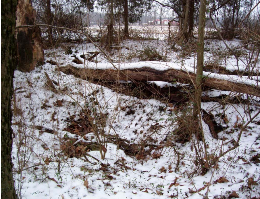
Photo 83: E-03, Single sinkhole approximately 25' diameter, with small swallow hole.
