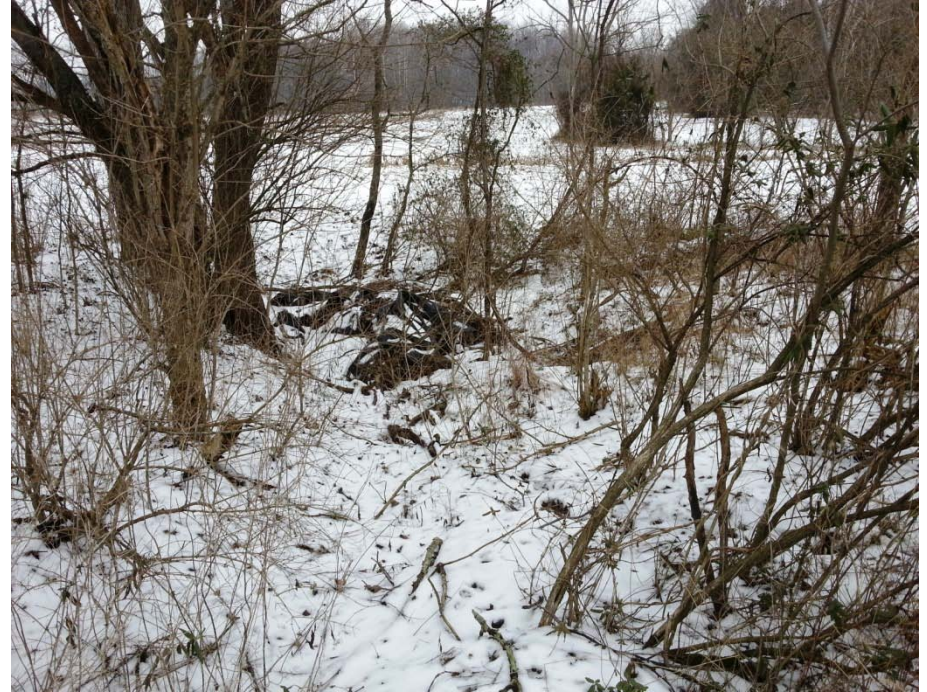
Photo 140: E-26, Large sink approximately 30' diameter, 6' deep, has PVC pipe draining into sinkhole and a pile of debris.
