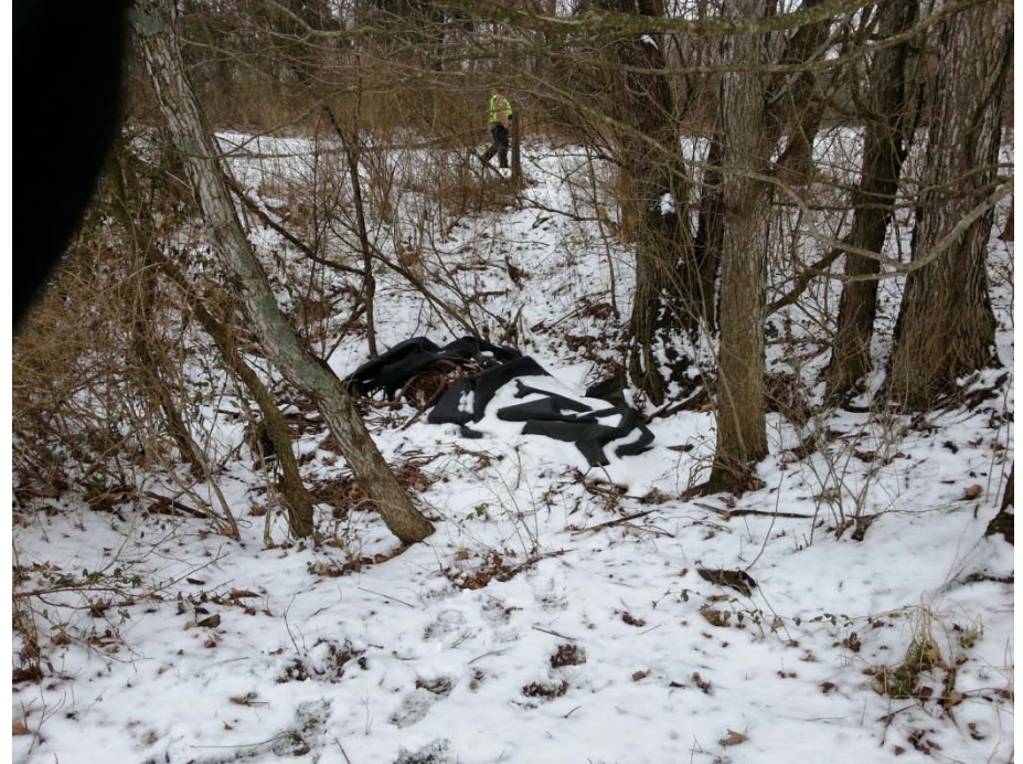
Photo 138: E-26, Large sink approximately 30' diameter, 6' deep, has PVC pipe draining into sinkhole and some debris piles.
