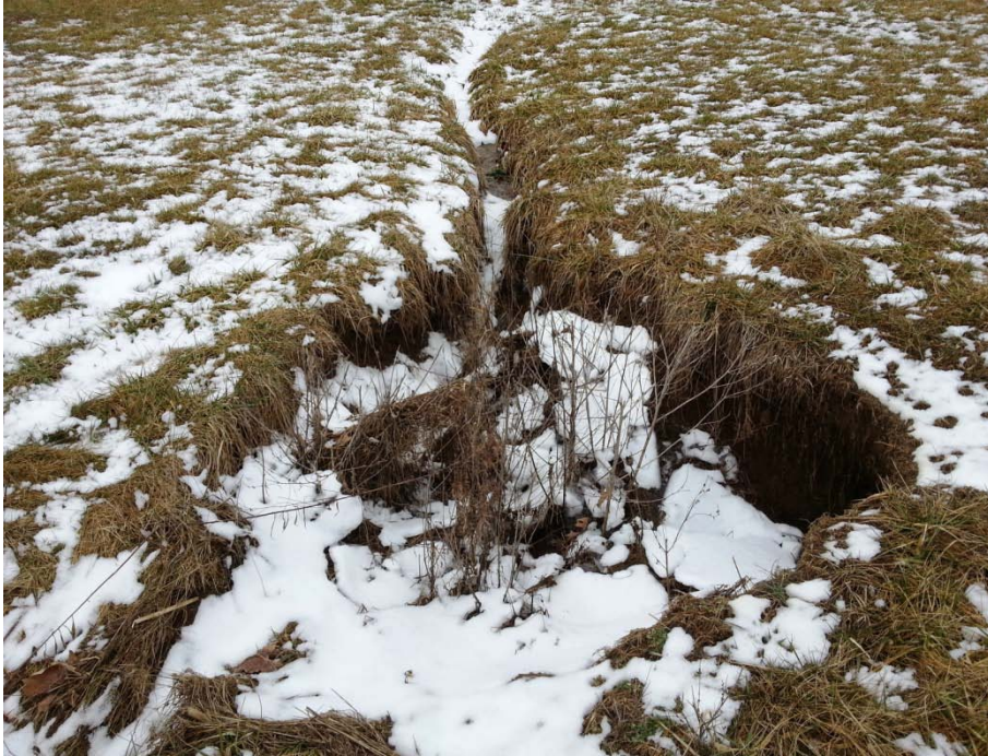
Photo 11: A-06, 2 small sinkholes, which swallow overflow from adjacent pond, both approximately 6' diameter, 3' deep.
