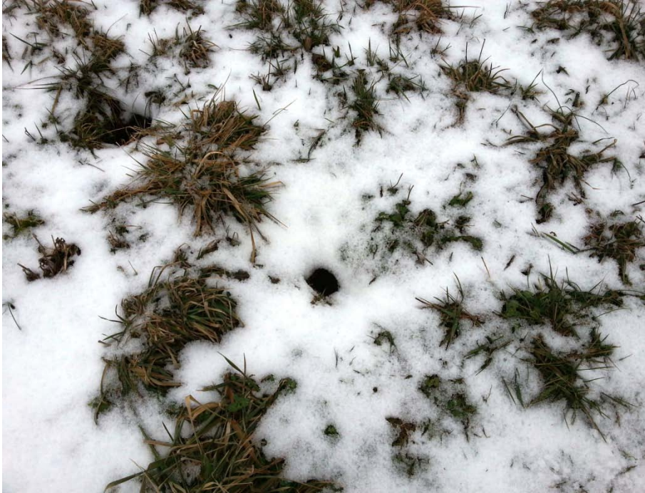
Photo 61: D-02 & D-03, 3" diameter open holes with no significant depression.
