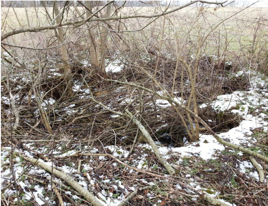
Photo 35: C-02, Small compact sinkhole, approximately 12' diameter, 4' deep, filled with piled sticks, has 8-10 potholes 2' diameter x 1' deep on north side of main sink.
