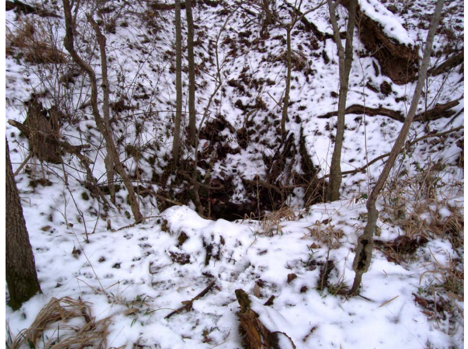
Photo 72: D-09, Set of 3 sinkholes approximately 10' diameter 7' deep with large swallow holes.
