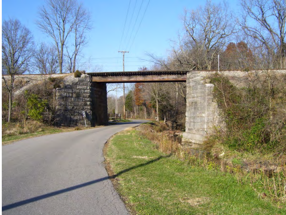
Plate 28. AL003 (079-087-20021), B & O Railroad Bridge, CR 75 East, looking northeast.
