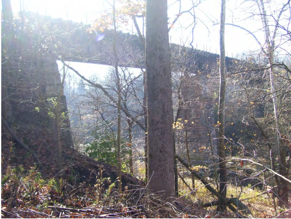
Plate 30. AL004, B & O Railroad Bridge, CR 175 North, looking south.
