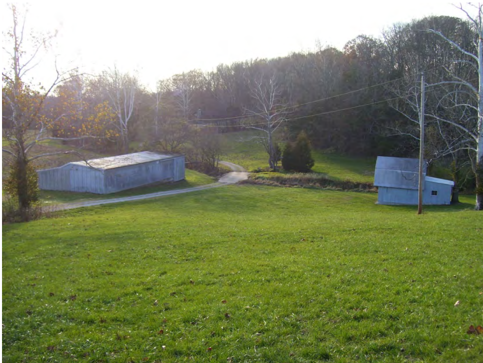
Plate 37. AL035 (079-087-20015), outbuildings at 75 East Private Road 235 North (Crech Farm), looking southwest.
