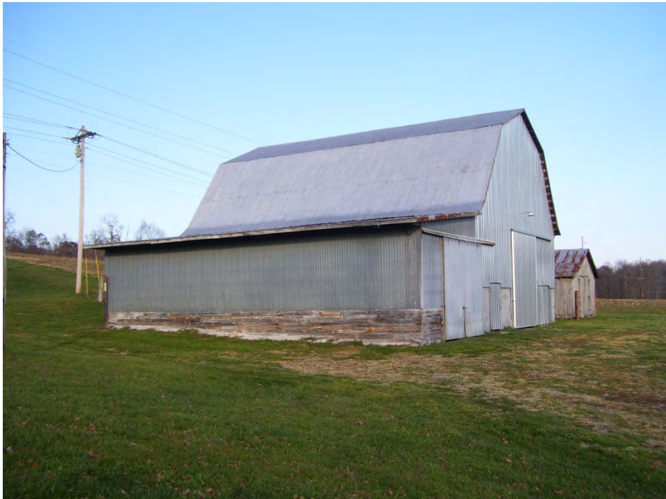
Plate 35. AL035 (079-087-20015), gambrel-roofed barn at 75 East Private Road 235 North (Creech Farm), looking northeast.
