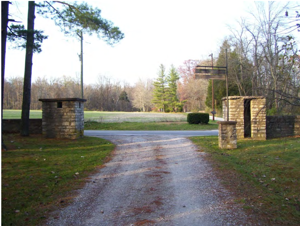
Plate 23. AL001 (079-087-20005), stone shelters at CR 350 North (Frank Selmier House), looking north.
