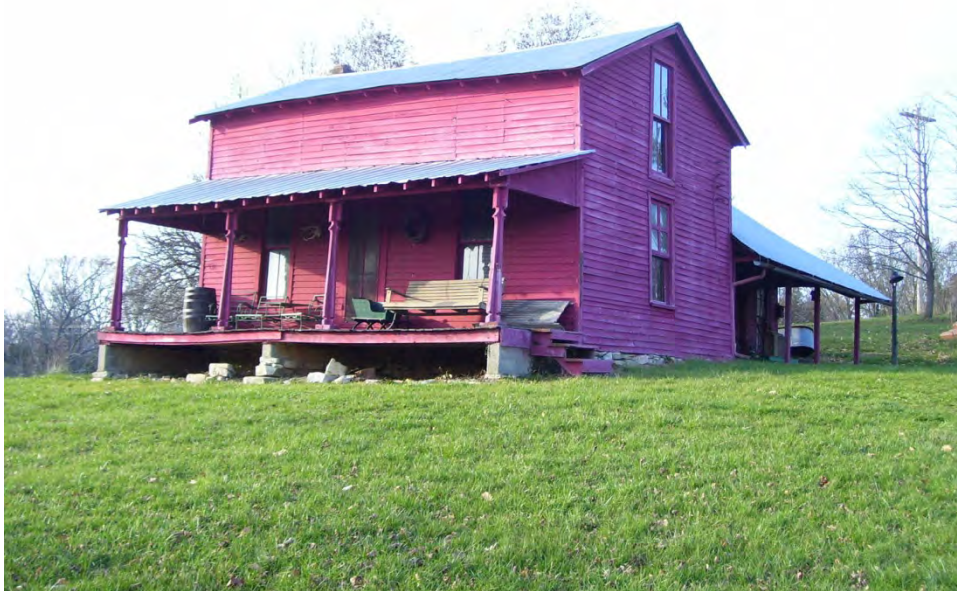
Plate 32. AL035 (079-087-20015), house at 75 East Private Road 235 North (Creech Farm), looking northwest.
