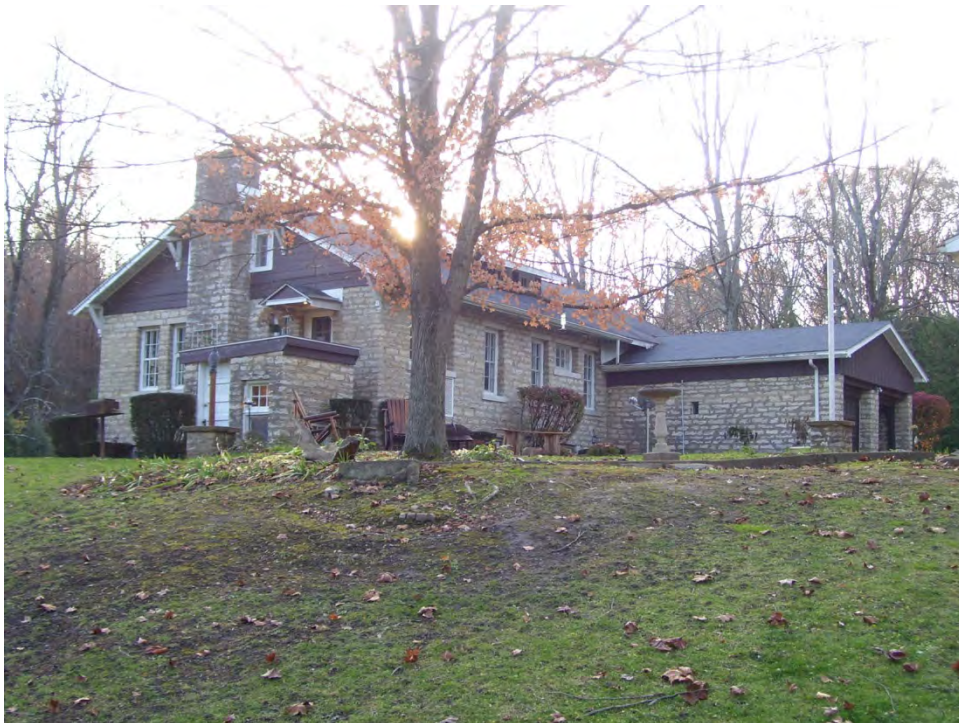
Plate 17. AL001 (079-087-20005), house at CR 350 North (Frank Selmier House), looking southwest.
