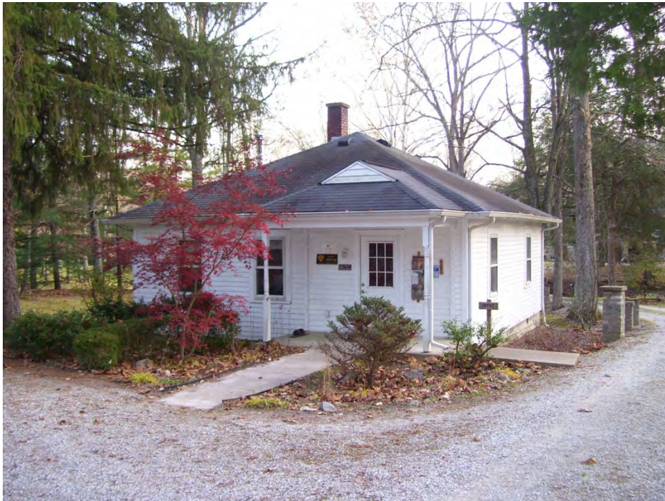
Plate 21. AL001 (079-087-20005), forester's office at CR 350 North (Frank Selmier House), looking southeast.
