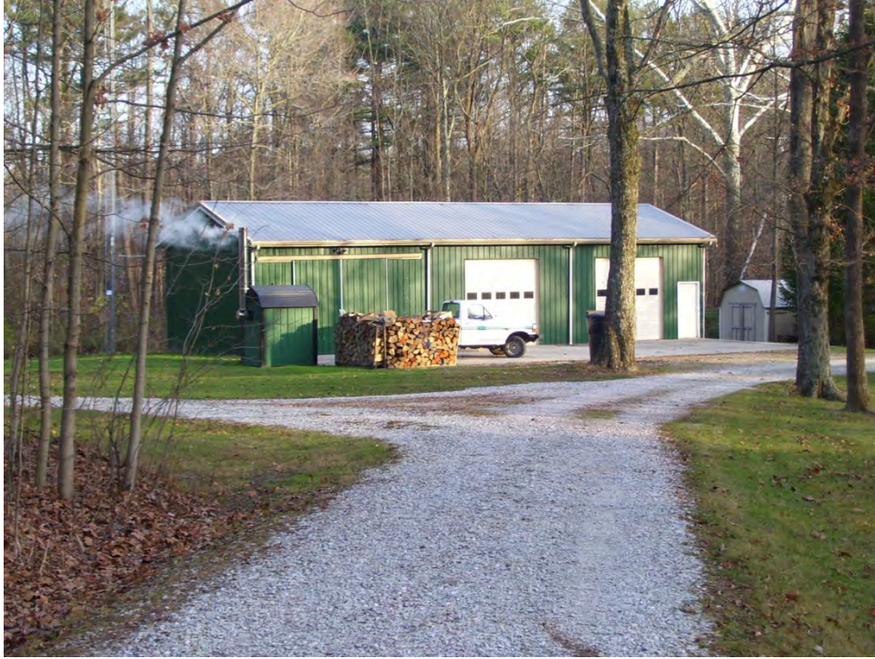
Plate 20. AL001 (079-087-20005), pole barn at CR 350 North (Frank Selmier House), looking southeast.
