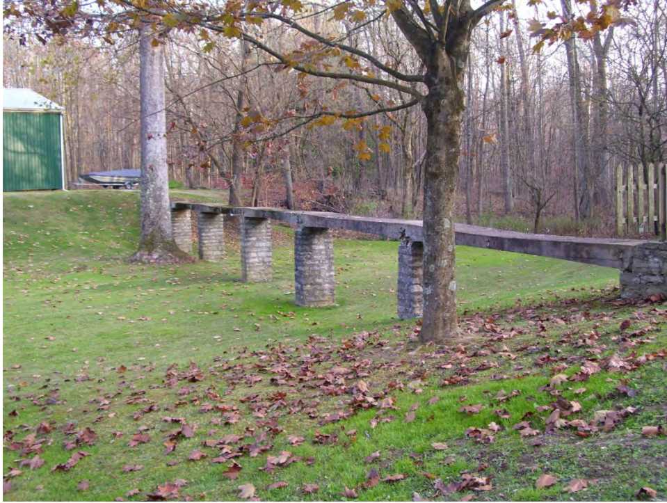
Plate 22. AL001 (079-087-20005), stone bridge at CR 350 North (Frank Selmier House), looking southeast.
