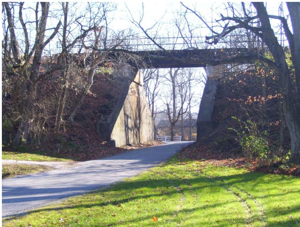
Plate 29. AL004, B & O Railroad Bridge, CR 175 North, looking southeast.
