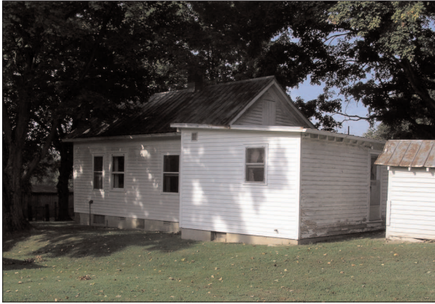
Pumphouse (right) and Kitchen Addition
