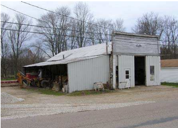
(50016) – Commercial Building Façade and East Elevation
