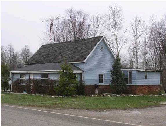
(36013) – Typical Alterations on a Clear Creek House
