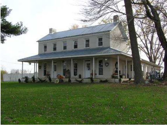
(45047) – Lawson Oliphant House Façade and West Elevation
