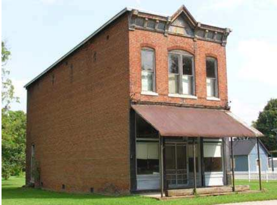
(56001) - Blackmore Store Façade and North Elevation
