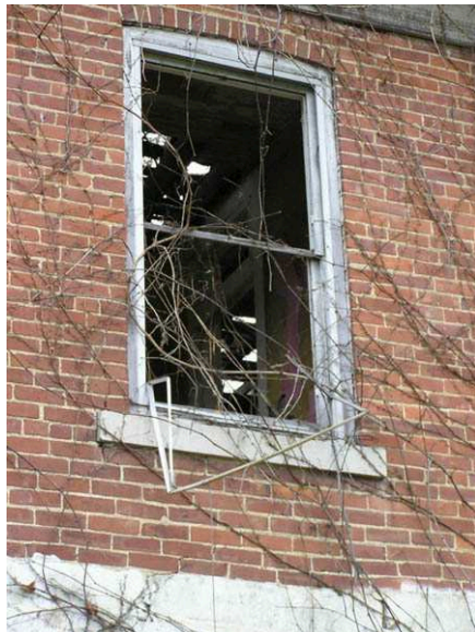
(40051) - Second Story Facade Window
