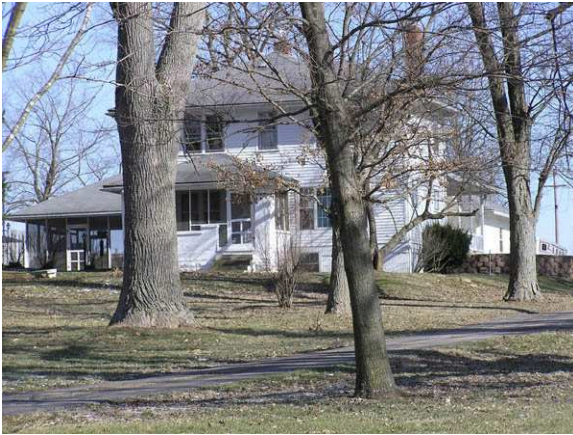
(35046) – House Façade and South Elevation
