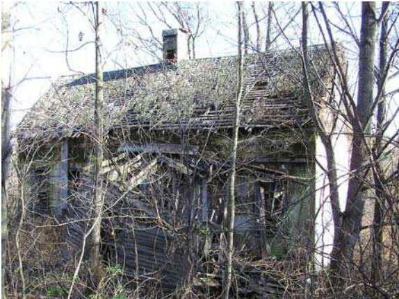
(55049) – Alexander Gilmore House Façade
