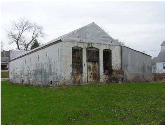
(50016) – Commercial Building West and South Elevations
