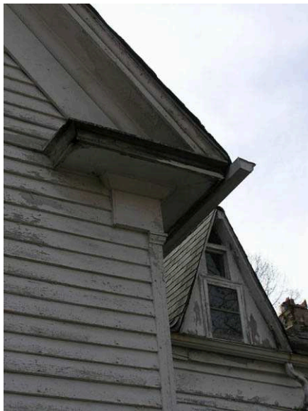
(45062) - Cornice Return and North Elevation Dormer
