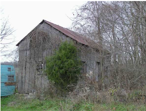
(40051) - Summer Kitchen South and East Elevations
