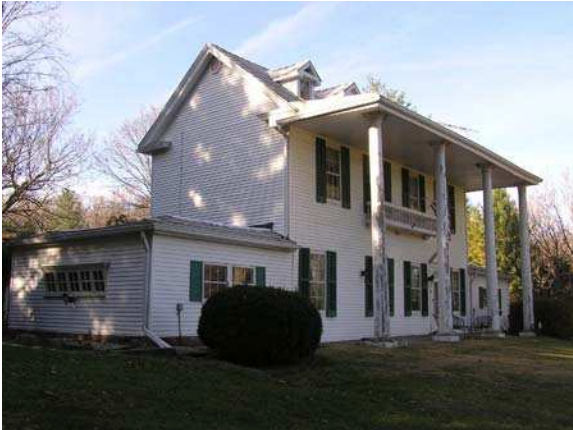
(50027) - Valhalla Façade and South Elevation
