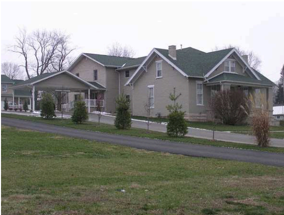
(36056) - House Façade and North Elevation with Associated Contemporary Residence to Rear
