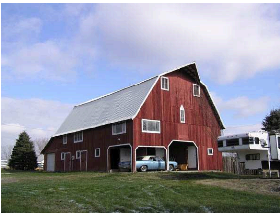
(35055) – Transverse Frame Barn Façade and West Elevation
