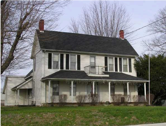
(35045) - House Façade and West Elevation
