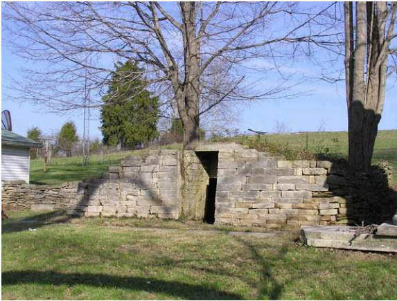
(45001) – Cold Cellar Façade
