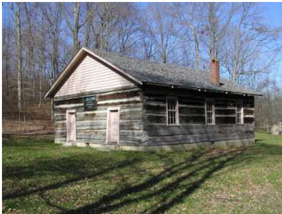
(50008) – Clifty Church Façade and East Elevation
