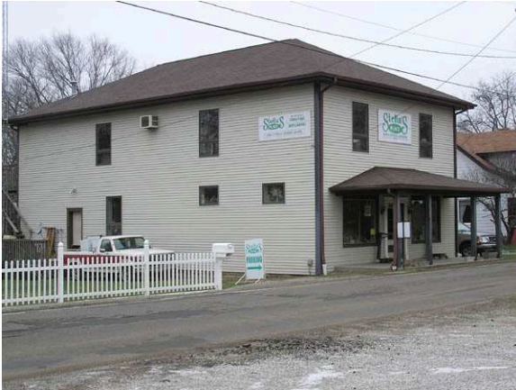
(36025) – Façade and South Elevation
