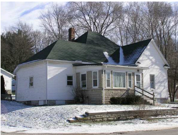
(36053) – Typical Alterations on a Clear Creek House
