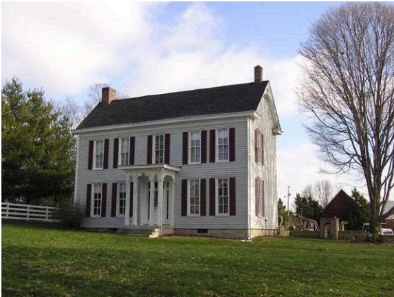
(35055) – House Façade and South Elevation
