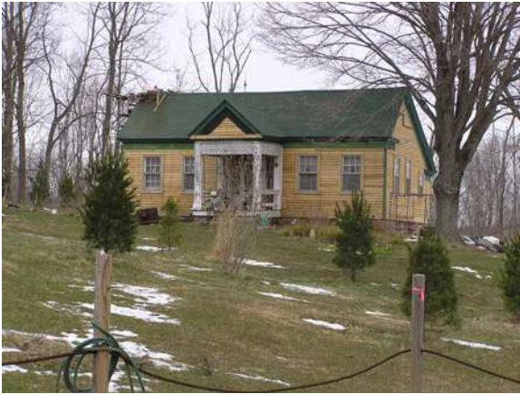
(45062) – Façade and North Elevation
