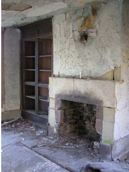
(55049) – Interior of Alexander Gilmore House
