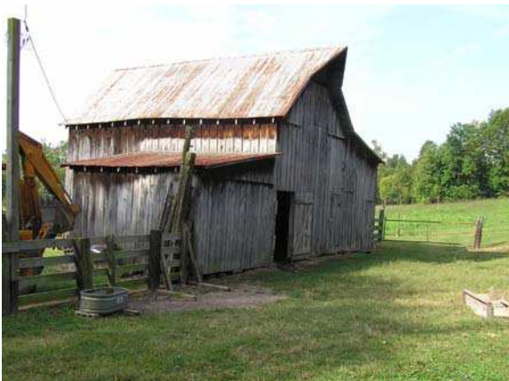
(55042) - Barn Façade and East Elevation
