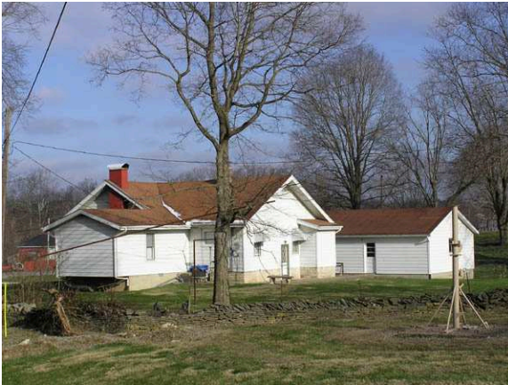
(35066) – House West and South Elevations with nearby Garage and Drystone Wall (35095)
