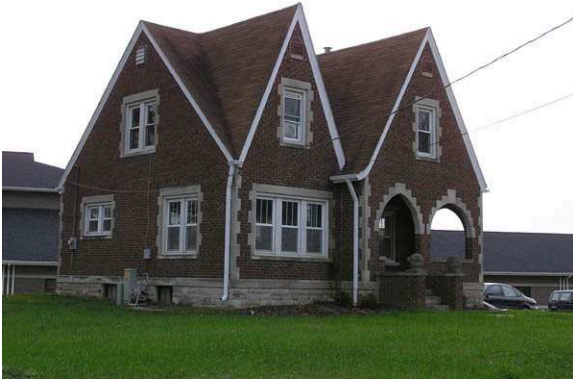
(35044) – Jameson House Façade and East Elevation
