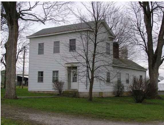
(35051) - House Façade and East Elevation
