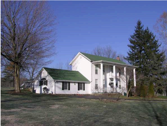
(35047) - House Façade and South Elevation
