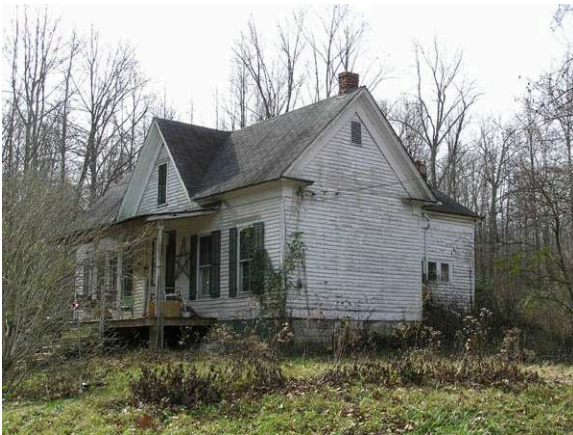
(45062) – House Facade and North Elevation
