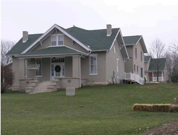
(36056) - House Façade and South Elevation with Associated Contemporary Residence to Rear
