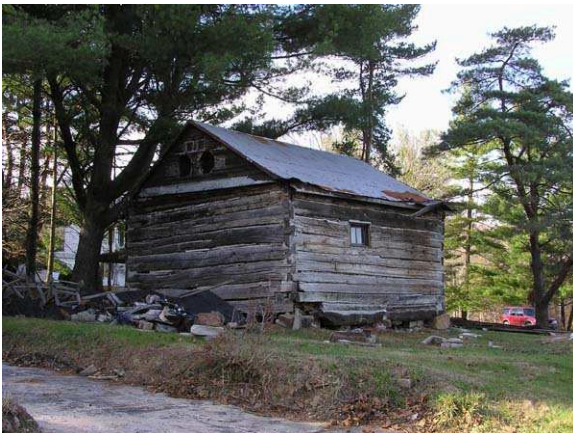
(50027) – Circa 1840 Log Structure
