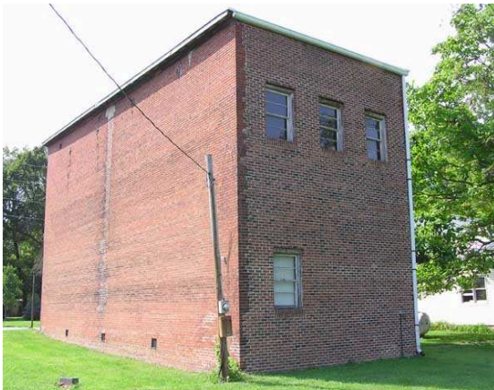
(56001) - Blackmore Store South and East Elevations
