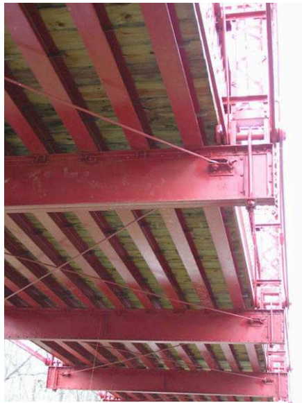
(35104) - Harris Ford Bridge Deck from Below
