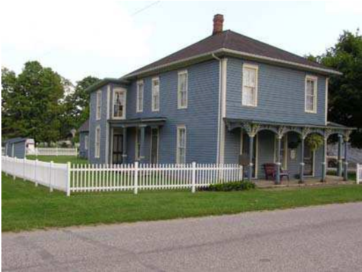
(56002) - Scotland Hotel Façade and North Elevation
