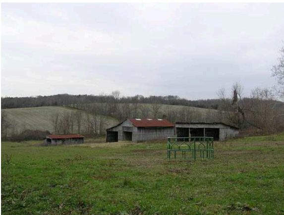
(40051) – Twentieth Century Outbuildings
