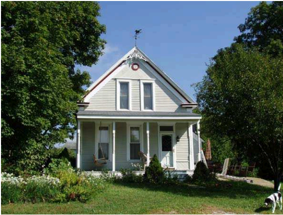
(45063) – Façade Looking North
