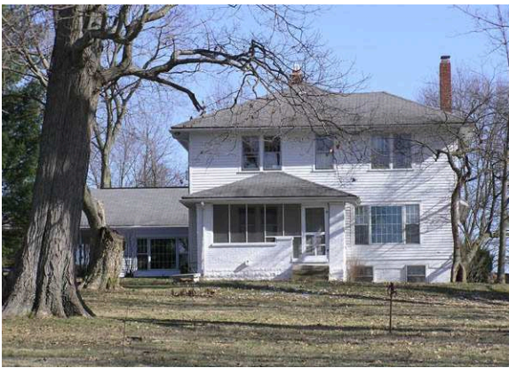
(35046) - House Façade with North Addition
