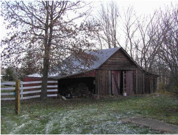
(35055) – Tool Shed Facade
