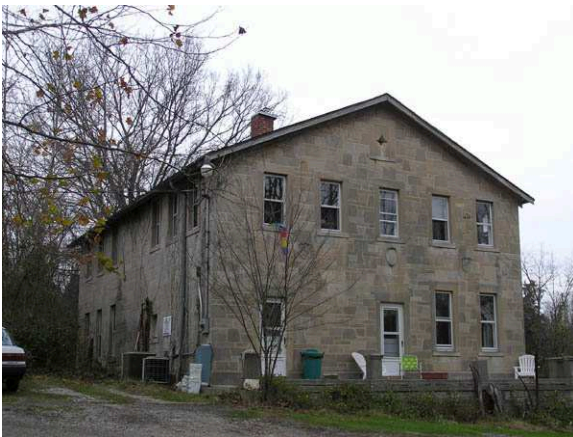
(35061) - Administration Building West Elevation and Facade
