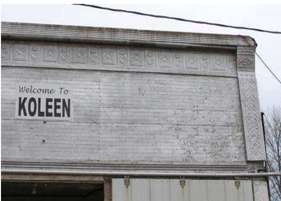
(50016) – Commercial Building Façade Detail
