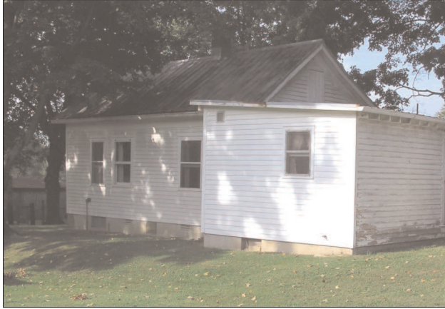
House Eastern and Northern Elevations
