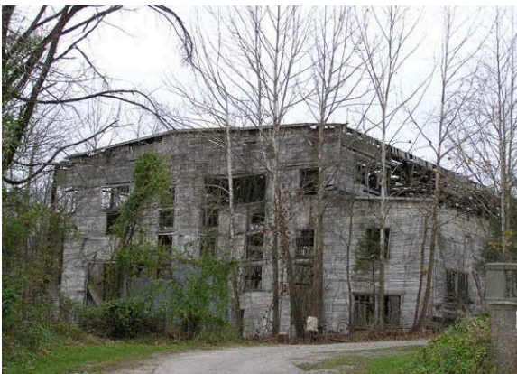
(35061) - Mill Building Facade
