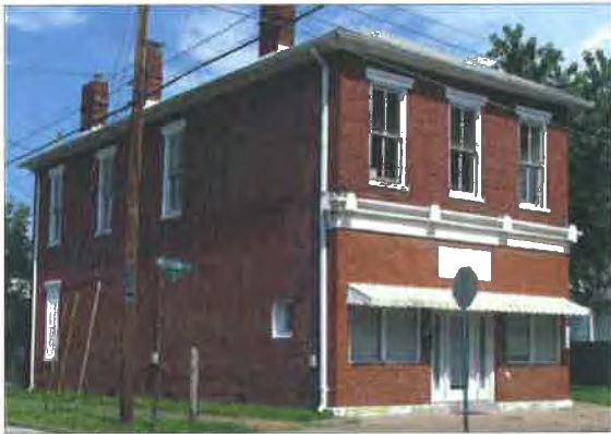
Commercial Building at 640 Mechanic Street
