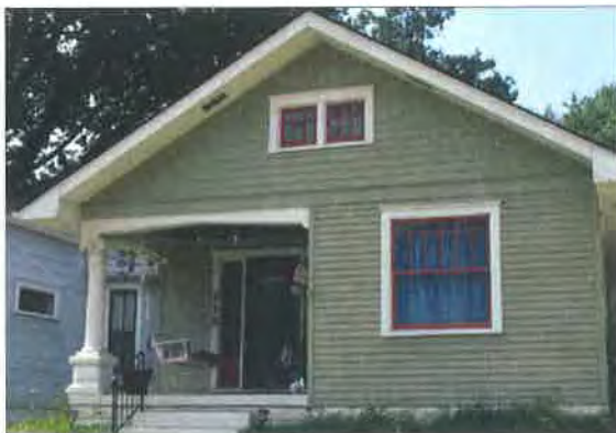
Residence at 713 E. Seventh Street
