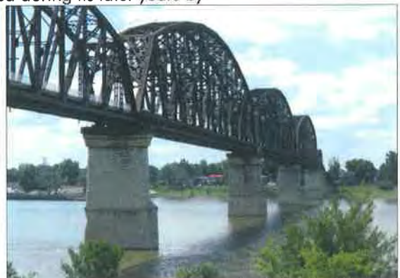
Conversion of the Big Four Bridge into a pedestrian/bicycle trail
