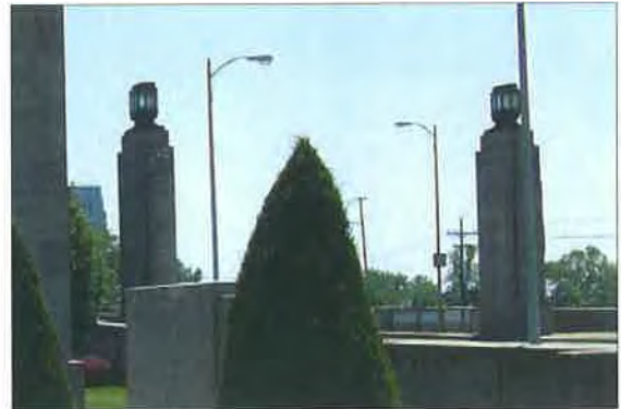
Art Deco Pylons at the George Rogers Clark Memorial Bridge
