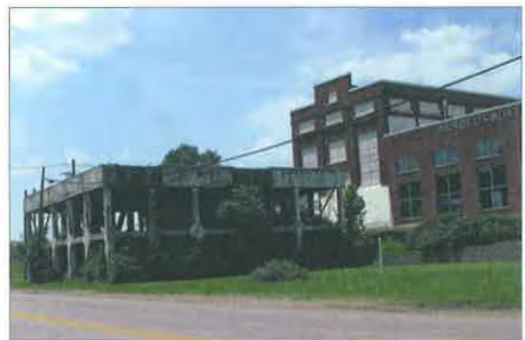
Industrial Complex at 2035–2039 River Road
