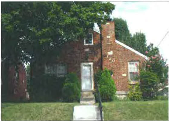
120 North Randolph Street
