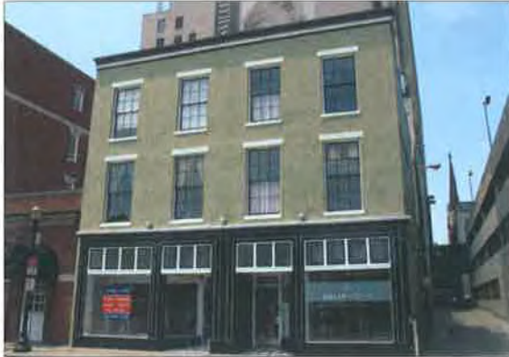
Commercial Building at 438 S. Third Street
