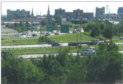
Kennedy Interchange in Downtown Louisville
