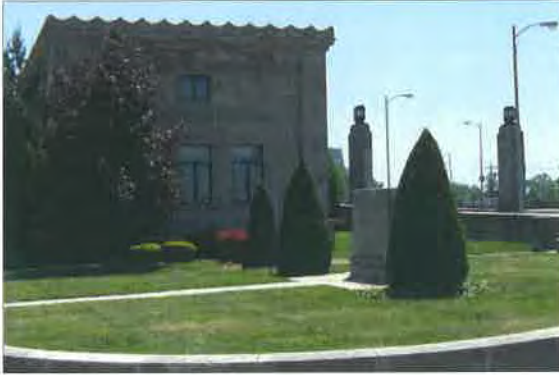
Municipal Bridge Administration Building and Pylons Beyond
