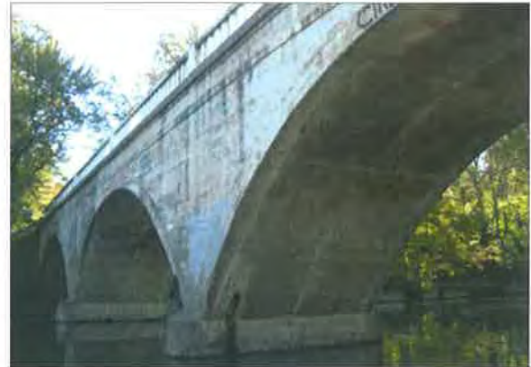
Upper River Road Bridge over Harrods Creek
