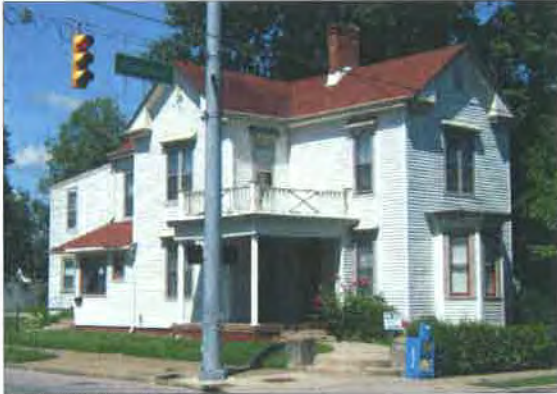
Gebhart-Hedden House at 801 Vincennes Street
