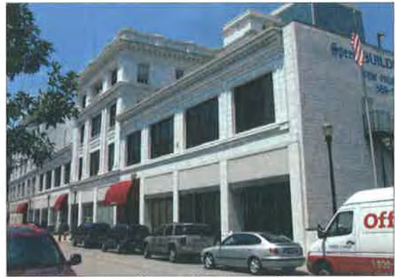
Speed Building Designed by Louisville Architect Arthur Loomis
