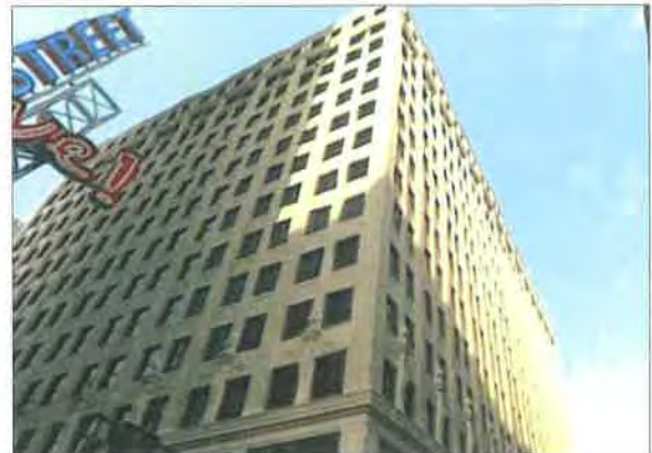
Starks Building at 455 S. Fourth
