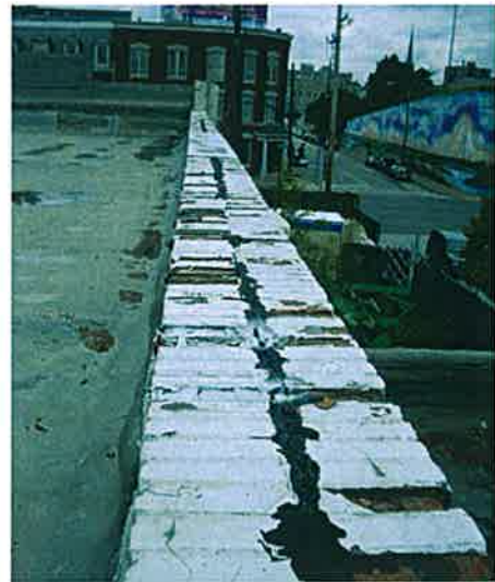
Typical Brick Wall Termination – No Coping
