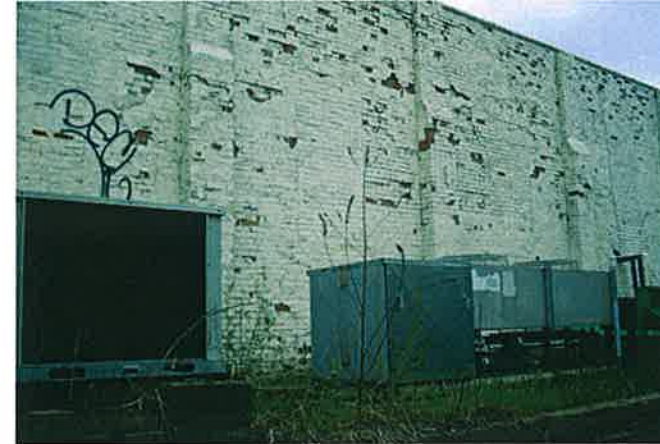
West Elevation Former Tank Room
