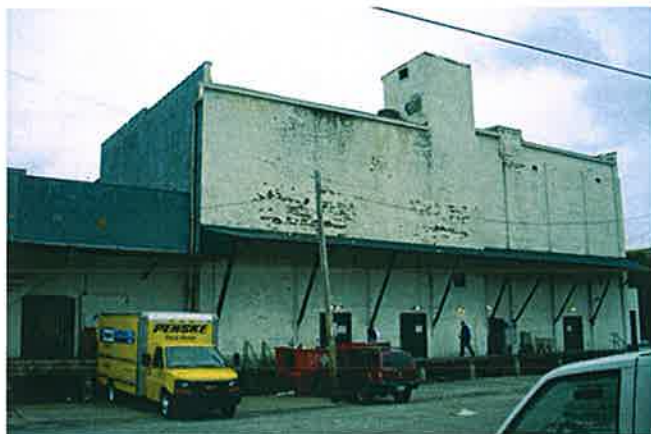
Loading Dock North Elevation at Coolers F and G
