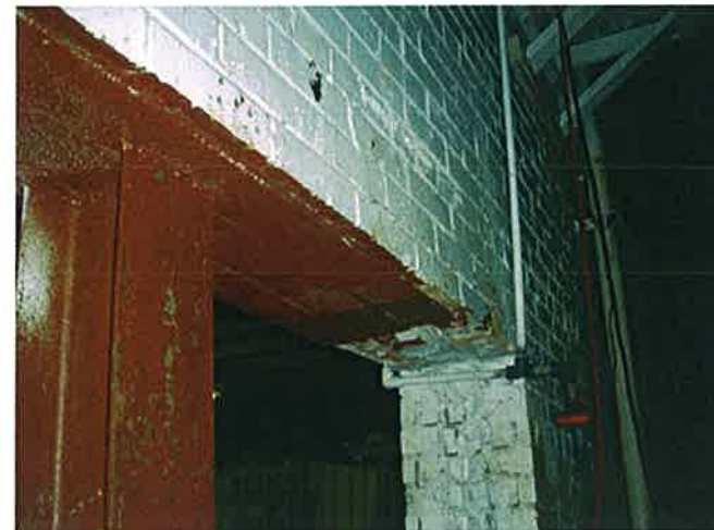
Expanded Masonry Opening -- Lintel Bearing Removed
