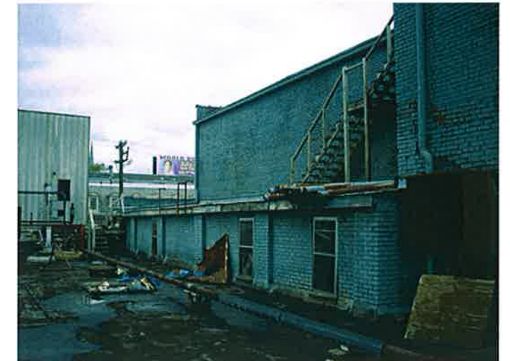
View on Ice Tank Roof looking towards Mechanical Room B.
