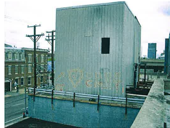
Metal Shed over Ice Shipping Room
