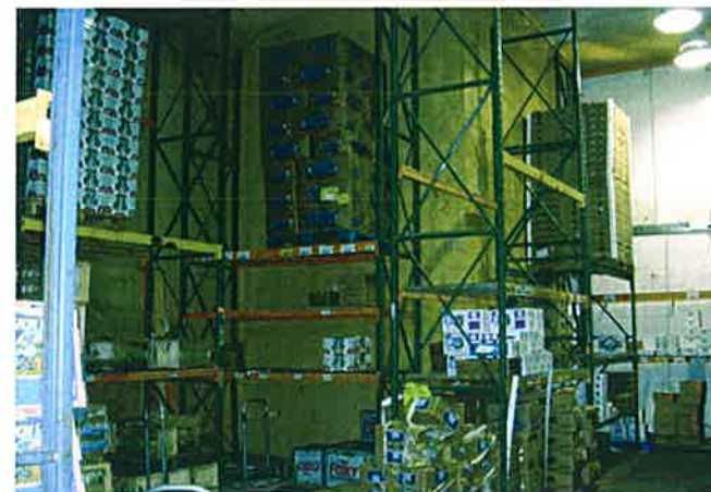
View of Main Cooler/Freezer with High Storage Racking
