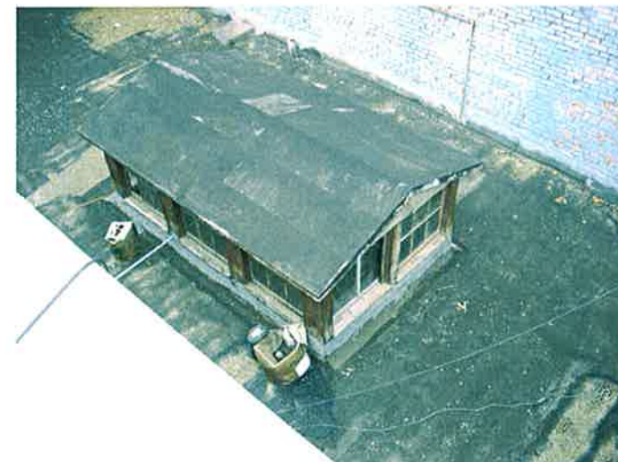
Monitor above Shop Space
