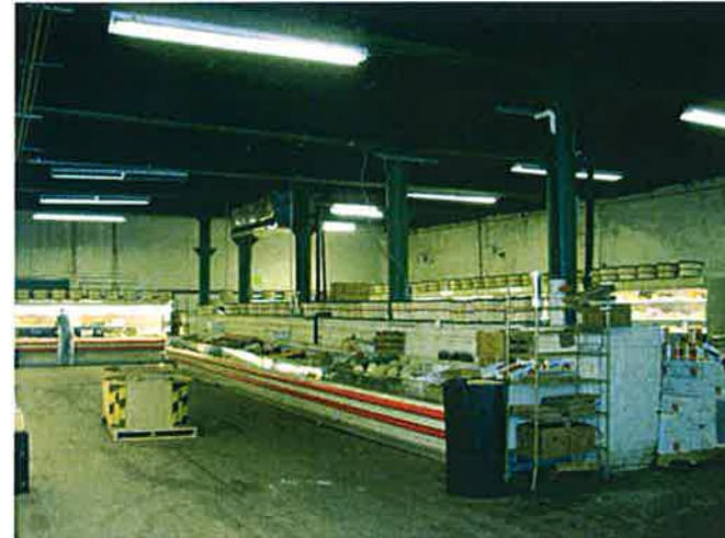
Former Tank Room looking Southwest
