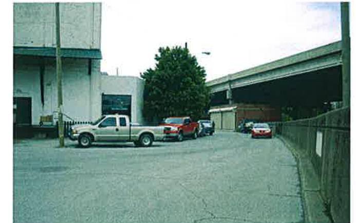
View North up Hancock Street -- Path of New Right-of-Way
