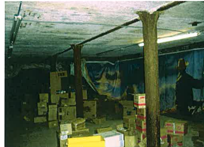
Cooler G Second Level looking Northeast
