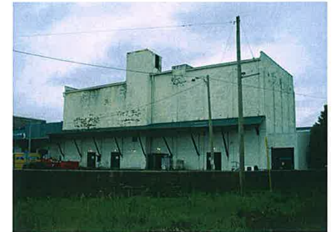
North Elevation showing Four Distinct Building Phases
