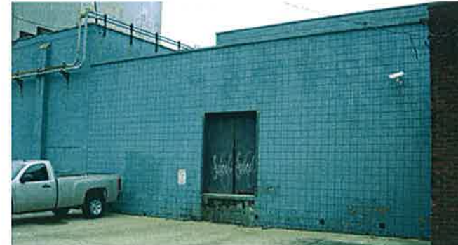
South East Dock (South Elevation), Ice Shipping Room to Left
