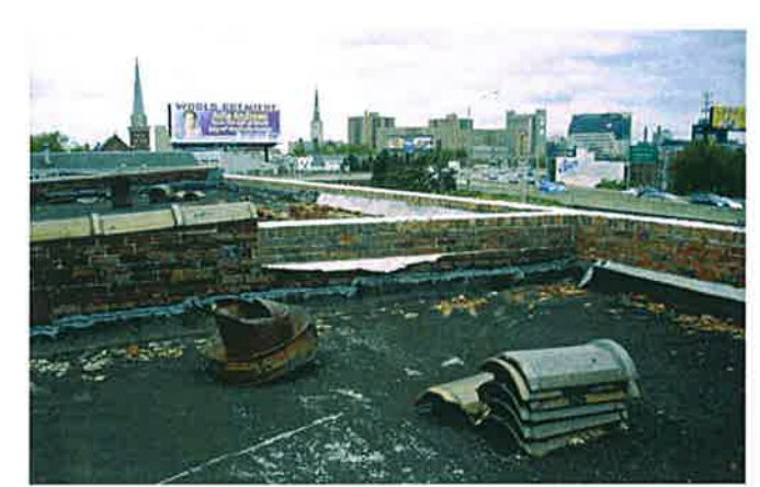
Roof at Cooler G
