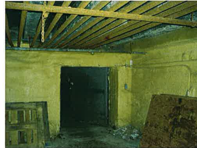
Ice Cooler C - Looking East
