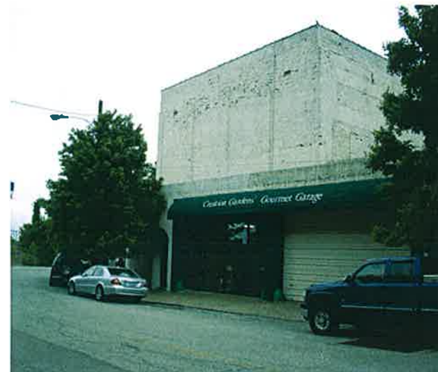
Former Garage Openings at West Elevation
