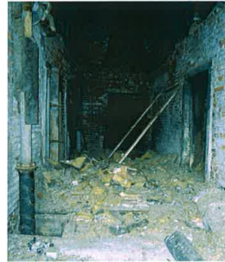
Corridor at Third Level between Cooler F and G
