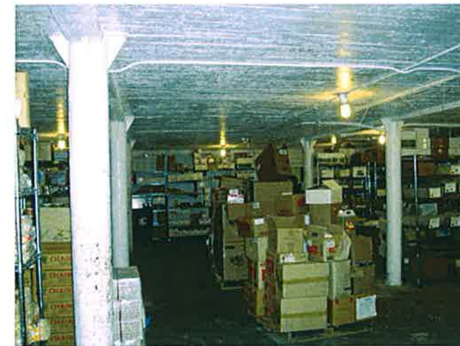
Cooler G Low Ceiling (8'-2"), Tight Column Grid (+/- 12'-0")
