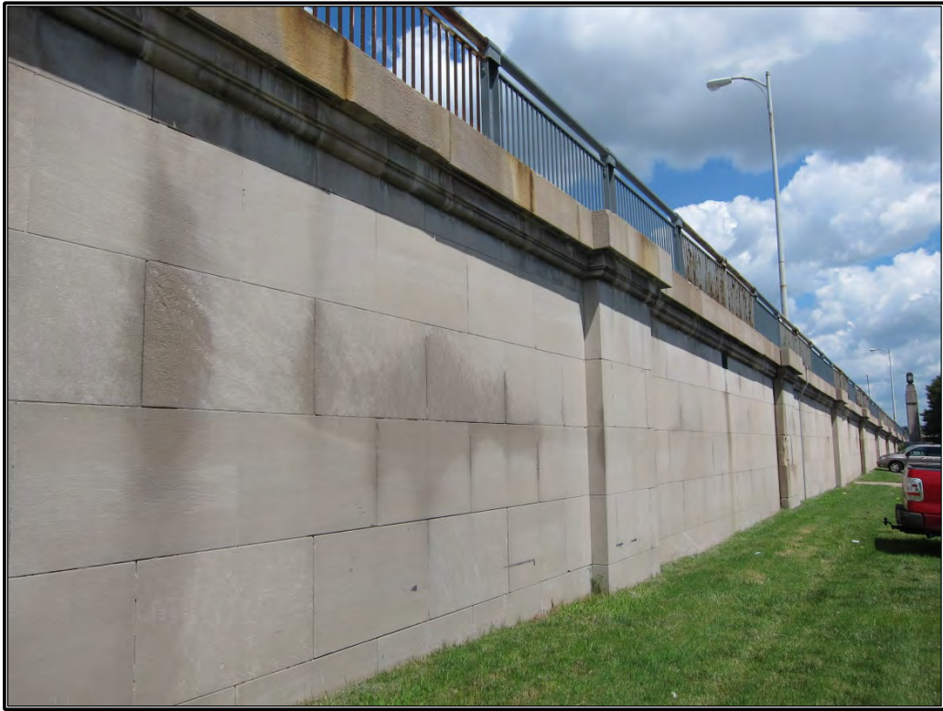
Figure 17. Overview of eastern mortared limestone block wall.
