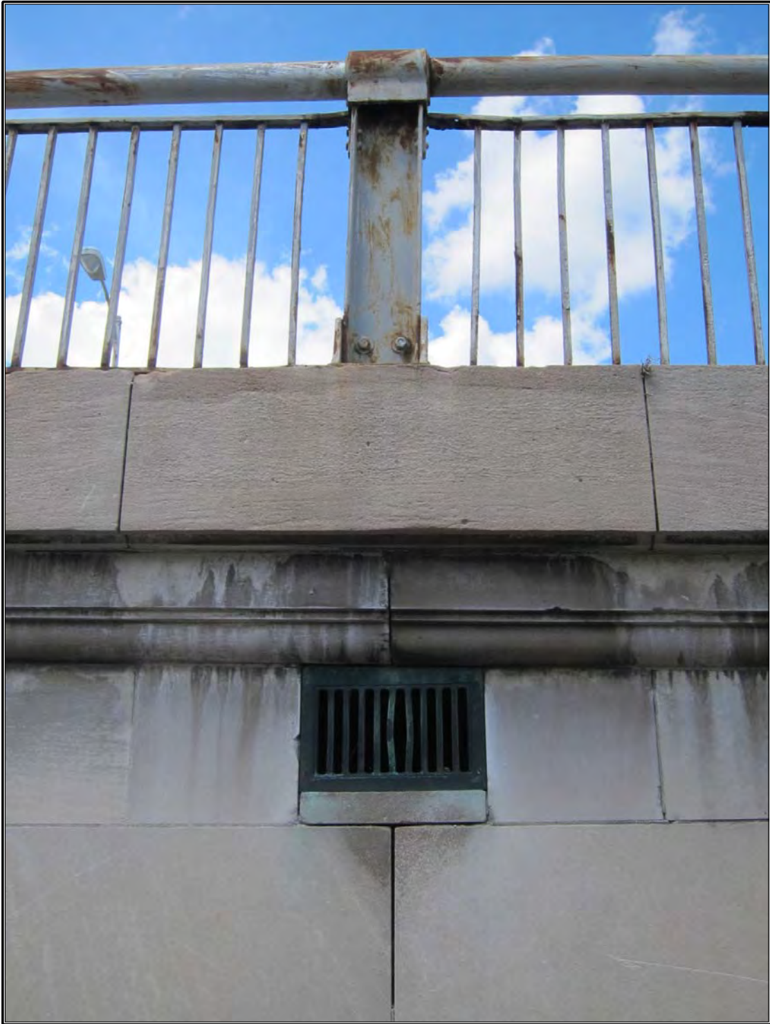
Figure 19. Detail of copper vent.
