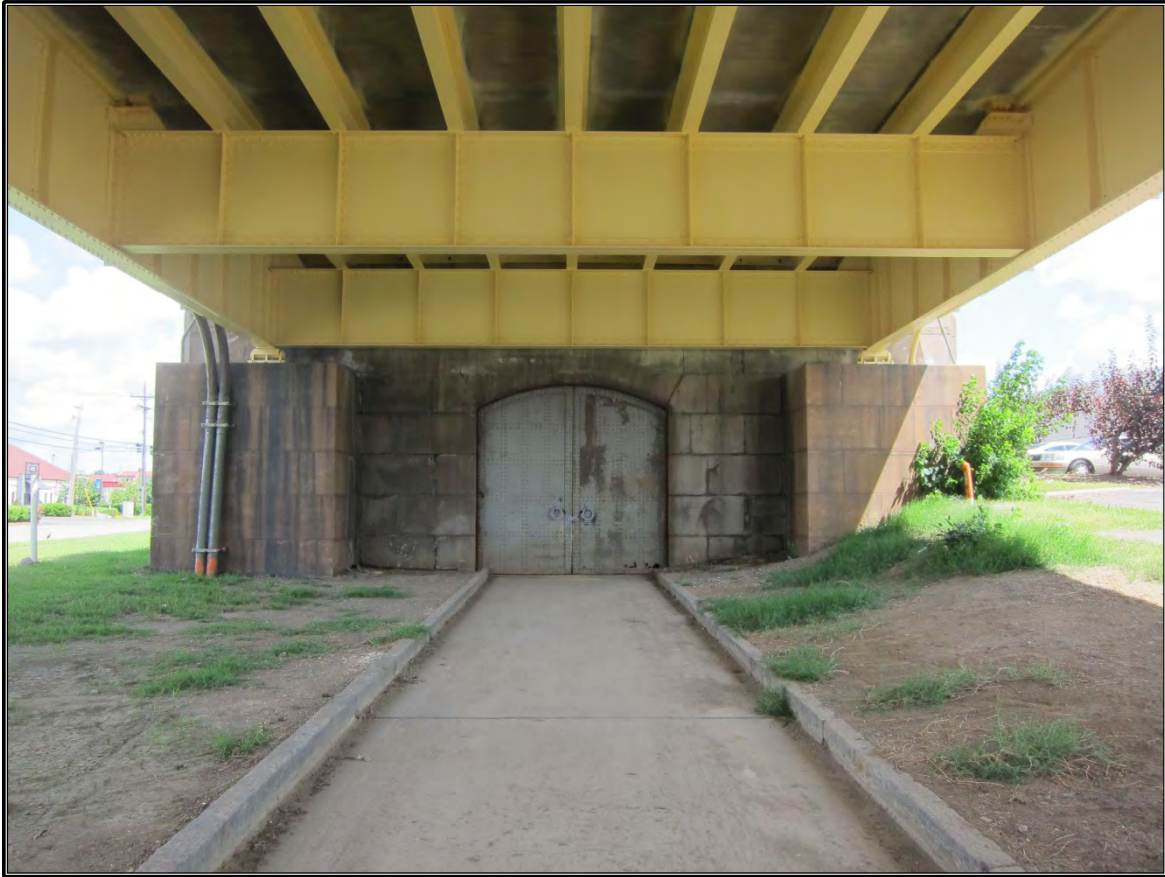
Figure 22. Riveted metal doors beneath southern end of approach.
