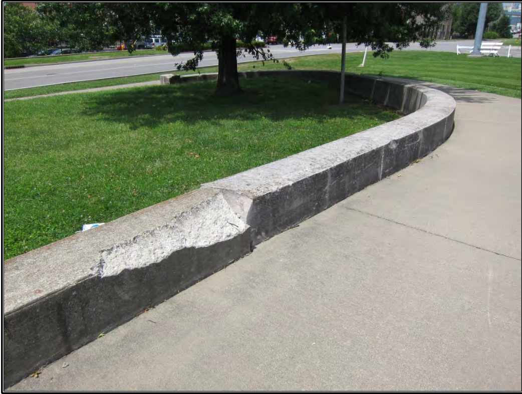
Figure 6. Damage to western edging wall north of pylons.
