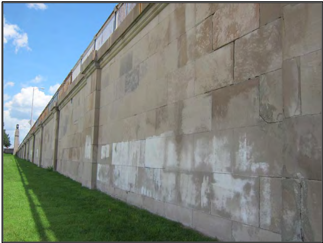
Figure 18. Overview of western mortared limestone block wall.
