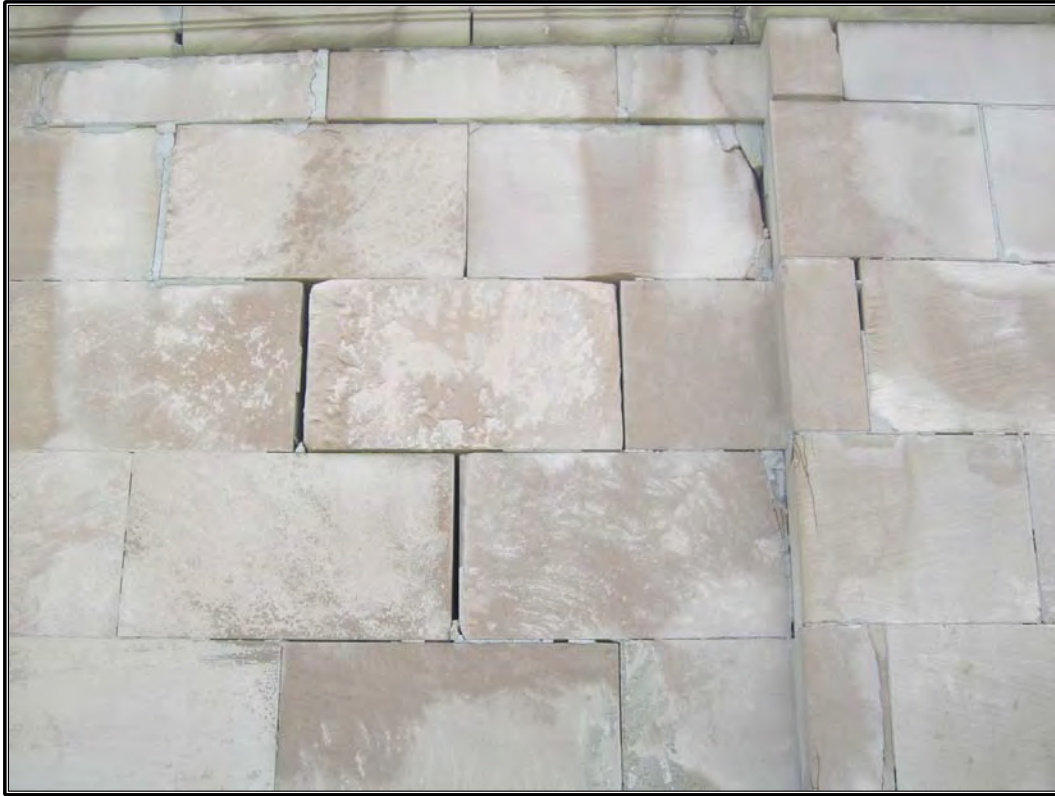
Figure 20. Damage to western limestone block wall.
