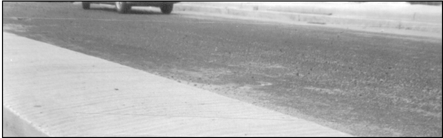
Figure 5-2. Concrete Center Curb
