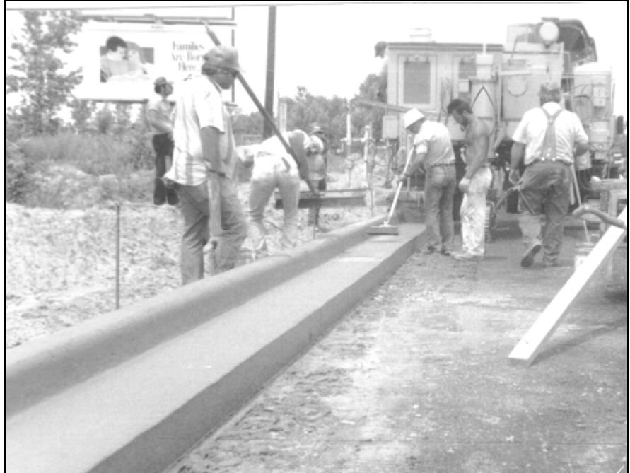
Figure 5-1. Combined Curb and Gutter
