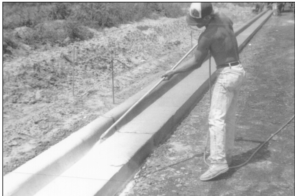
Figure 5-5. Applying Curing Compound
