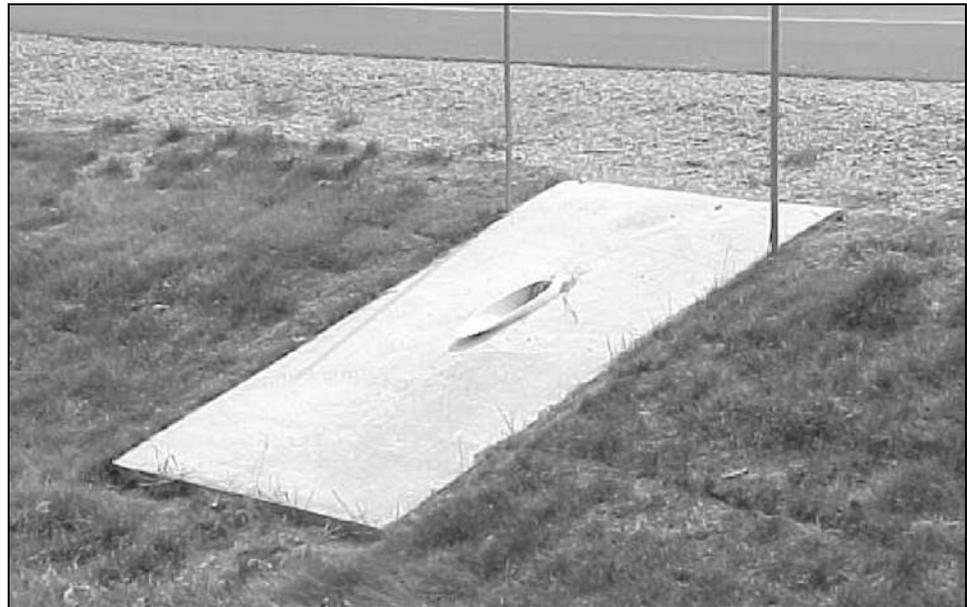
**Figure 10-8. Underdrain Outlet Protector**
