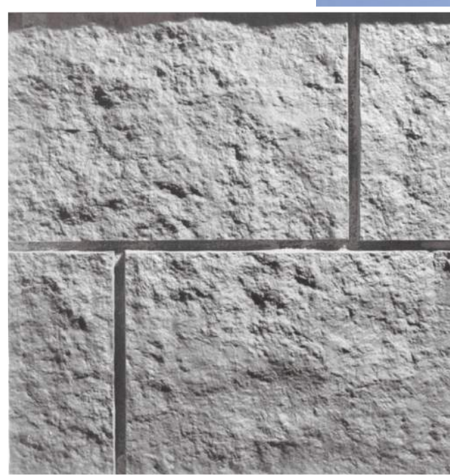
Chiseled Limestone w/ Joints
