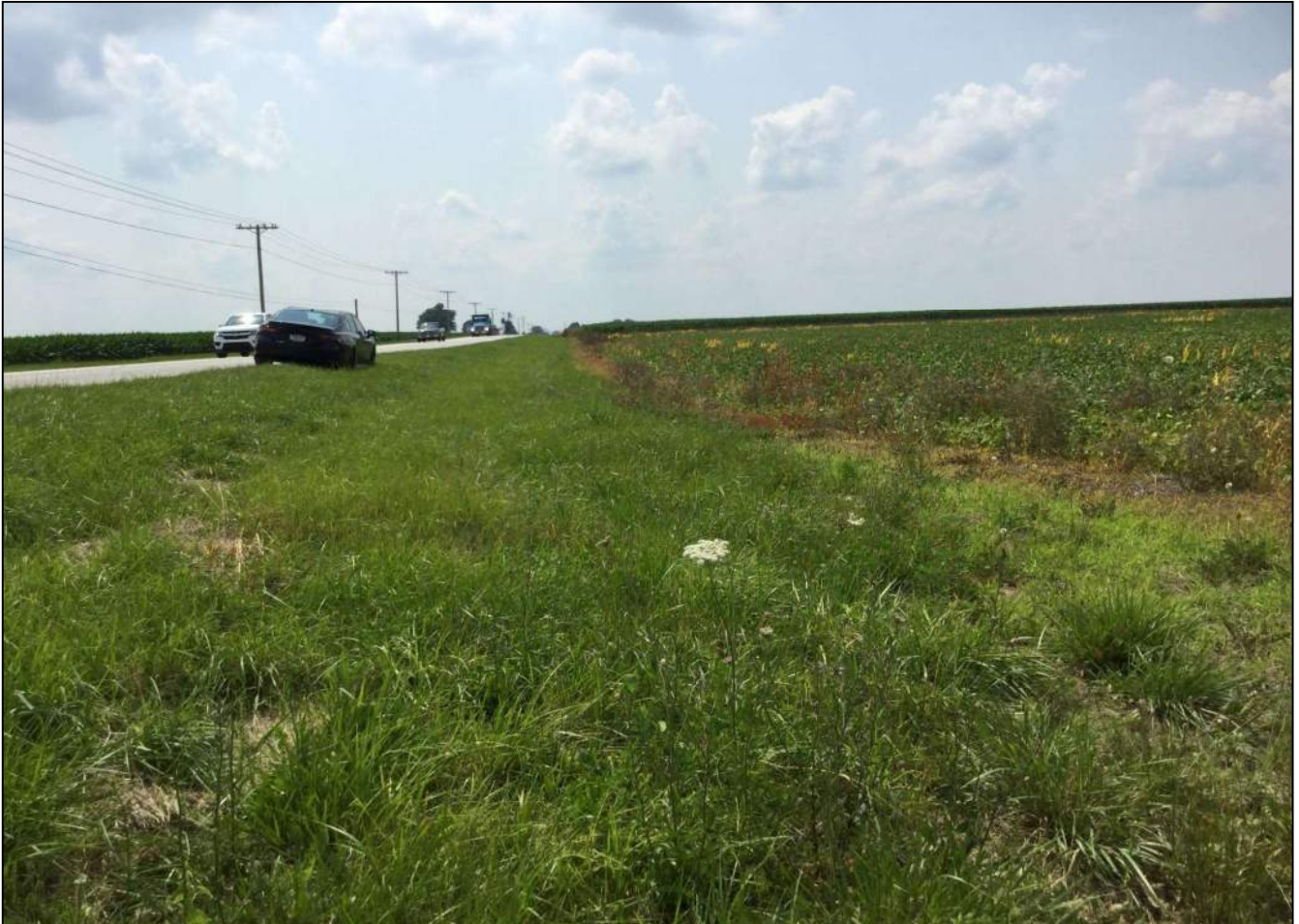
172. Looking west along the north side (WB lane) of SR 32 just west of Structure No. 111. Photo taken July 6, 2021.
