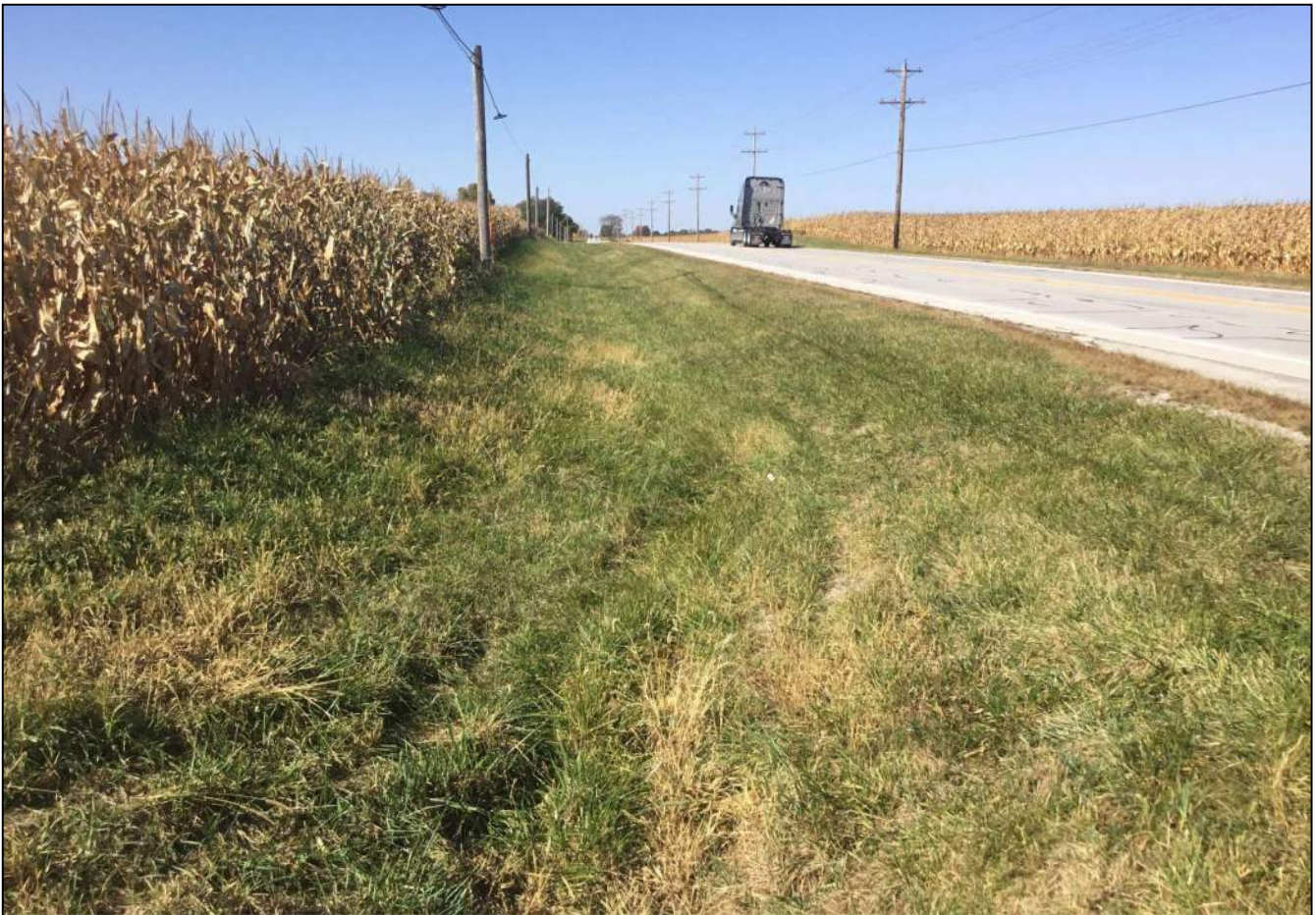
125. Looking west along the south side (EB lane) of SR 32 just west of CR 650 W. This photo also denotes the end of the second EB passing lane. Photo taken October 8, 2020.
