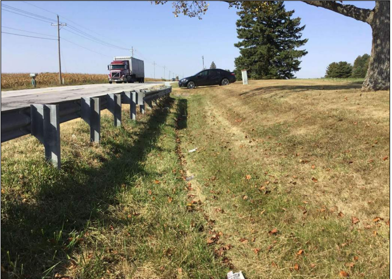
96. Looking west up the north side (WB lane) of SR 32 just west of Wolf Creek. Photo taken October 7, 2020.
