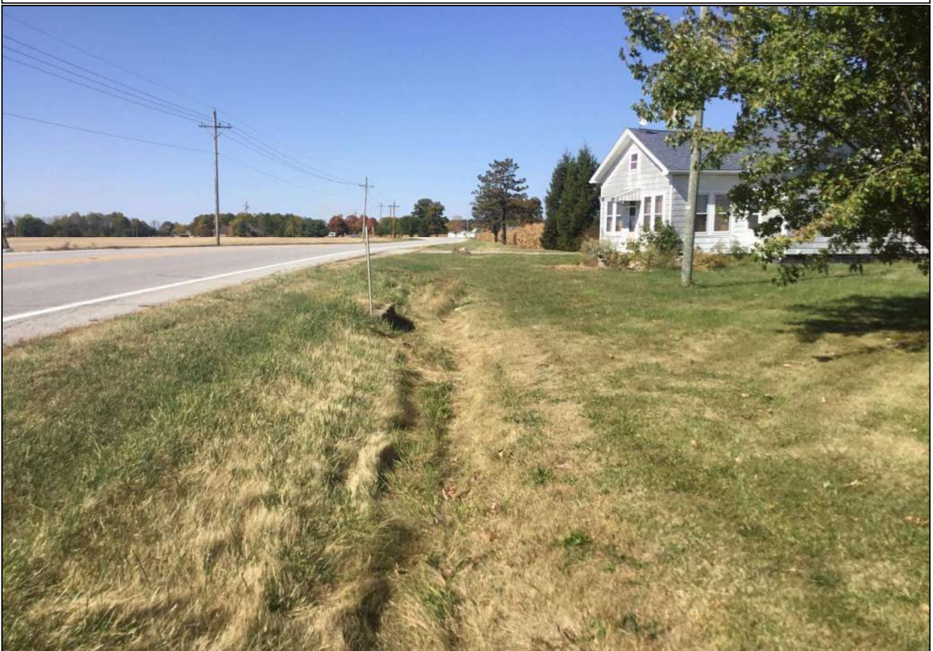
70. Looking west along the north side of SR 32 (WB lane) at the surrounding landscape. Please note the concrete headwall in the background. This structure will not be impacted as part of this project. Photo taken October 7, 2020.
