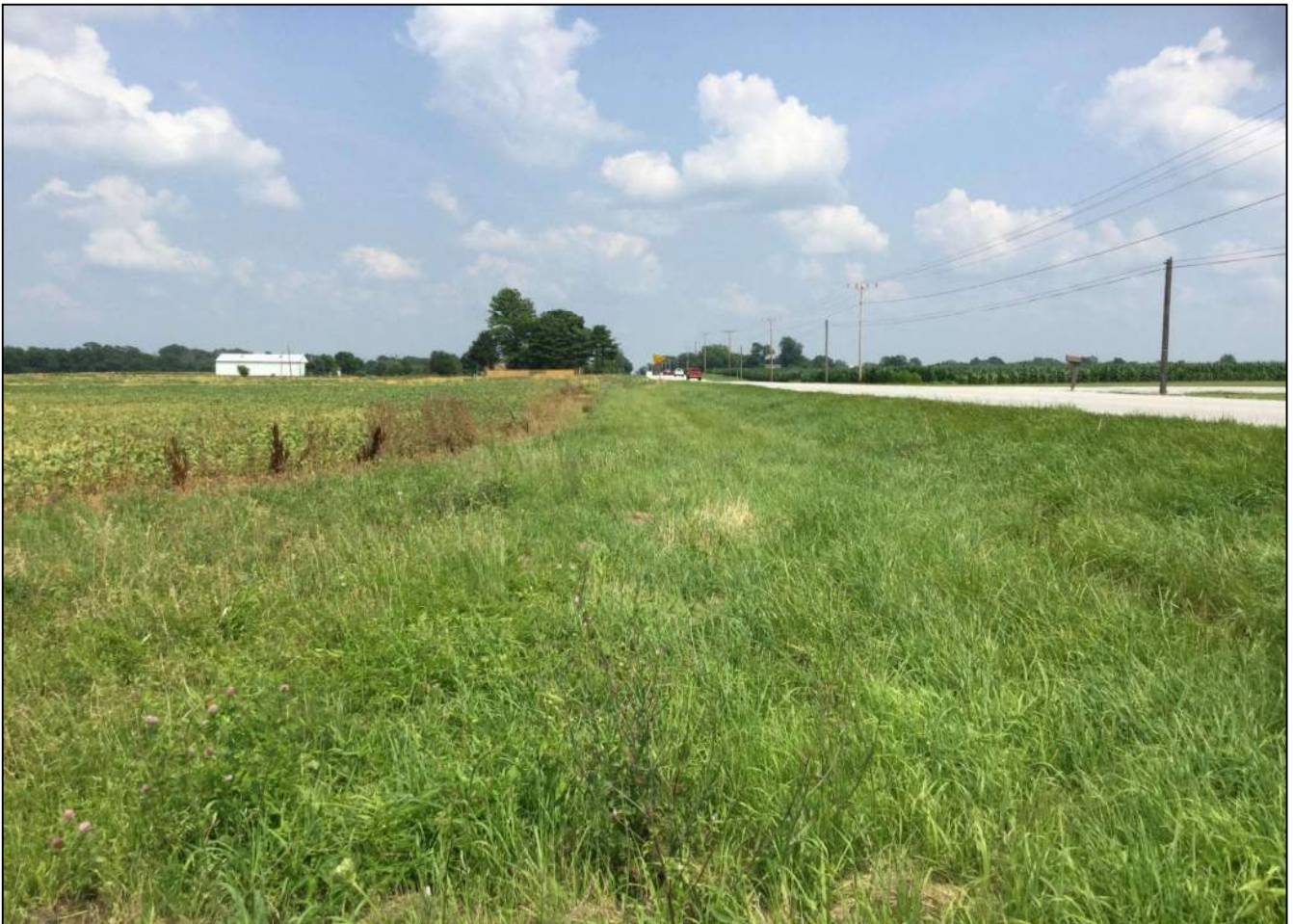
169. Looking east along the north side (WB lane) of SR 32 just east of Structure No. 111. Photo taken July 6, 2021.
