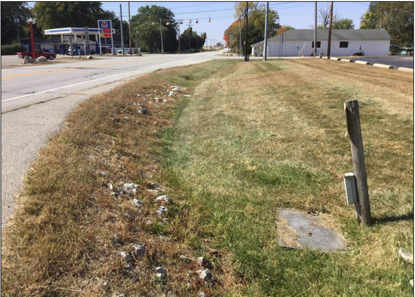
159. Looking west along the north side (WB lane) of SR 32 at the surrounding landscape. Photo taken October 7, 2020.
