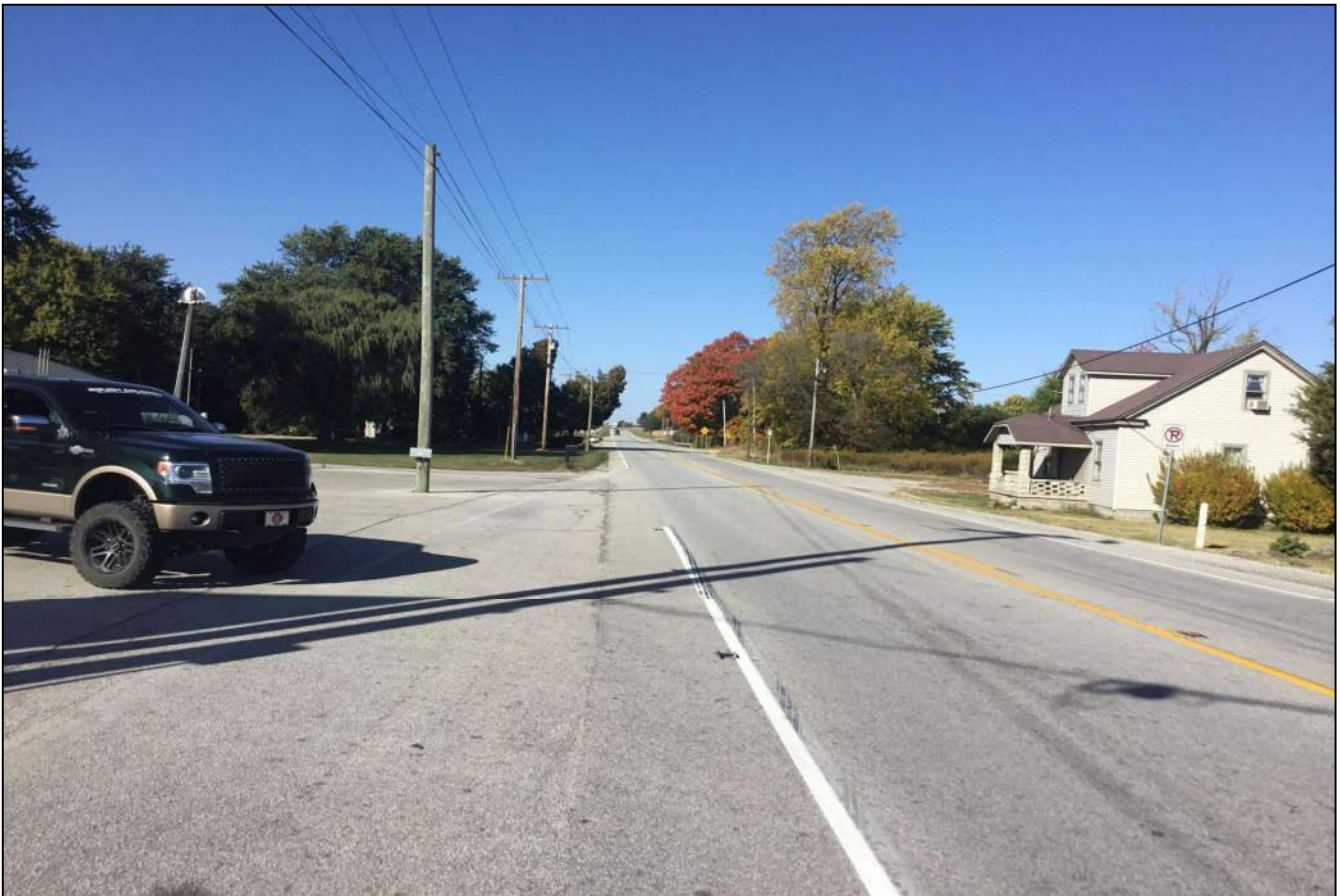
Looking west down SR 32 just west of the SR 75 intersection. The Marathon gas station is located to the left of photo. 161. Des No. 2101655 proposes to install a curbed island at this location to better define the entrance/exit to the gas station to alleviate conflicts for motorists accessing SR 32 from SR 75. Photo taken October 8, 2020.
