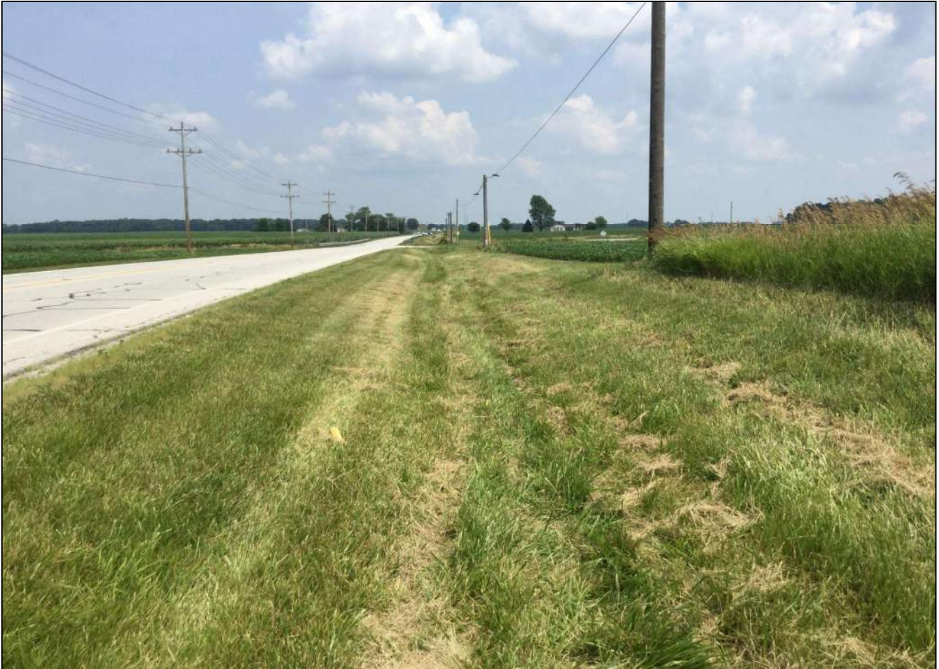
126. Looking east along the south side (EB lane) of SR 32 at the surrounding landscape. Photo taken July 6, 2020.
