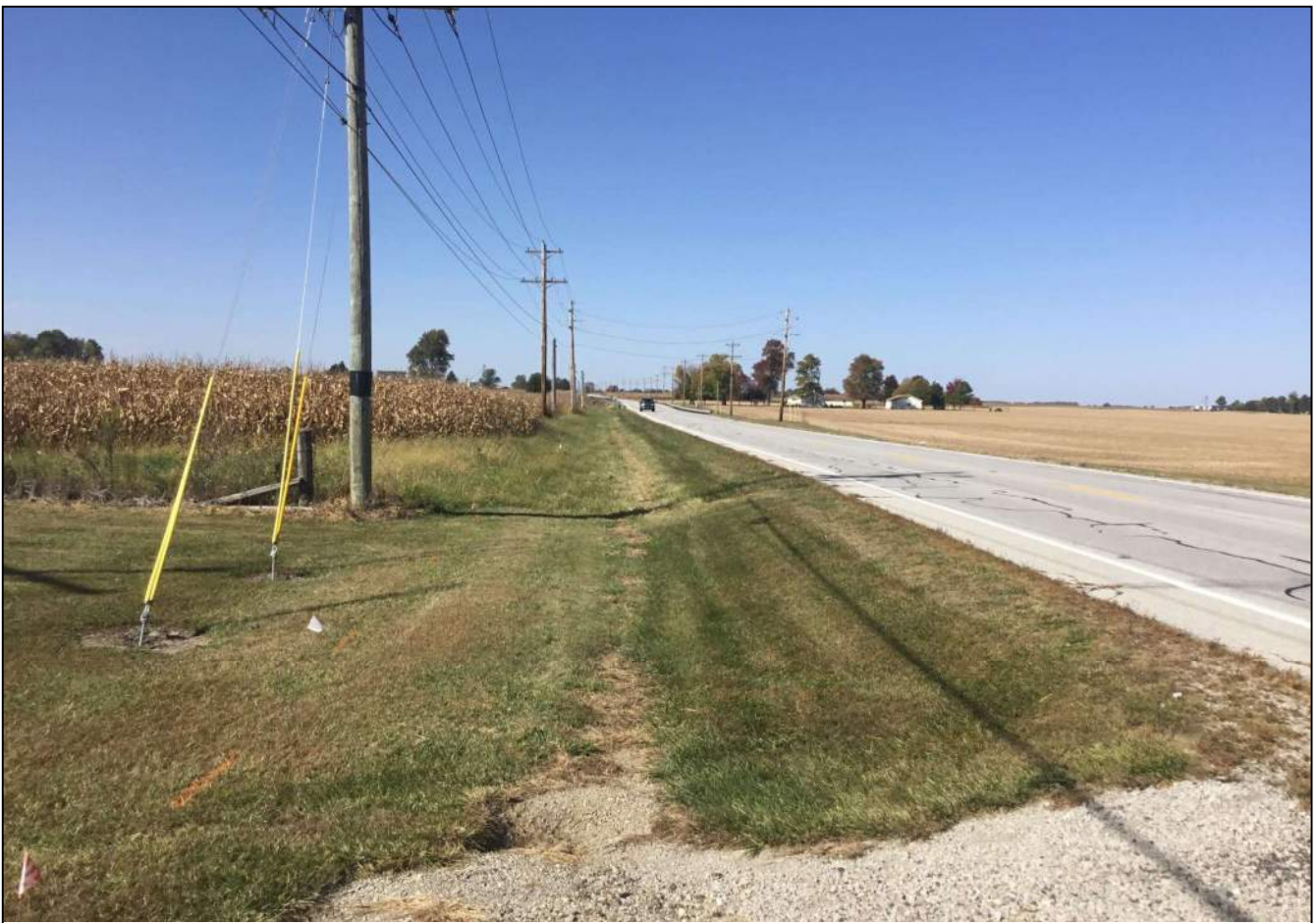
111. Looking west from an access drive to an electric substation along the south side (EB lane) of SR 32 at the surrounding landscape. Photo taken October 8, 2020.
