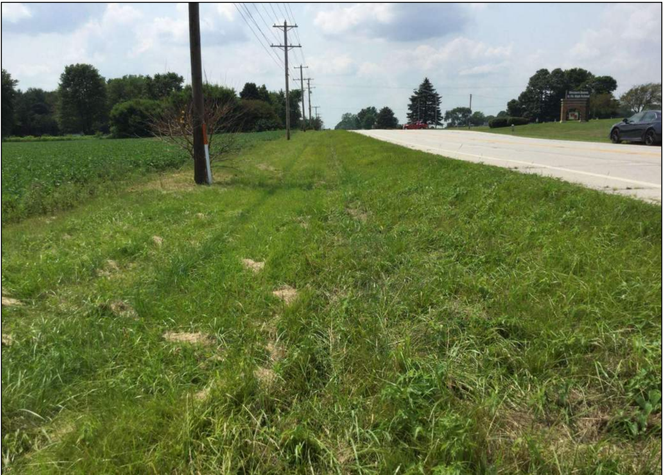
155. Looking west along the south side (EB lane) of SR 32 just west of Structure No. 120. Photo taken July 6, 2021.
