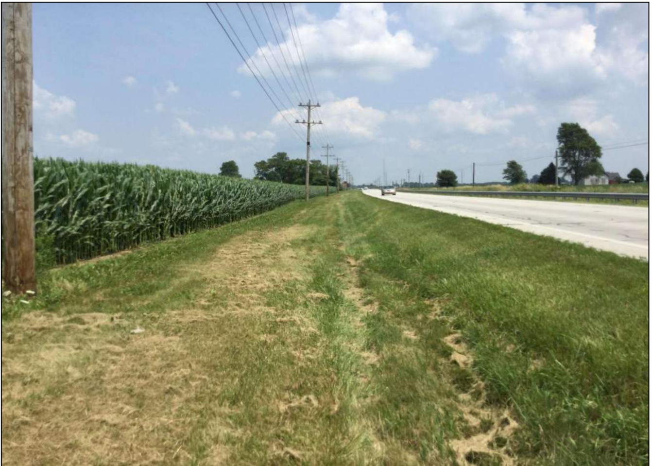
119. Looking east at the surrounding landscape located along the north side (WB) lane of SR 32. Photo taken July 6, 2021.
