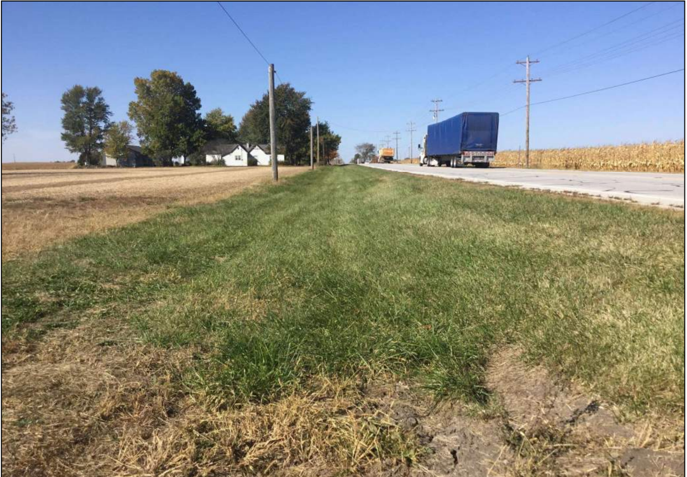
132. Looking west along the south side (EB lane) of SR 32 at the existing landscape just west of Structure No. 123. Photo taken October 8, 2020.
