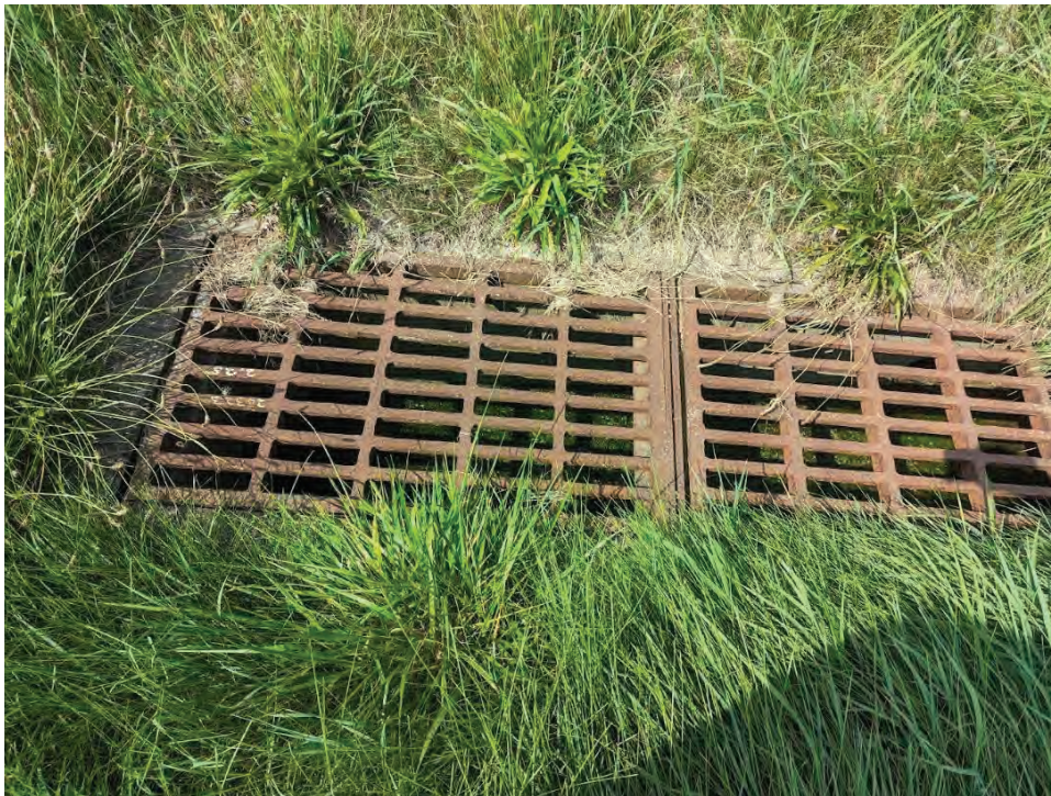
Photograph 48. View of the stormwater inlet basin found at the southern terminus of RSD1. This basin captures flow from RSD1 and outlets to the west into Wetland B.
