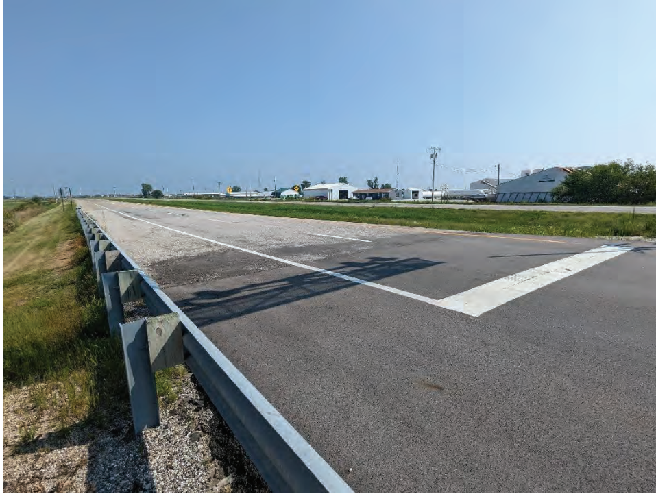
Photograph 7. View of US 41 southbound at the southern terminus of the project area, facing northeast.
