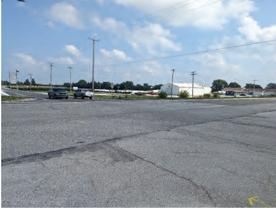
Photograph 3. View of the US 41 and SR 352 intersection, facing southeast.
