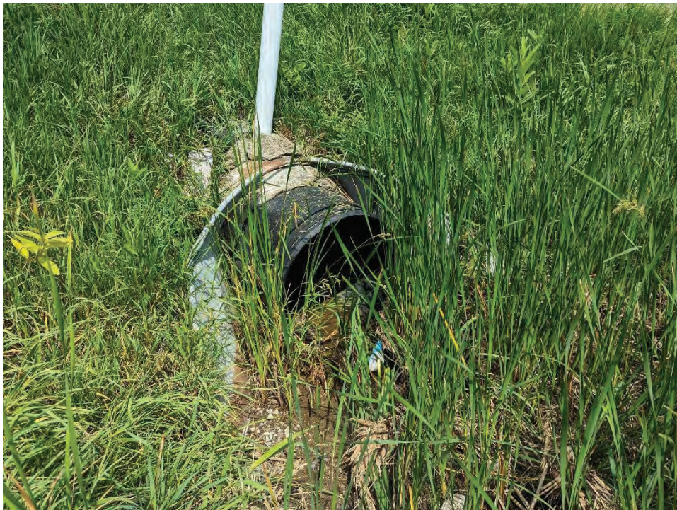
Photograph 12. View of the culvert inlet on the eastern side of the US 41 and SR 352 intersection, facing north.
