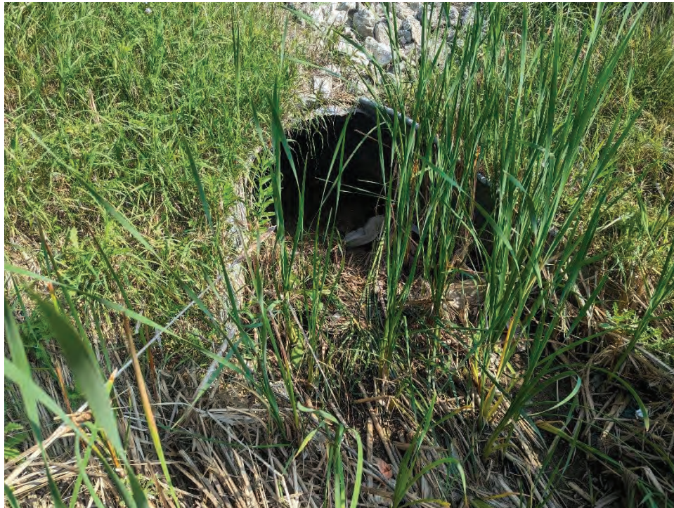
Photograph 13. View of the culvert outlet on the western side of the US 41 and SR 352 intersection, facing north.
