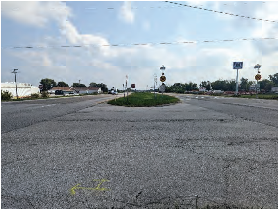
Photograph 2. View of the US 41 and SR 352 intersection, facing south.
