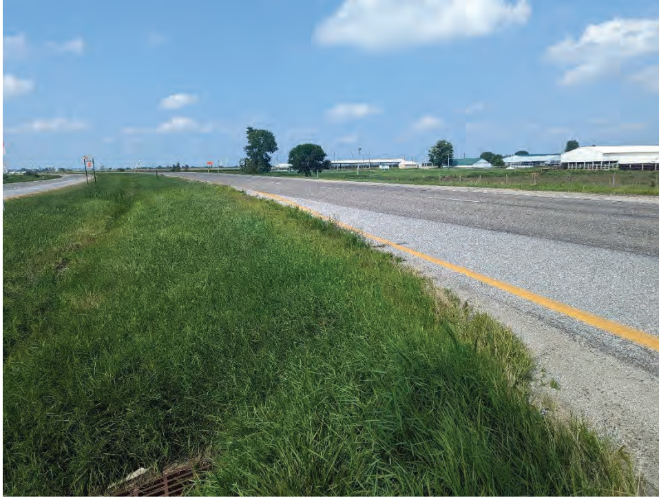
Photograph 5. View of US 41 northbound, facing northeast.
