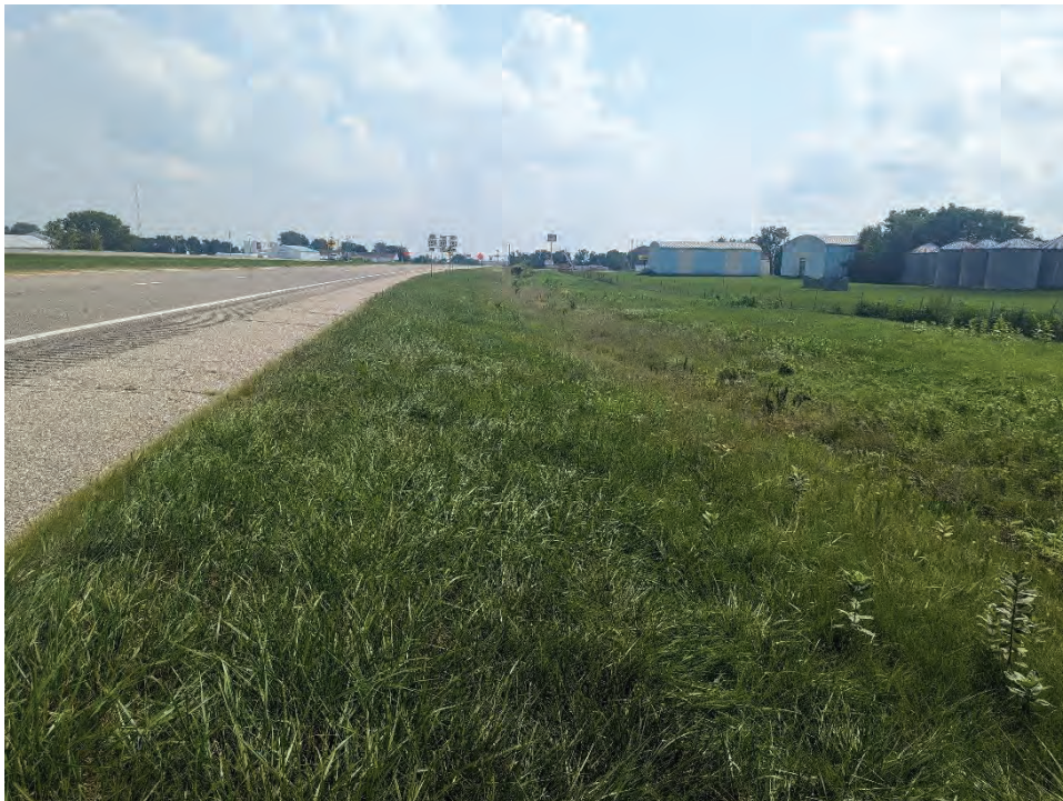
Photograph 10. View of US 41 southbound, facing south at the northern terminus of the project area.
