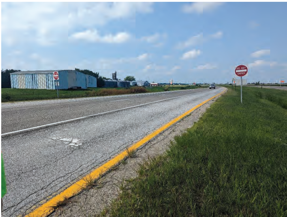
Photograph 6. View of US 41 southbound, facing northwest.
