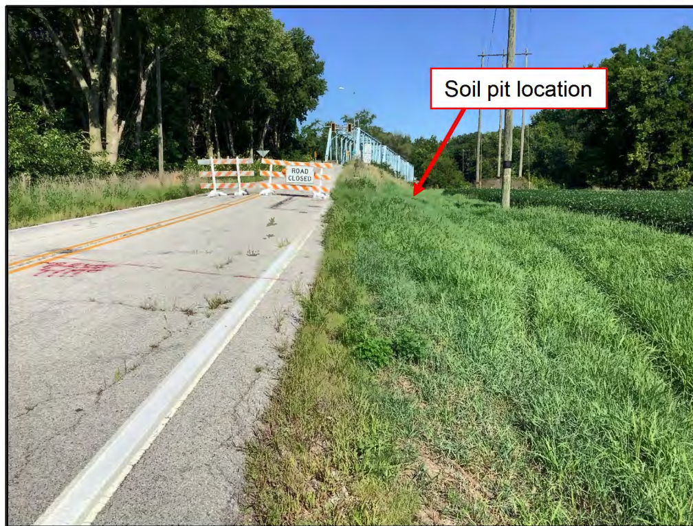
Photo 4: Looking northwest at the structure from the southeastern side of SR 225.
