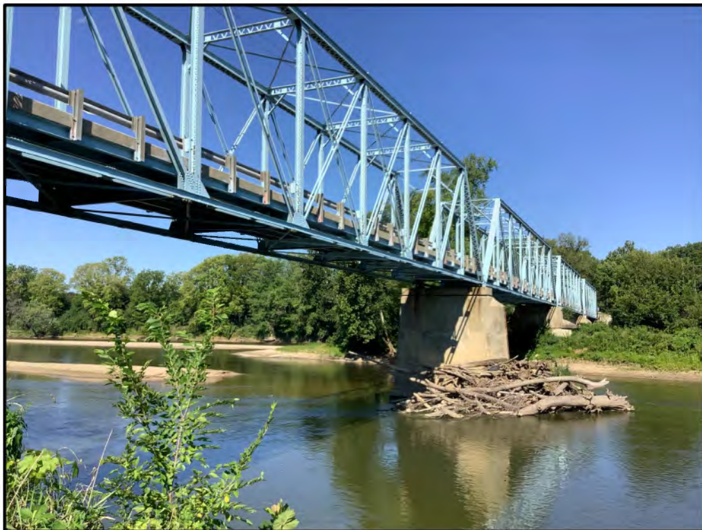
Photo 8: Looking west at the structure from the eastern quadrant.
