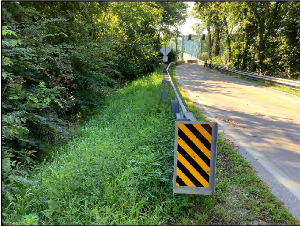
Photo 3: Looking southeast at the structure from the northwestern side of SR 225.
