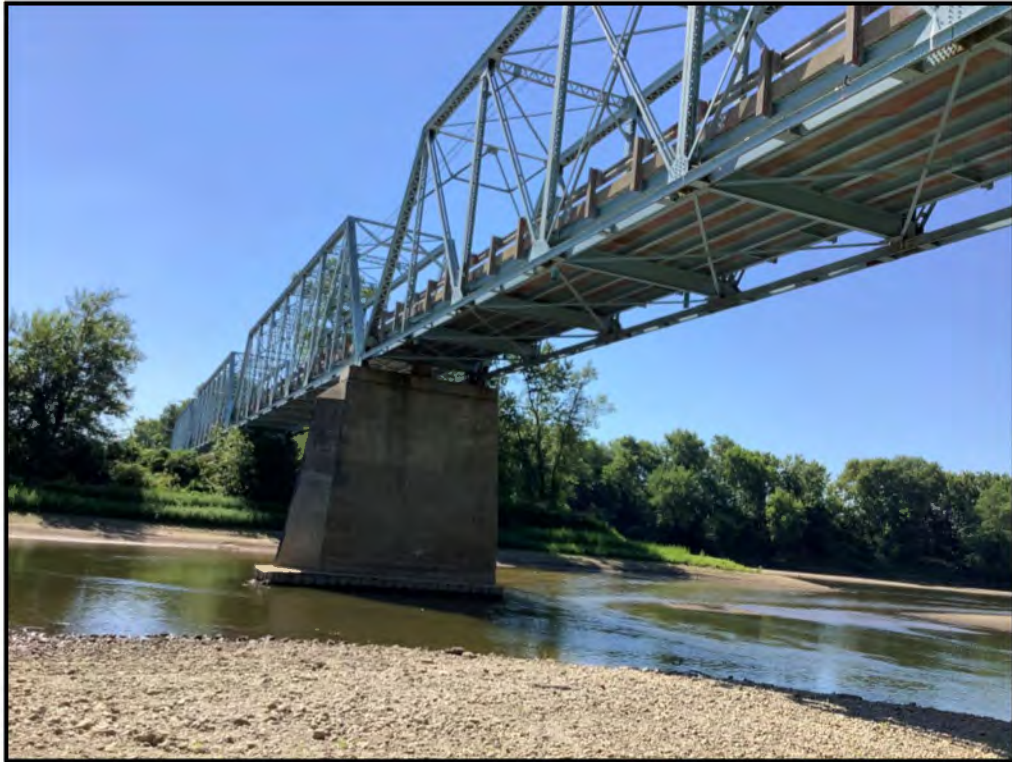
Photo 9: Looking southeast at the structure from the northwest quadrant.
