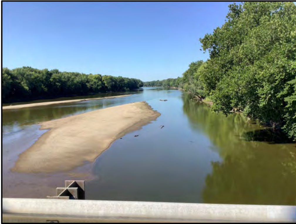
Photo 11: Looking southwest (downstream) from the top of the structure.
