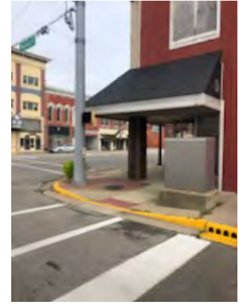
Corner of East Walnut and Meridian looking north.
