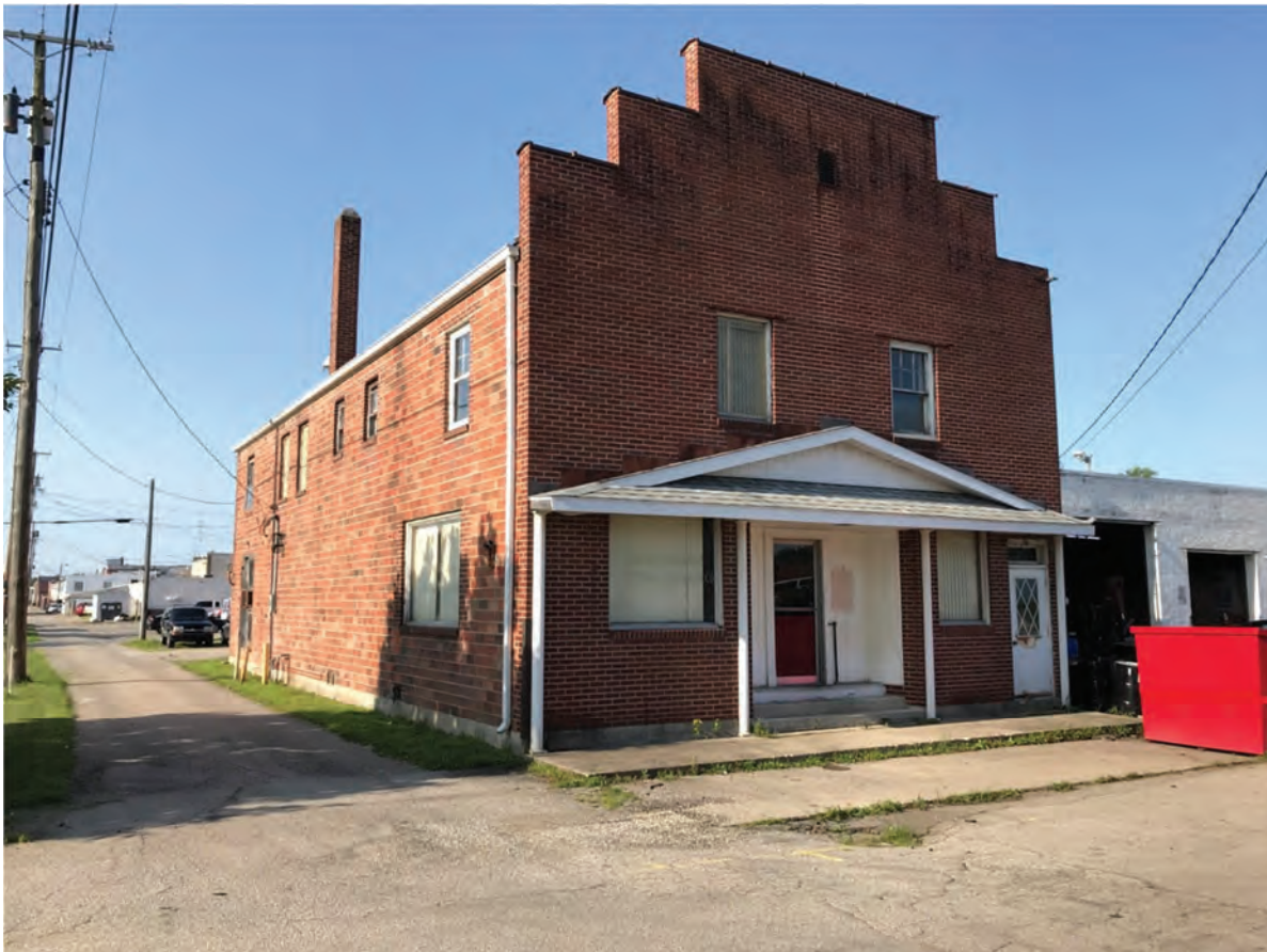
162. Looking SW at Lochmueller #46, Contributing, 113 E. Race Street
