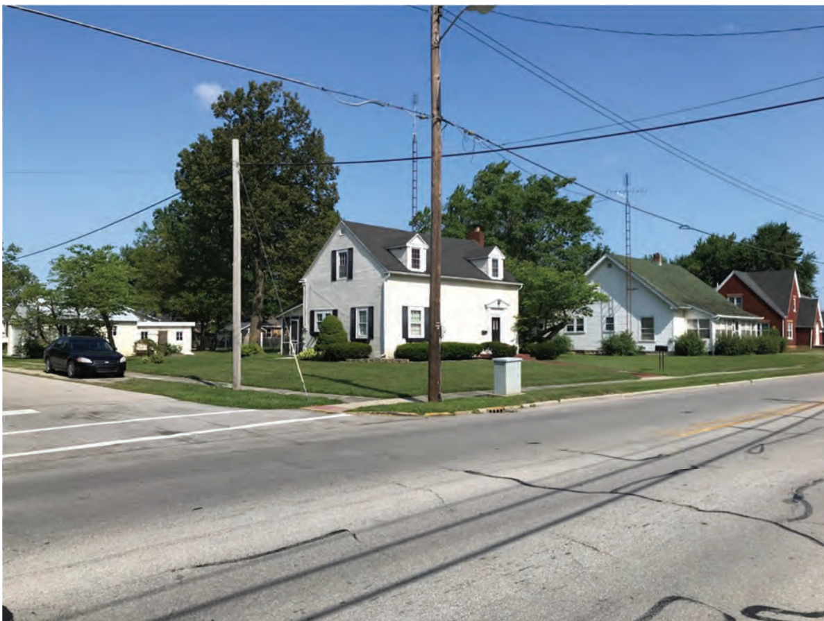
42. Looking NW at the intersection of US 27 (Meridian Street) and W. 10th Street
