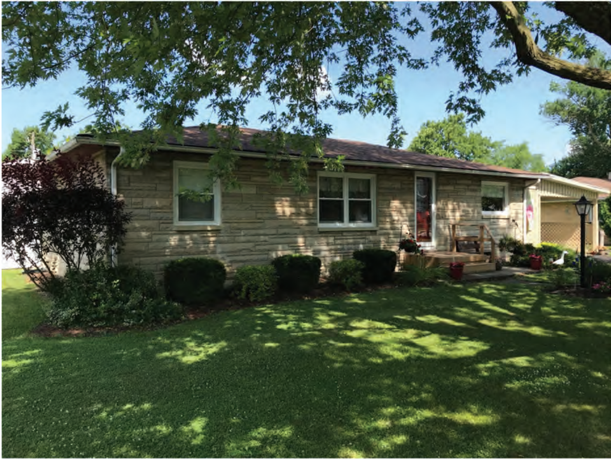
35. Looking NW at Lochmueller #19, Contributing, 1216 S. Meridian Street
