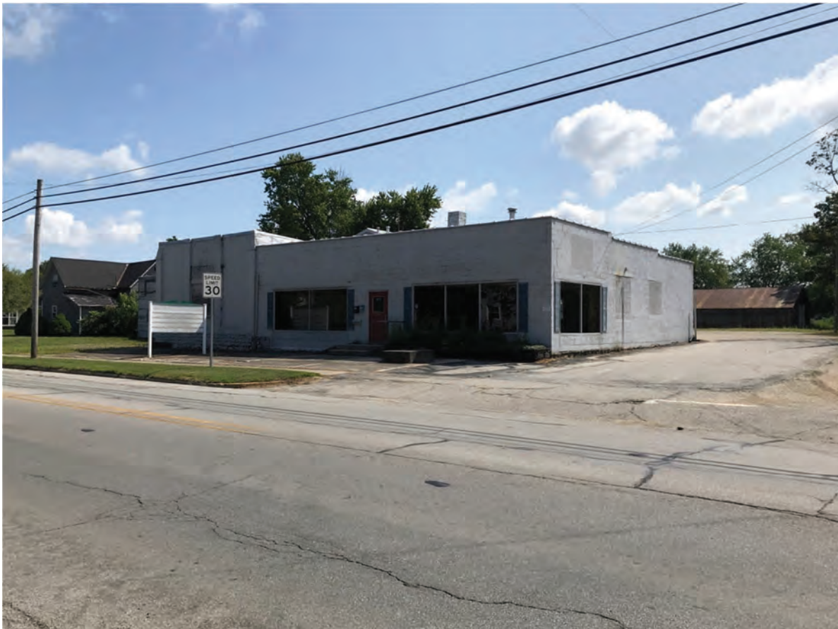
48. Looking NE at the intersection of US 27 (Meridian Street) and W. 9th Street
