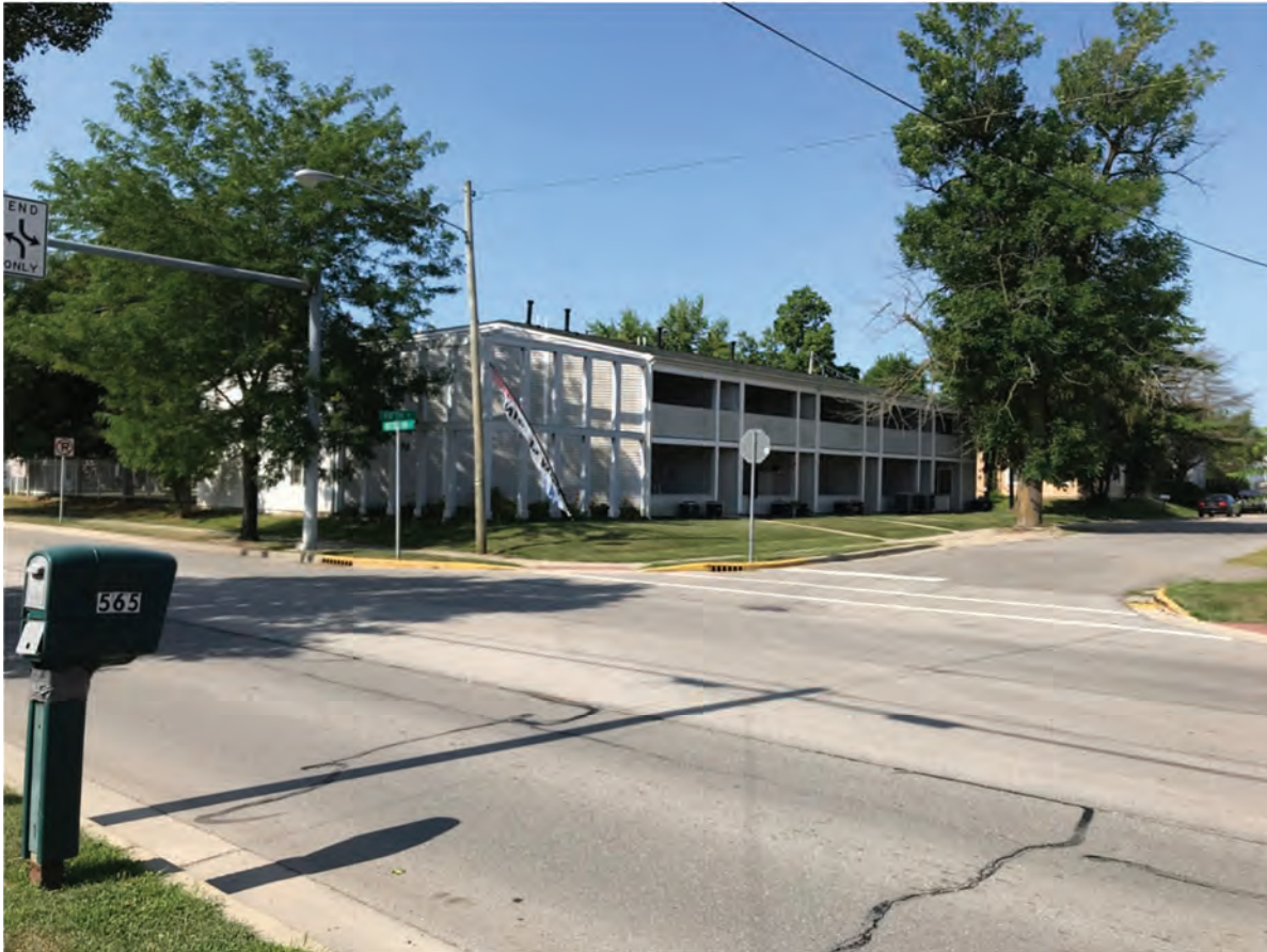
85. Looking SW at the intersection of US 27 (Meridian Street) and 5th Street
