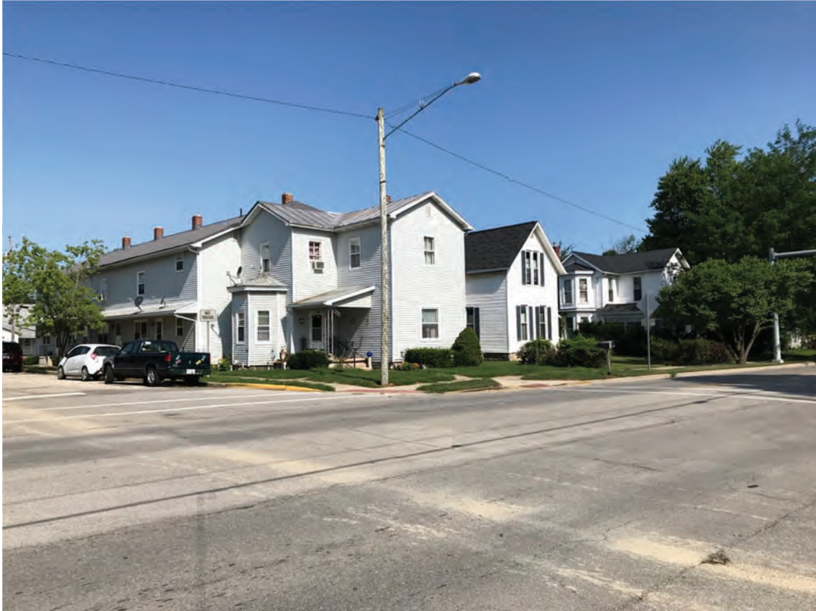
107. Looking NW at the intersection of US 27 (Meridian Street) and 3rd Street
