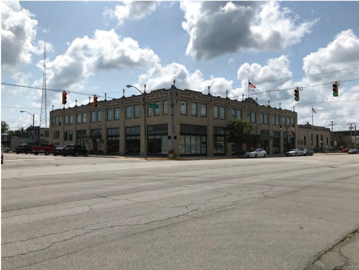
135. Looking SE in Portland Commercial Historic District (NR-1299) at the intersection of US 27 (Meridian Street) and Main Street
