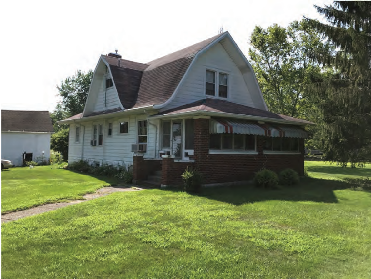
33. Looking SE at Lochmueller #17, Contributing, 1229 S. Meridian Street
