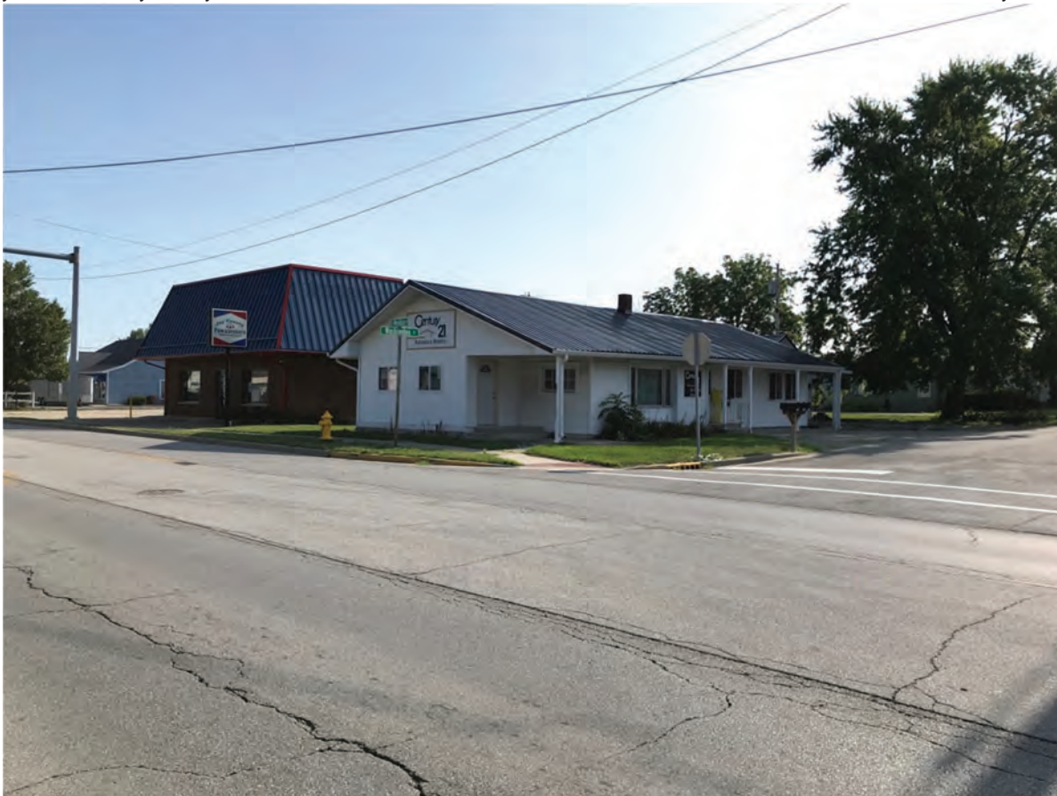
193. Looking NE at the intersection of US 27 (Meridian Street) and Washington Street
