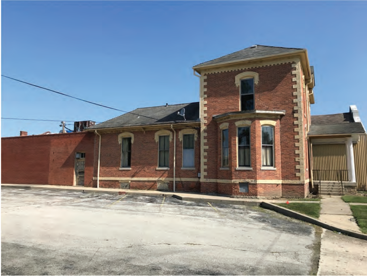
87. Looking NNW at IHSSI #075-521-33091, Elias Shewalter House, Outstanding, 500 S. Meridian Street,
