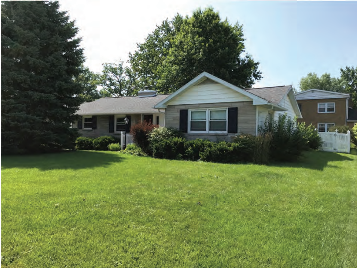
31. Looking SE at Lochmueller #15, Contributing, 101 W. 12th Street
