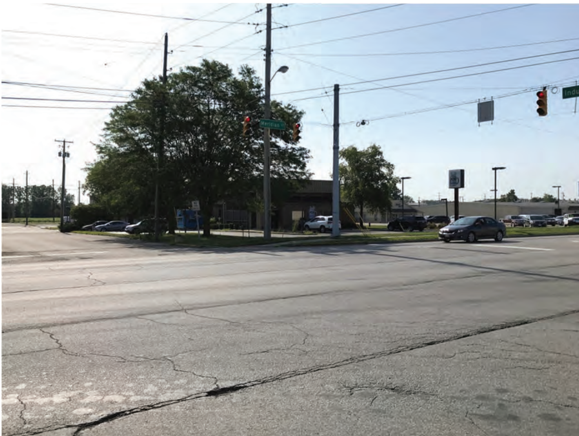
210. Looking SE at the intersection of US 27 (Meridian Street) and Industrial Drive
