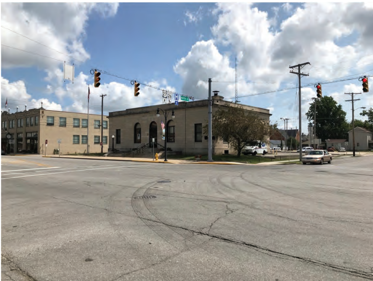
126. Looking NE in Portland Commercial Historic District (NR-1299) at the intersection of US 27 (Meridian Street) and Water Street
