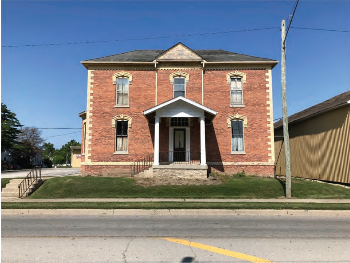
89. Looking W at IHSSI #075-521-33091, Elias Shewalter House, Outstanding, 500 S. Meridian Street
