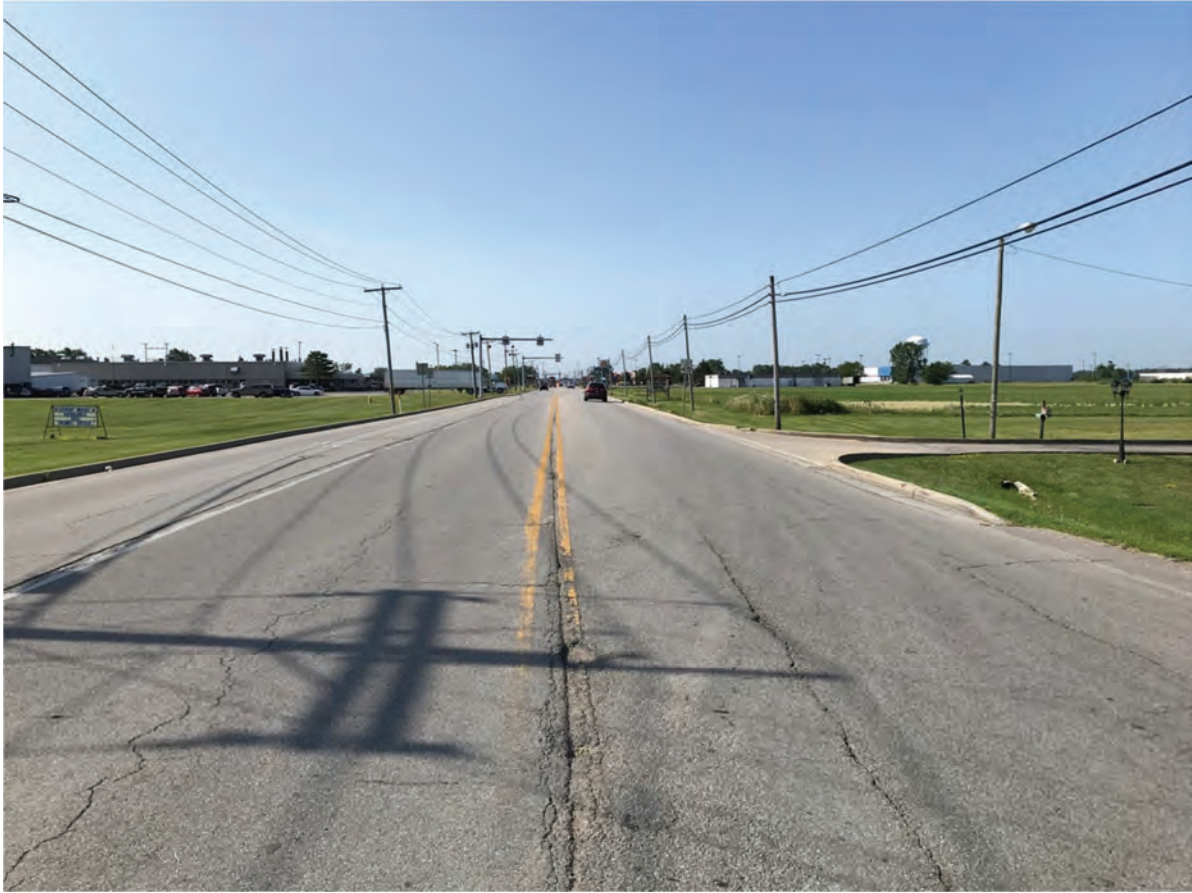
217. Looking S at the N end of the project limits on US 27 (Meridian Street)
