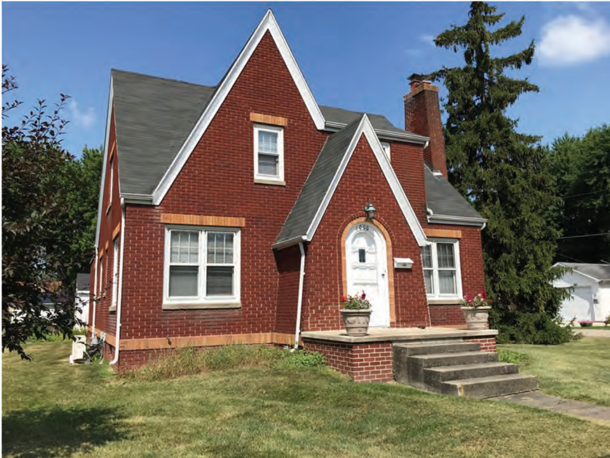
47. Looking NW at IHSSI #075-521-33095, Contributing, 1000 S. Meridian Street
