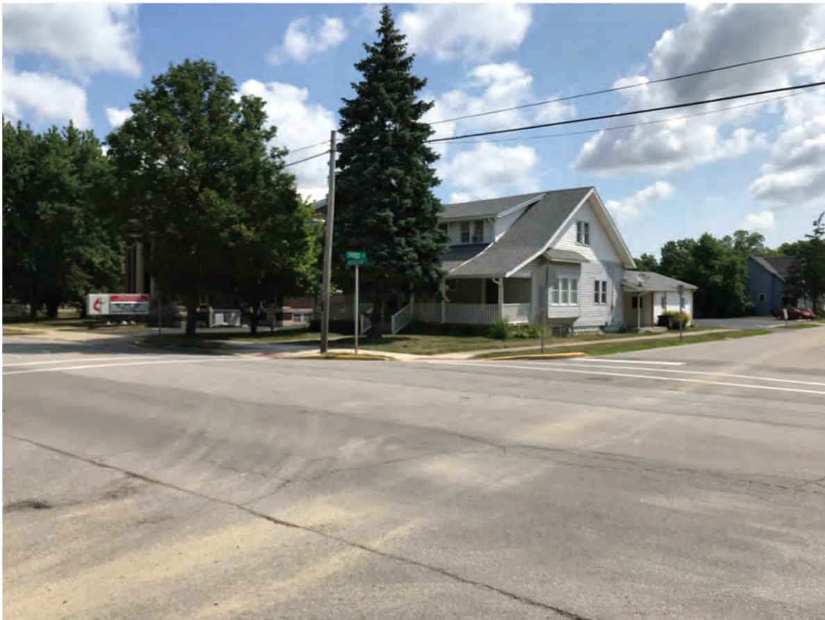
104. Looking NE at the intersection of US 27 (Meridian Street) and 3rd Street
