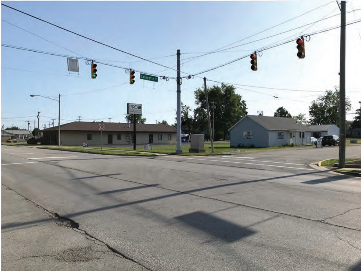
197. Looking NE at the intersection of US 27 (Meridian Street) and Lafayette Street
