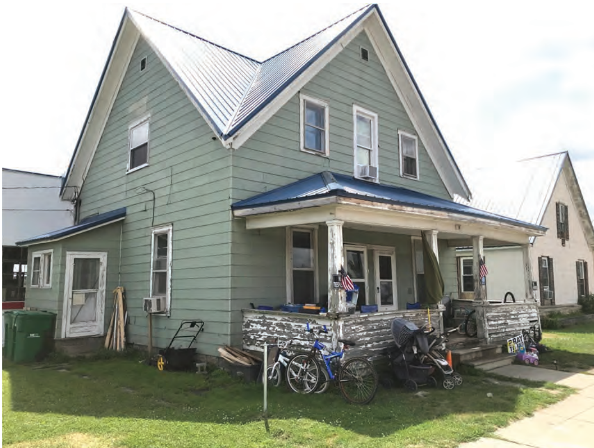
164. Looking SE at Lochmueller #48, Contributing, 525 N. Meridian Street
