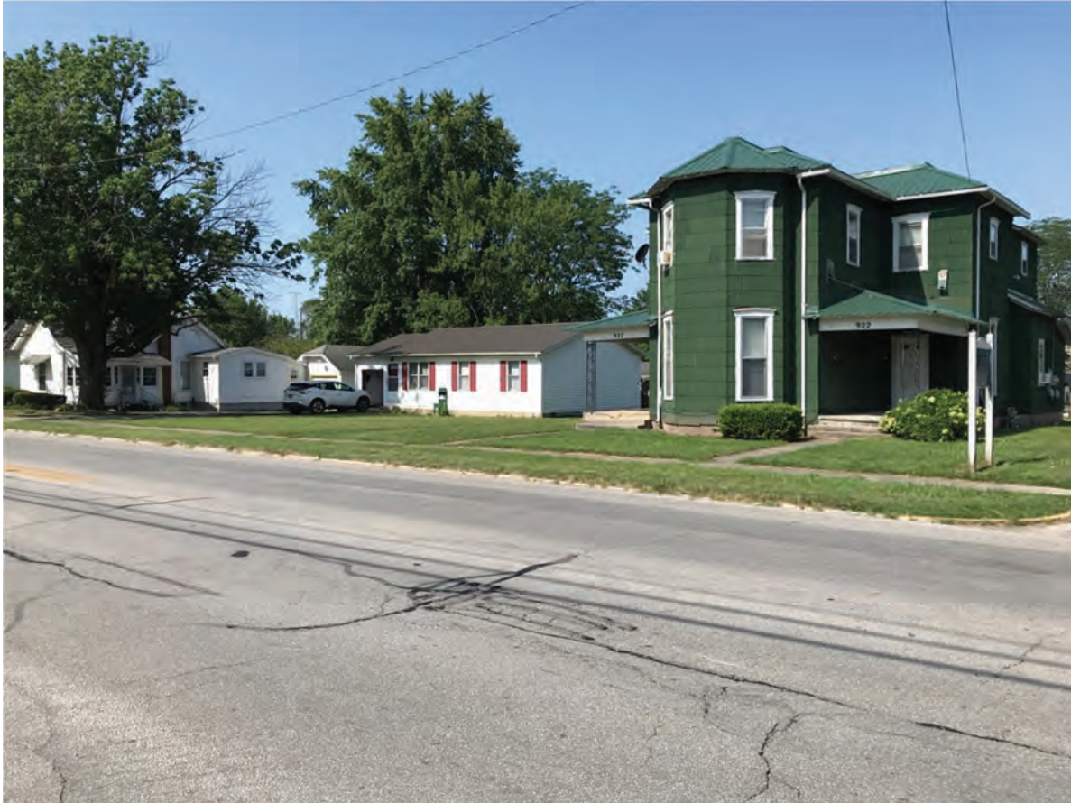
63. Looking SW at the intersection of US 27 (Meridian Street) and Elder Street
