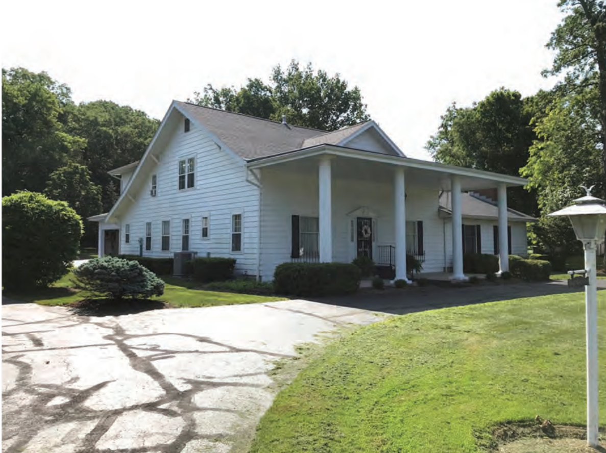
37. Looking SE at Lochmueller #21, Contributing, 1011 S. Meridian Street
