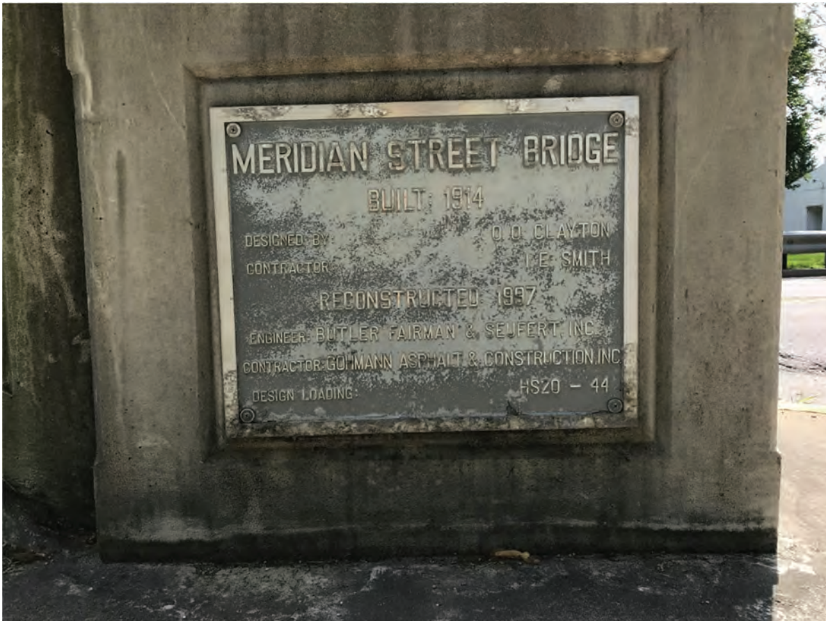
118. Looking E in Portland Commercial Historic District (NR-1299) at plaque on IHSSI #075-521-33086, Meridian Street Bridge, Outstanding
