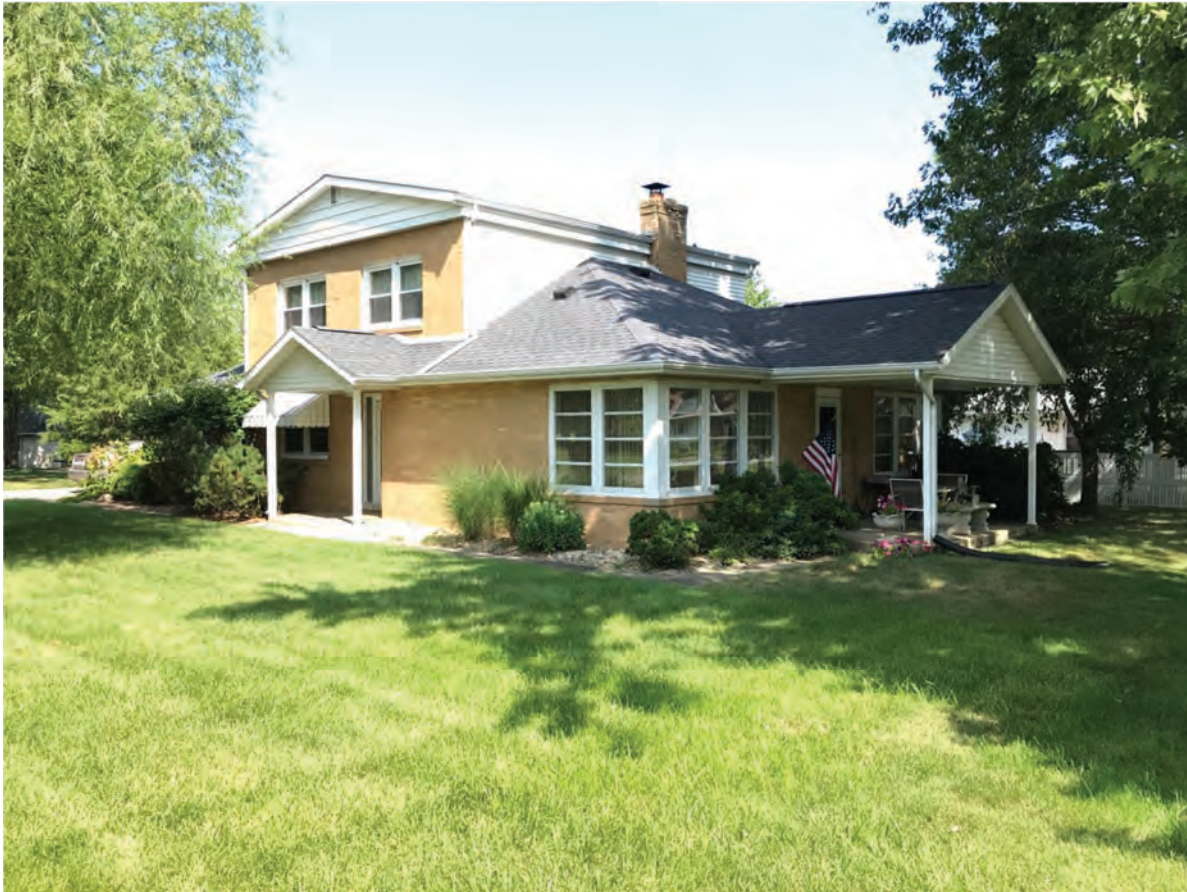
25. Looking NW at Lochmueller #13, Contributing, 104 Meridian Heights
