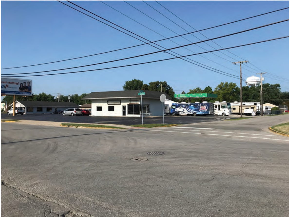
207. Looking SW at the intersection of US 27 (Meridian Street) and Lincoln Street
