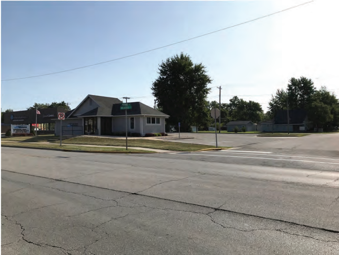
181. Looking NE at the intersection of US 27 (Meridian Street) and Adams Street
