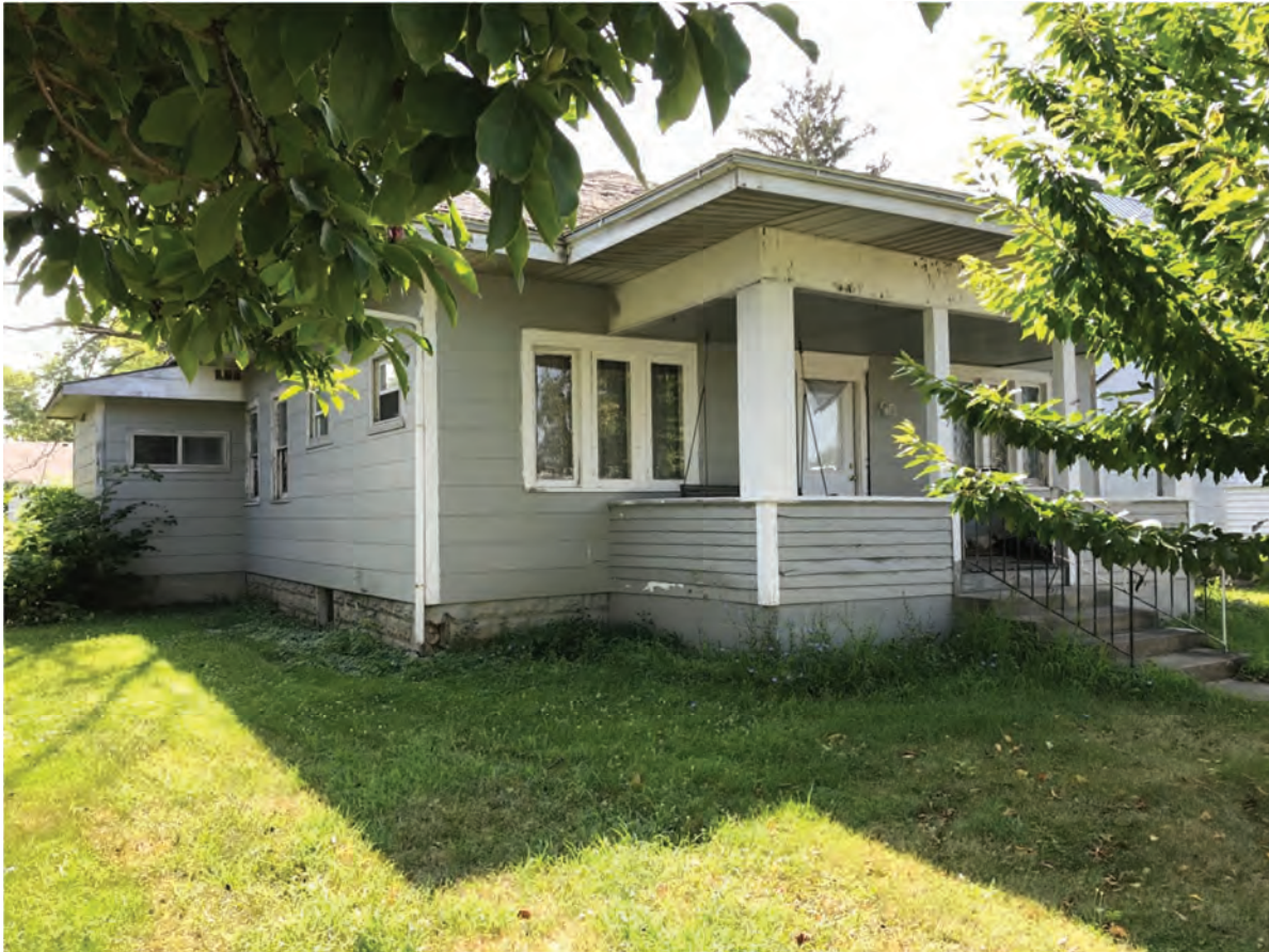
99. Looking SE at Lochmueller #35, Contributing, 439 S Meridian Street
