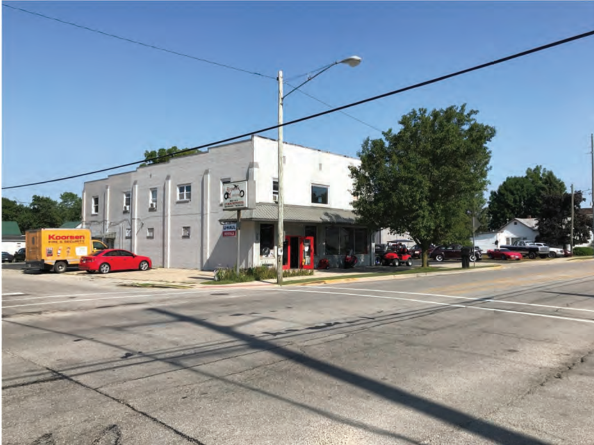
75. Looking NW at the intersection of US 27 (Meridian Street) and 7th Street
