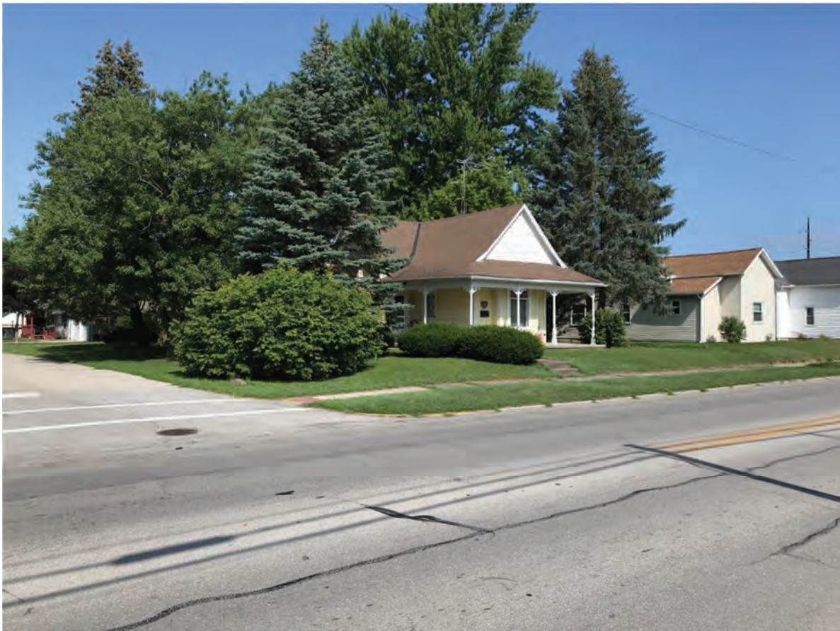
68. Looking NW at the intersection of US 27 (Meridian Street) and 8th Street
