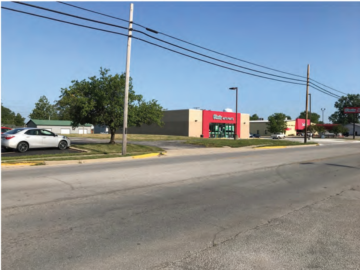
188. Looking NW at the intersection of US 27 (Meridian Street) and Baker Street
