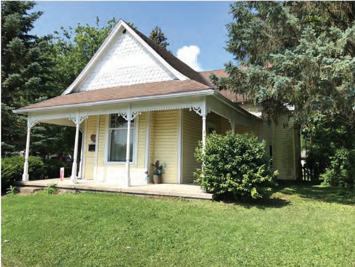
69. Looking SW at IHSSI #075-521-33094, Notable, 834 S. Meridian Street, National Register-eligible
