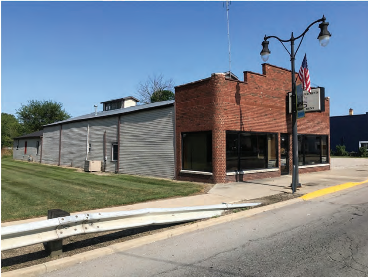
123. Looking NW in Portland Commercial Historic District (NR-1299) at Lochmueller #43, Contributing, 240 S. Meridian Street
