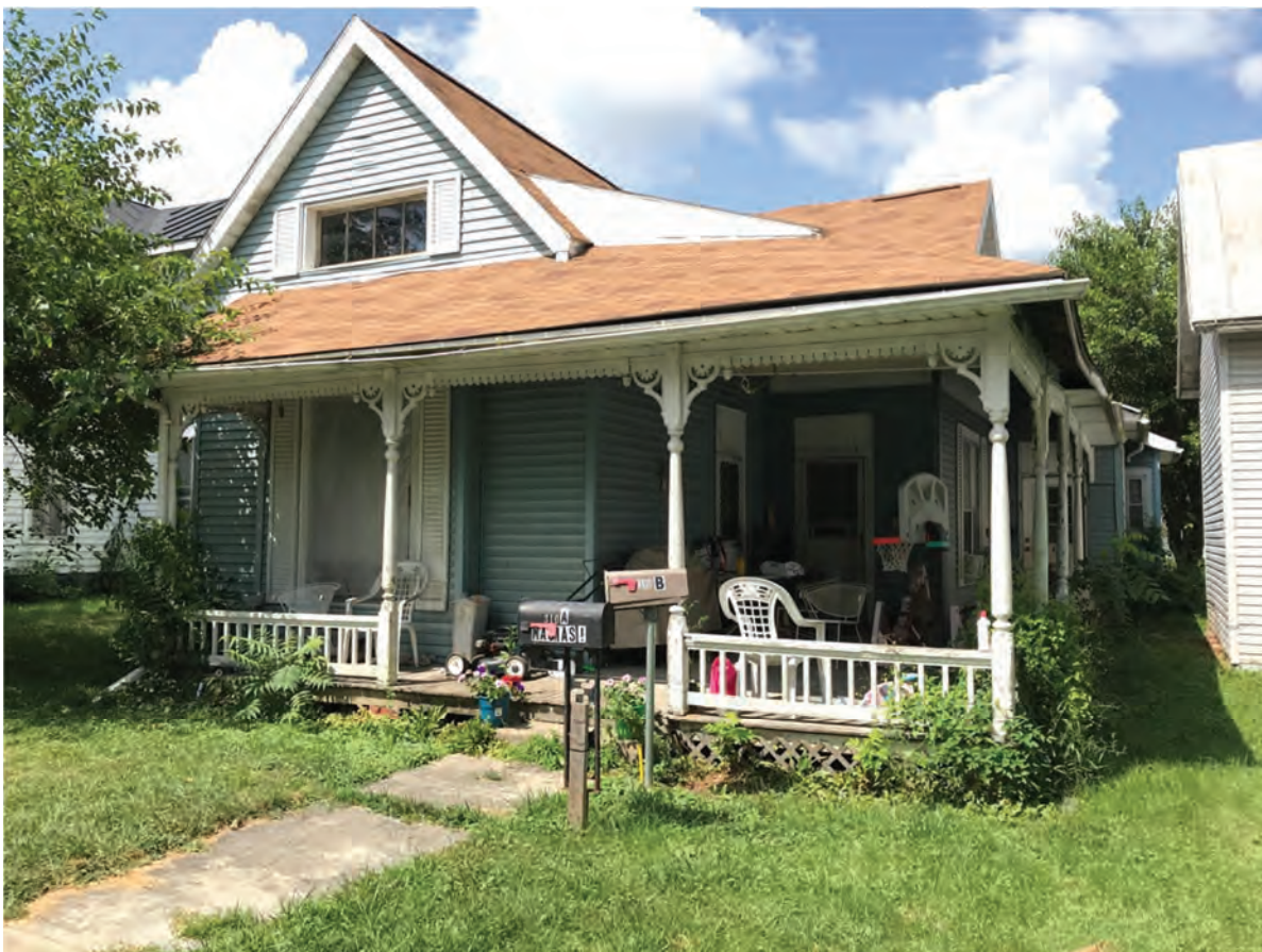
112. Looking SW at Lochmueller #41, Contributing, 310 S. Meridian Street
