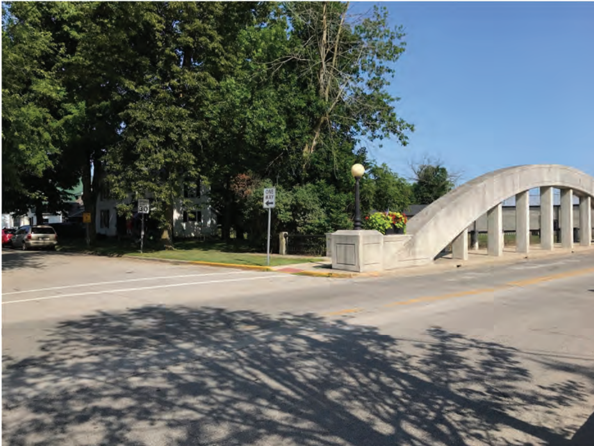
117. Looking NW at the intersection of US 27 (Meridian Street) and 2nd Street
