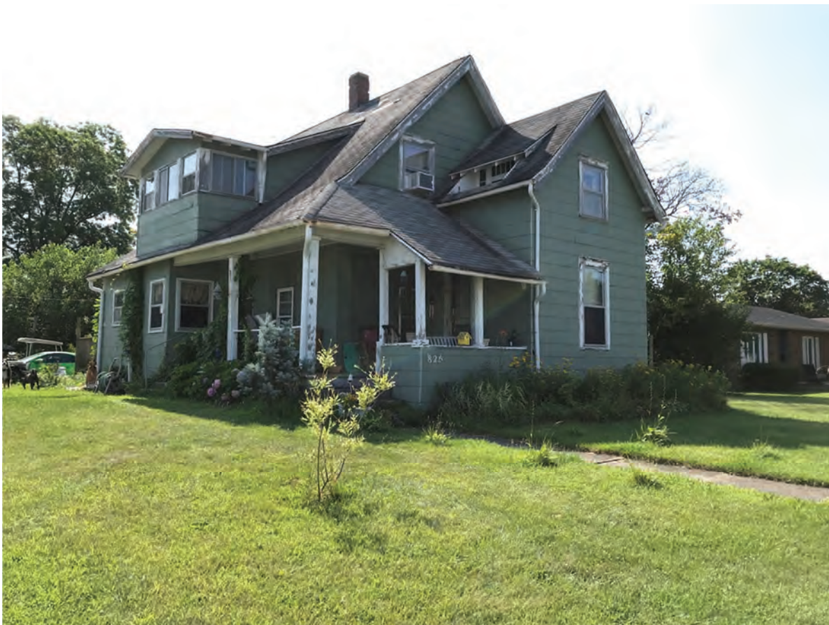
70. Looking SE at Lochmueller #28, Contributing, 825 S. Meridian Street
