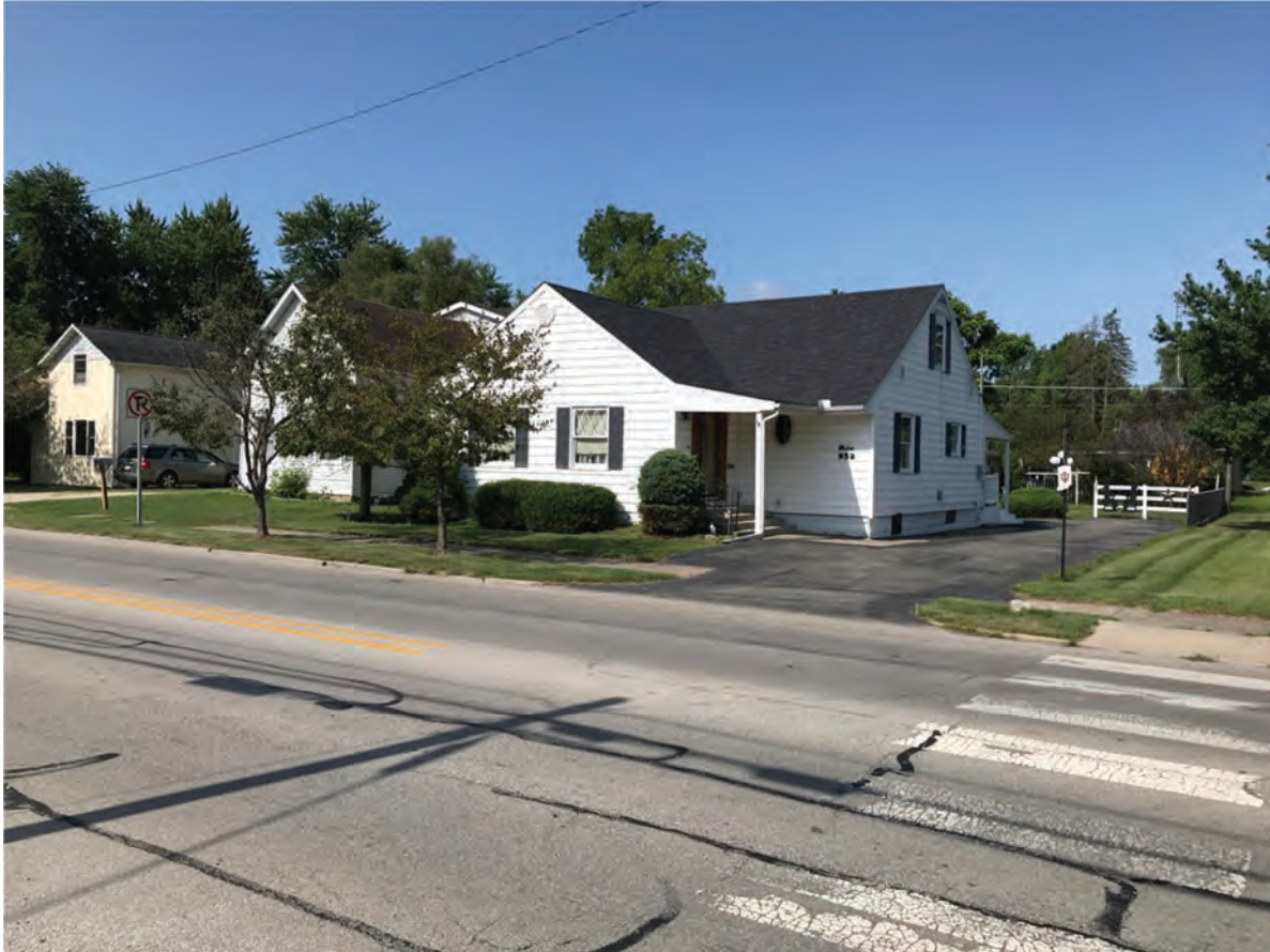
55. Looking SW at the intersection of US 27 (Meridian Street) and Clark Street
