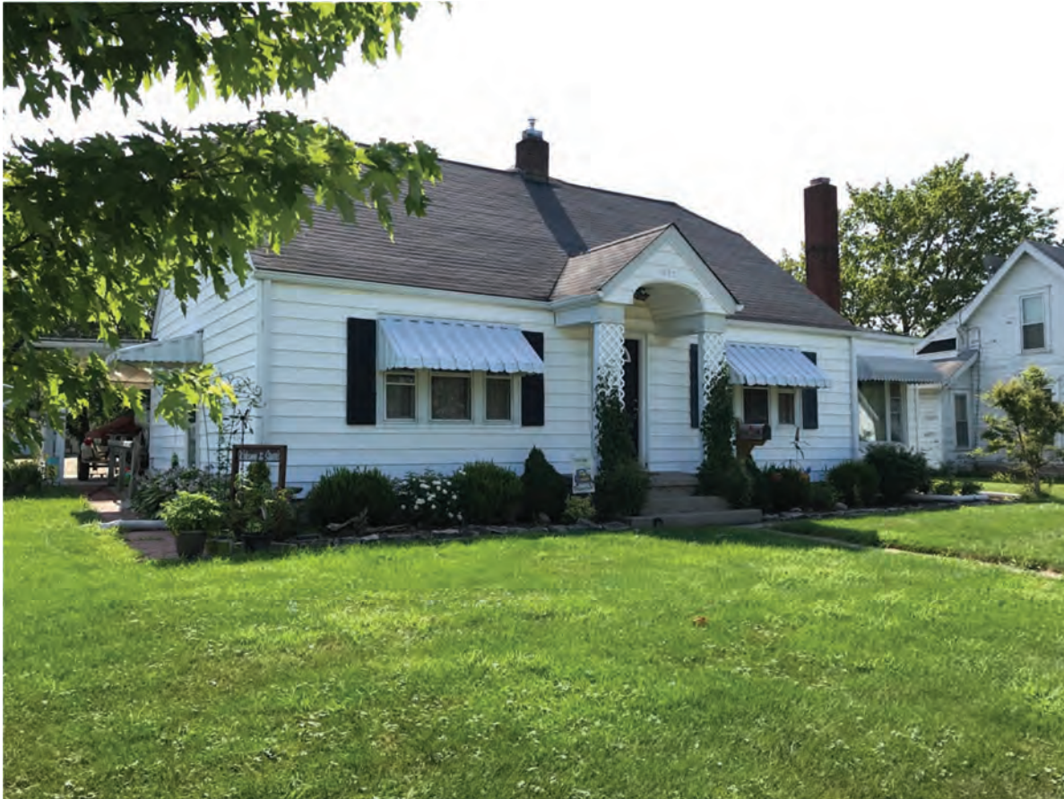
59. Looking SE at Lochmueller #26, Contributing, 903 S. Meridian Street
