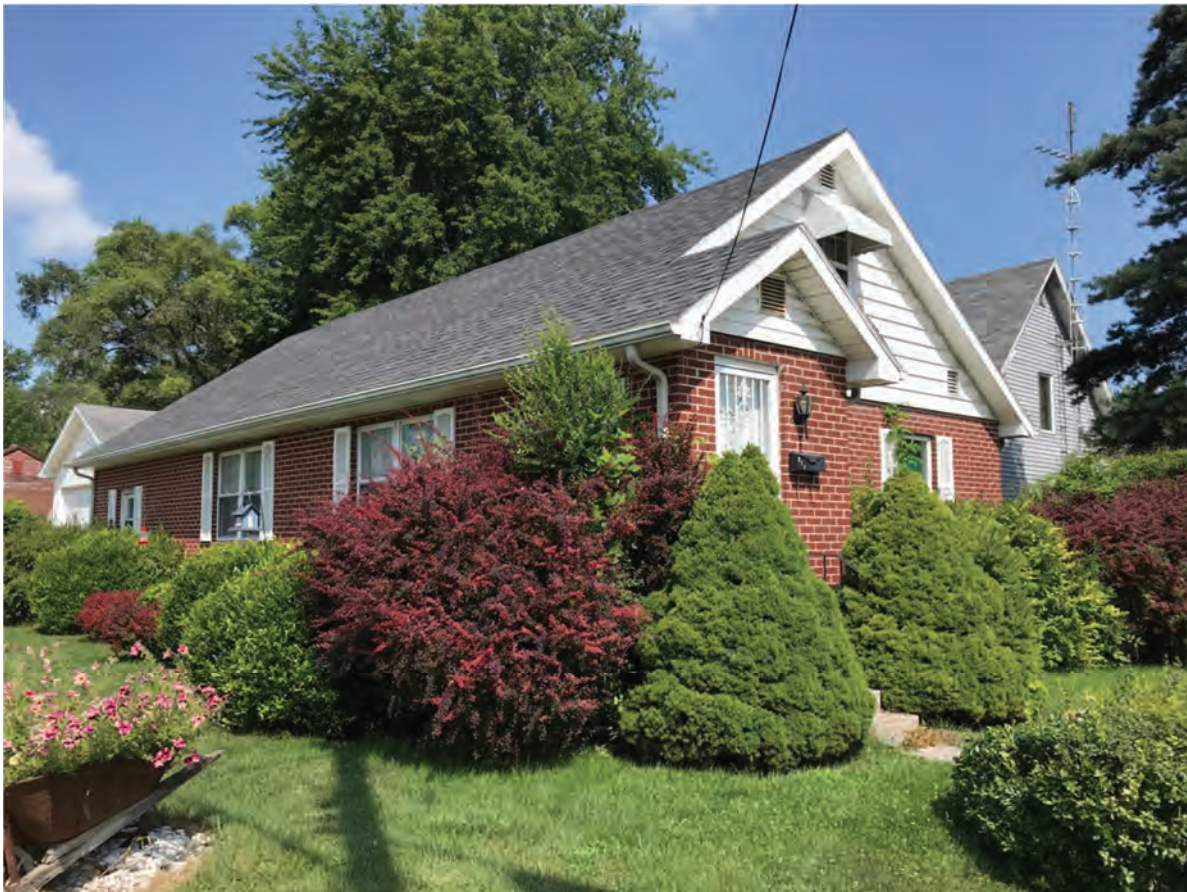
52. Looking NW at Lochmueller #23, Contributing, 974 S. Meridian Street
