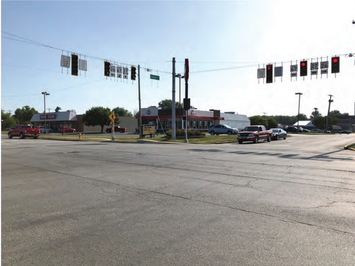
171. Looking NE at the intersection of US 27 (Meridian Street) and Votaw Street
