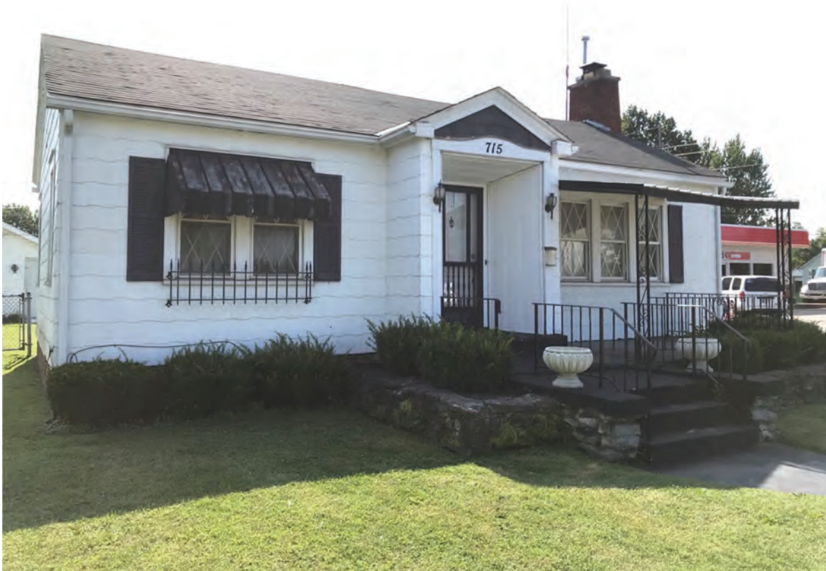
76. Looking SE at Lochmueller #30, Contributing, 715 S. Meridian Street
