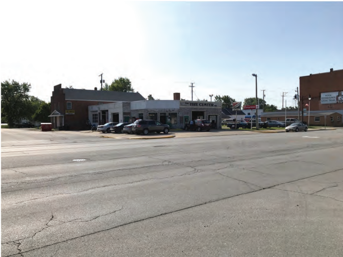
158. Looking SE at the intersection of US 27 (Meridian Street) and Race Street
