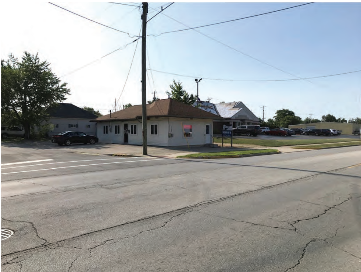
194. Looking SE at the intersection of US 27 (Meridian Street) and Washington Street
