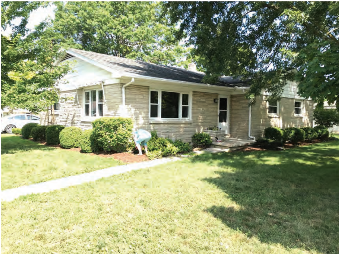
30. Looking NW at Lochmueller #14, Contributing, 1224 S. Meridian Street
