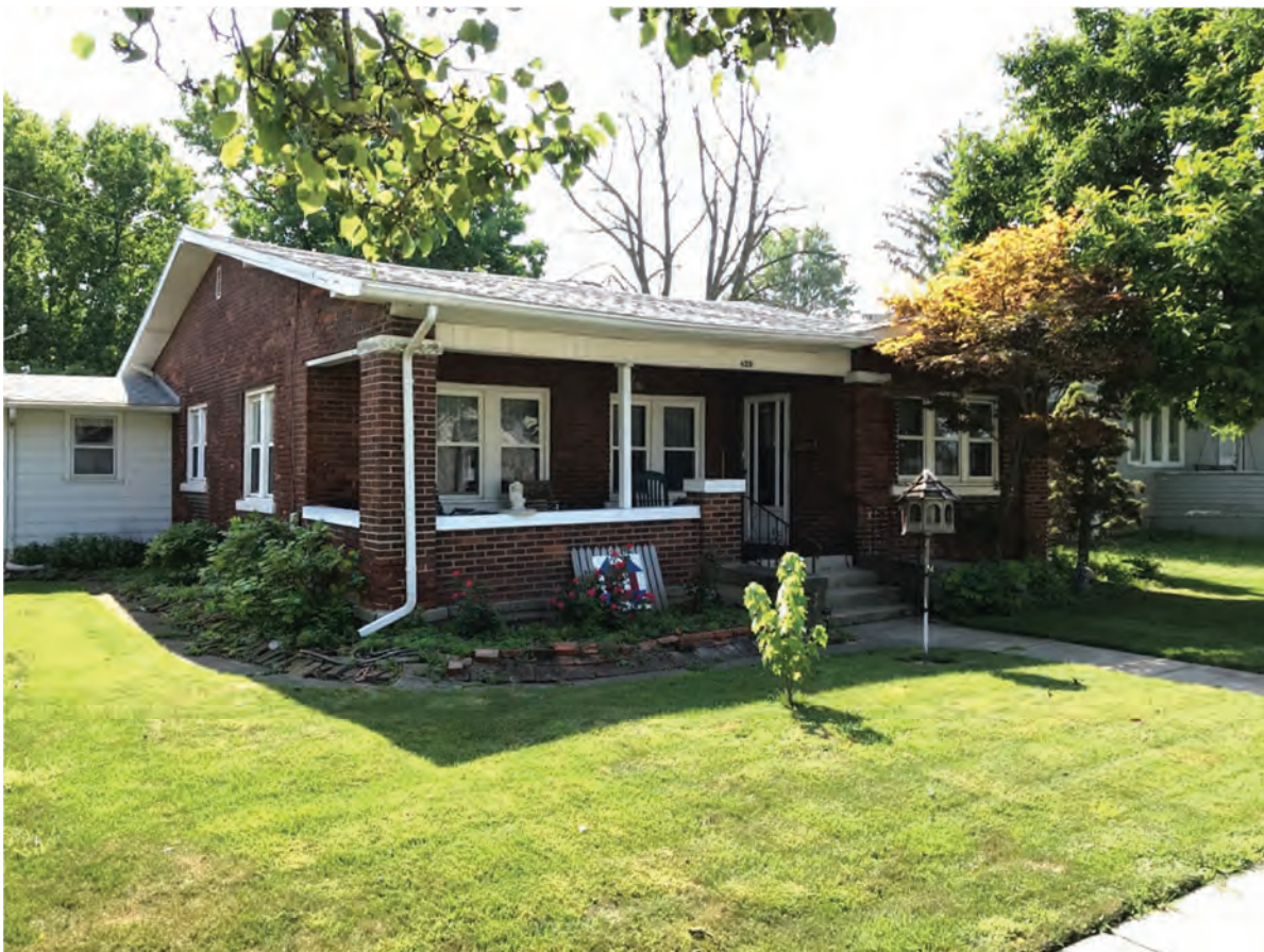
100. Looking SE at Lochmueller #36, Contributing, 429 S. Meridian Street
