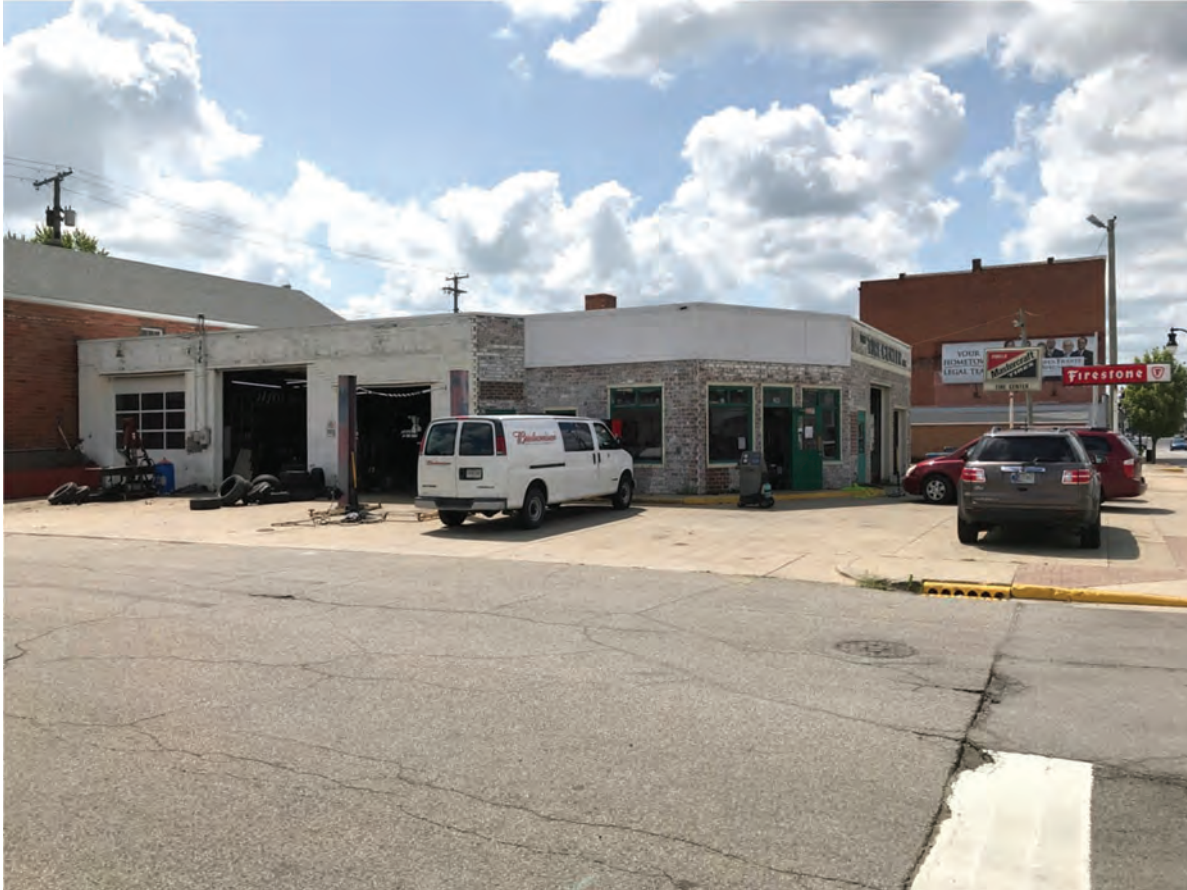
161. Looking SE at Lochmueller #45, Contributing, 421 N. Meridian Street
