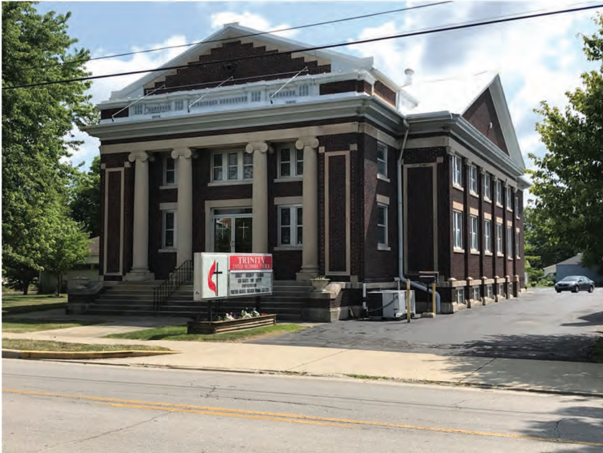
109. Looking NE at IHSSI #075-521-33088, First United Brethren Church, Notable, 323 S. Meridian Street, National Register-eligible
