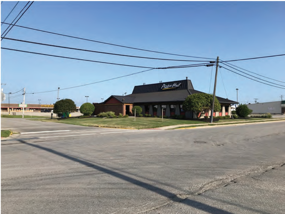
208. Looking NW at the intersection of US 27 (Meridian Street) and Lincoln Street
