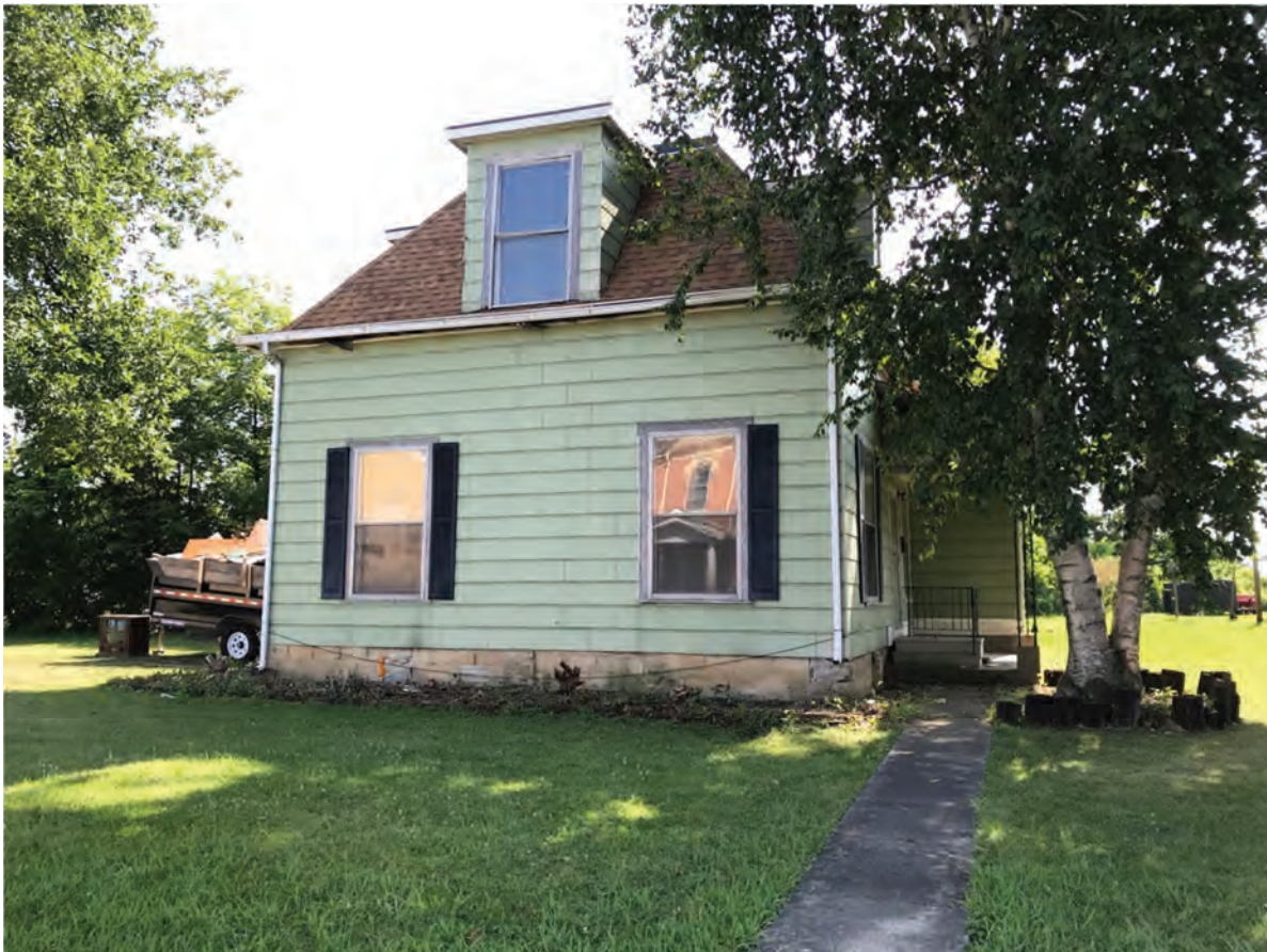
88. Looking NNE at Lochmueller #33, Contributing, 557 S. Meridian Street
