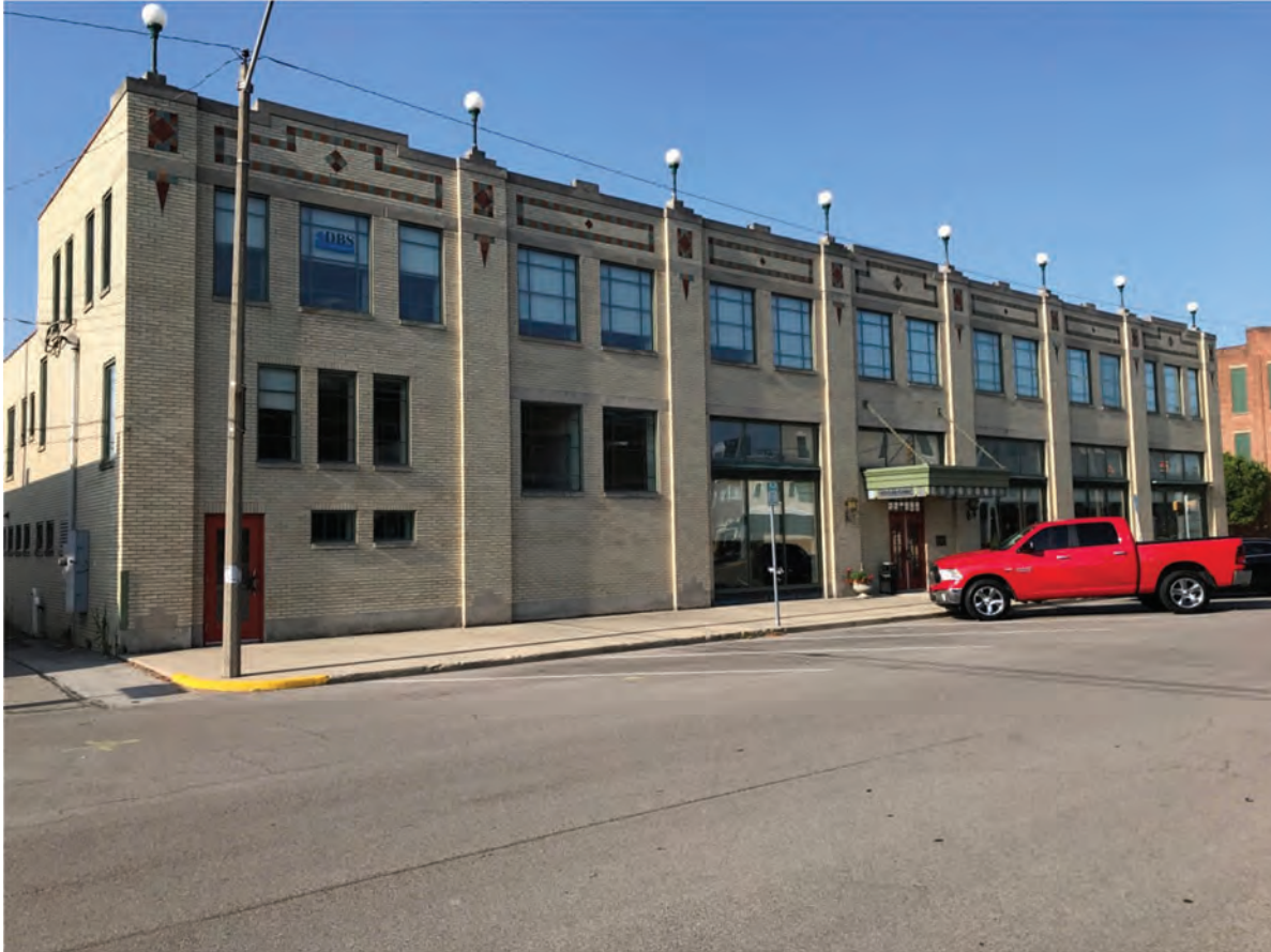
139. Looking SW in Portland Commercial Historic District (NR-1299) at IHSSI #075-521-31058, Weiler Building, Outstanding, 101-107 S. Meridian Street
