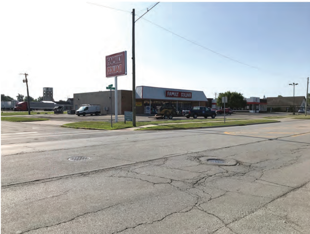
176. Looking SE at the intersection of US 27 (Meridian Street) and McNeil Street
