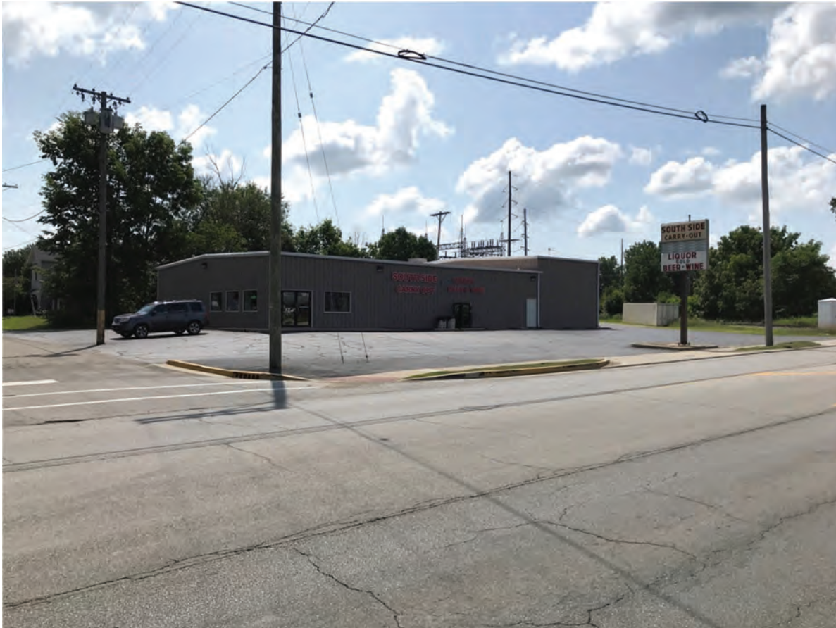
91. Looking SE at the intersection of US 27 (Meridian Street) and Union Street
