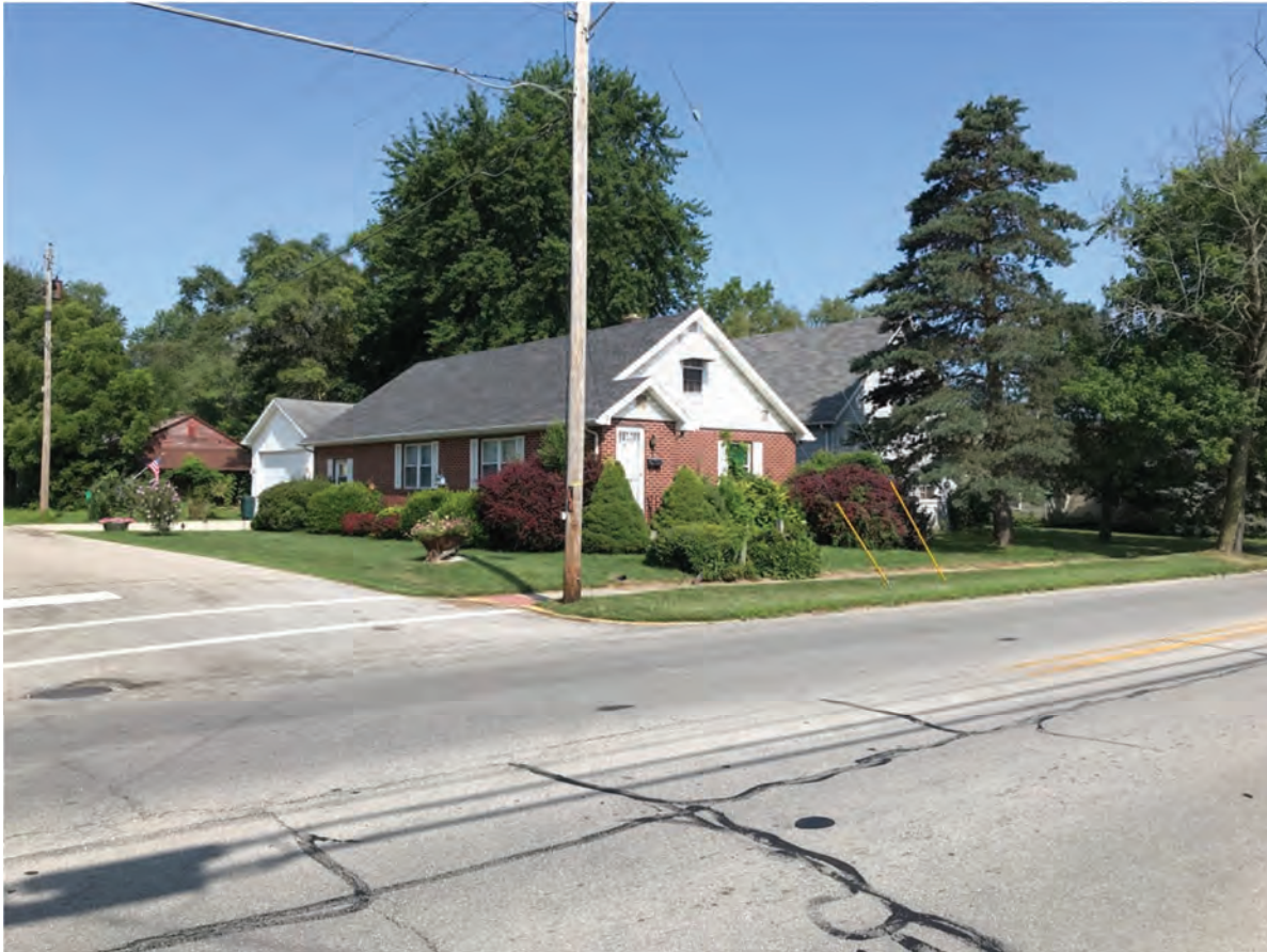
51. Looking NW at the intersection of US 27 (Meridian Street) and W. 9th Street
