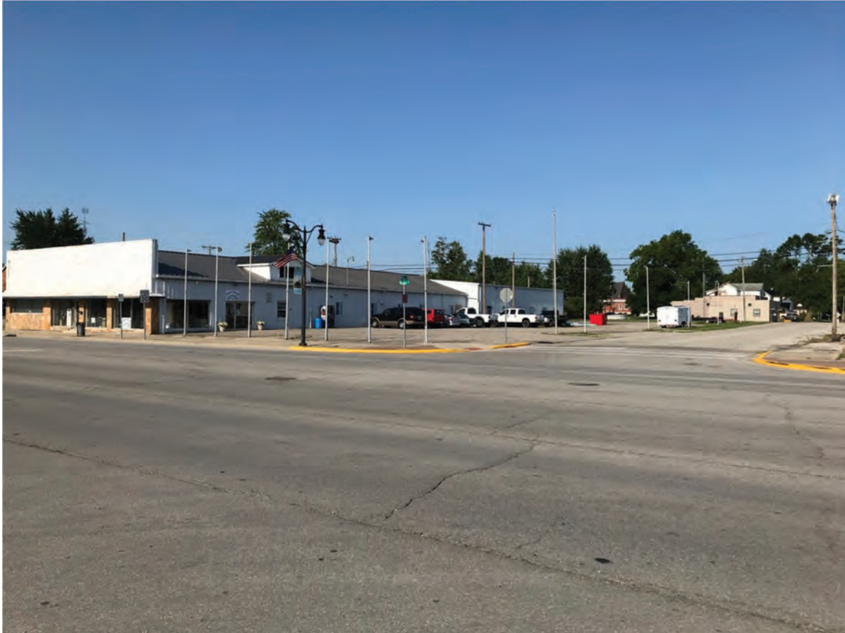
159. Looking SW at the intersection of US 27 (Meridian Street) and Race Street
