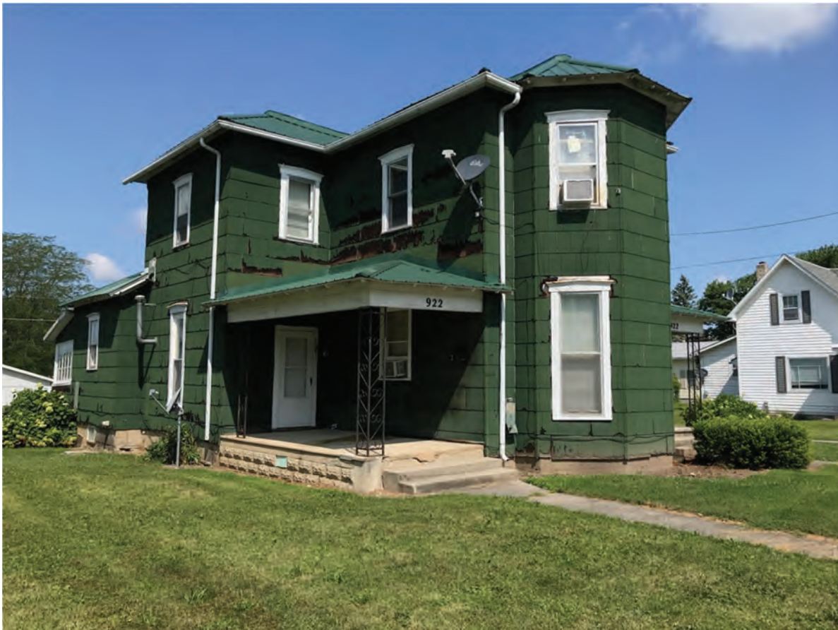
60. Looking NW at Lochmueller #27, Contributing, 922 S. Meridian Street
