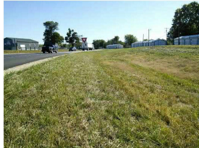
PP-2: Looking east at the southwest junction from SR 3 to SR 46 (2019-10-14)
