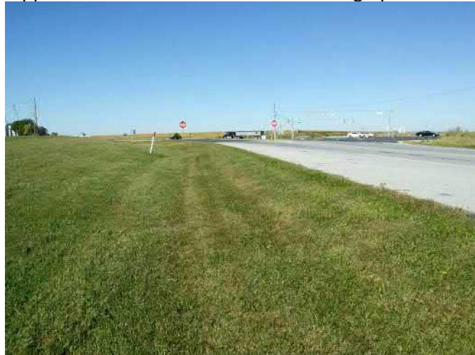
PP-1: Looking west from the southeast side of the project area along SR 46 (2019-10-14)
