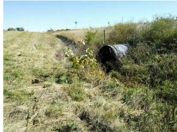
PP-11: Looking west at the culvert located east of Wetland A (2019-10-14)
