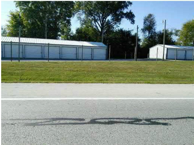
Photo Point 1: Looking south at storage business, from SR 46, south of the intersection
