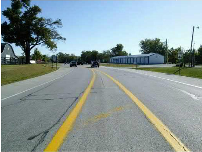
Photo Point 1: Looking east at SR 46 from south of the intersection
