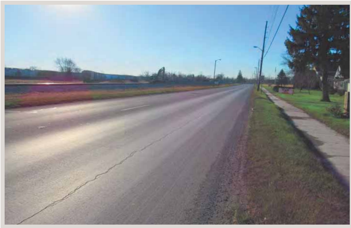
Photo 3: Looking south along US 31 from Maryland Street.
