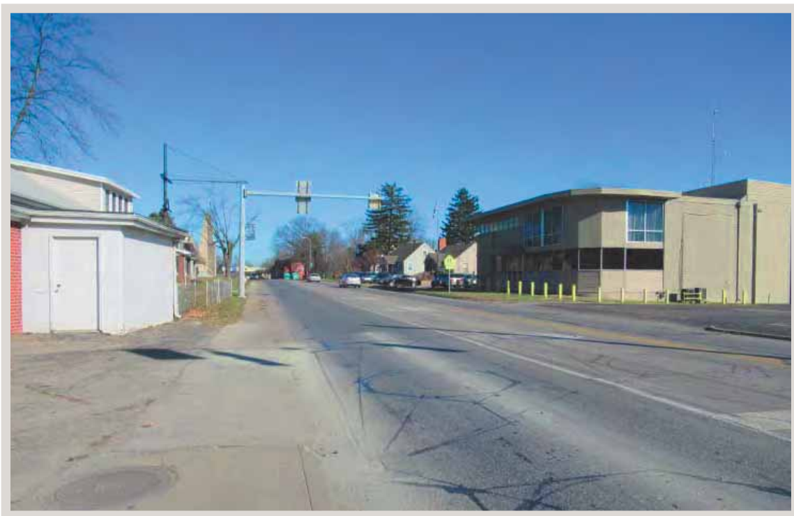
Photo 10: Looking northeast along US 31 from Utica Street.
