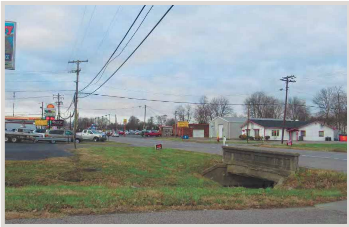
Photo 17: Looking northwest along US 31 from Foothill Drive, the southern project terminus.
