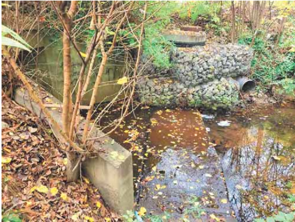
Photo 7: Investigation Area 1; looking north along the east side of US 31; culvert shown on the left carries US 31 over UNT to Silver Creek (downstream side pictured); no culvert work is proposed
