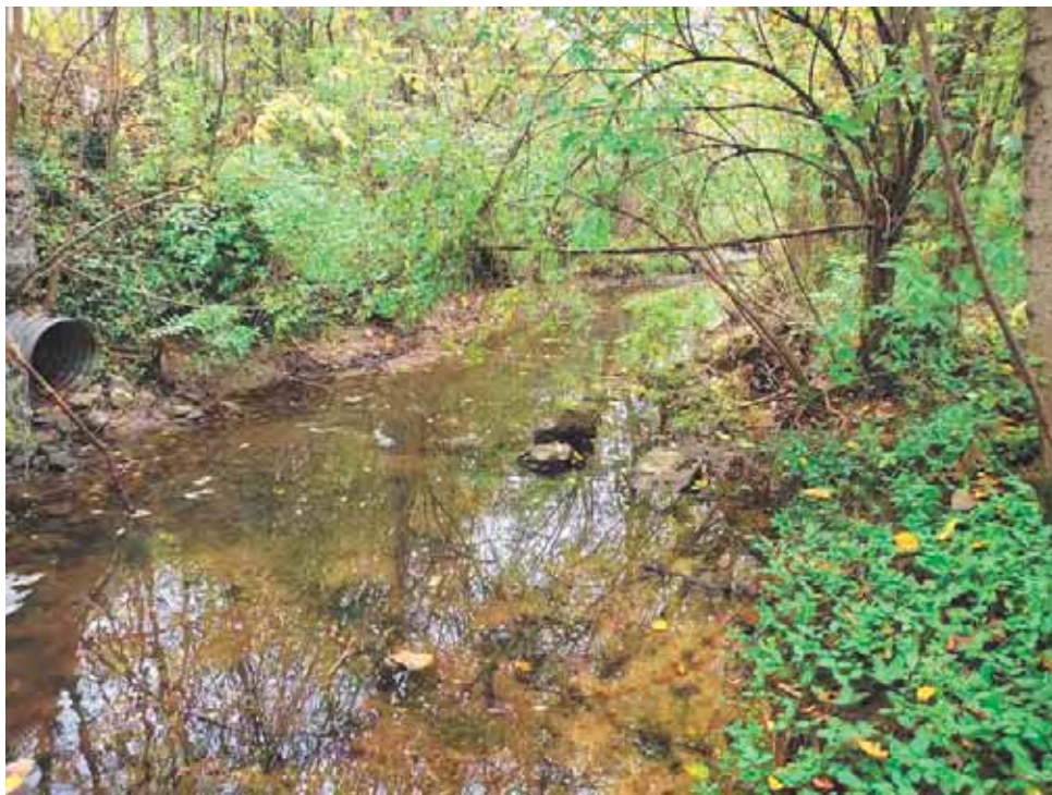
Photo 8: Investigation Area 1; looking east (downstream) along UNT to Silver Creek from the outlet of the US 31 culvert
