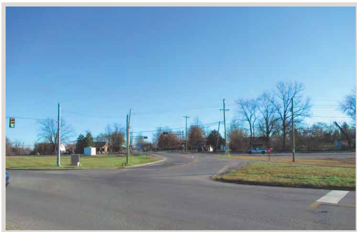
Photo 6: Looking northwest at CR 403 from the west side of US 31.
