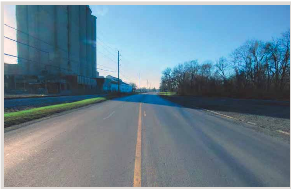
Photo 2: Looking south along US 31 from the northern project terminus. The Louisville Cement Company is at left.
