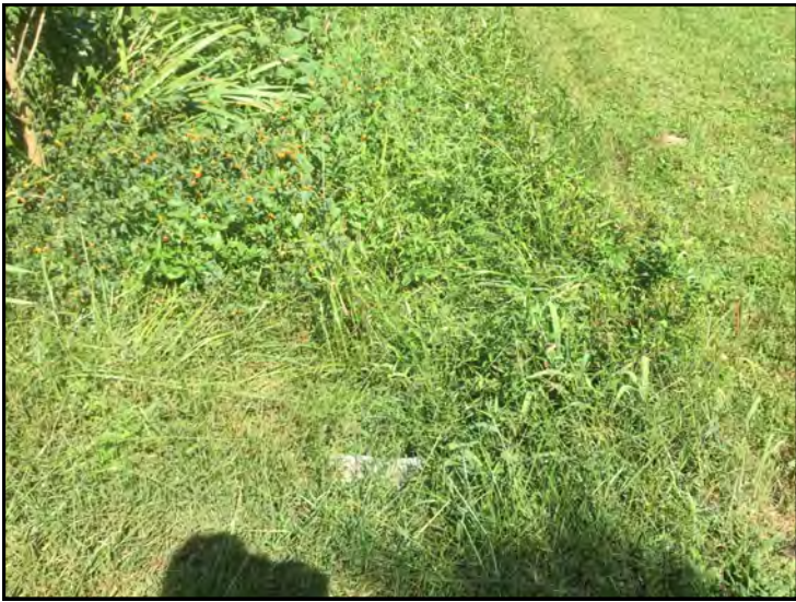
29. View of UNT 2 and Culvert 1 - inlet, looking northeast (upstream).
