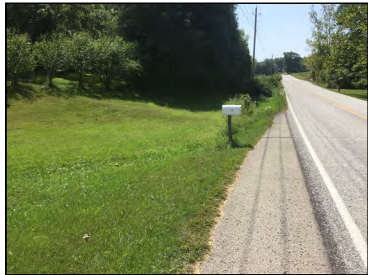
20. View of S.R. 58 ROW from the PSL, looking southwest.
