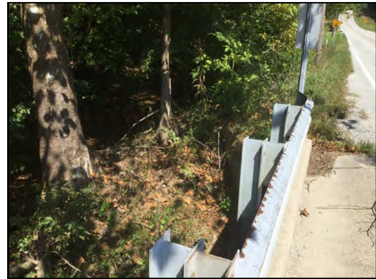
10. View of S.R. 58 ROW and south bank of UNT 1, looking northeast.
