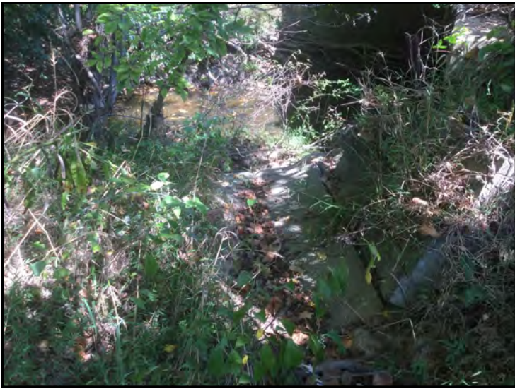
5. View of RSD 1, looking northeast.
