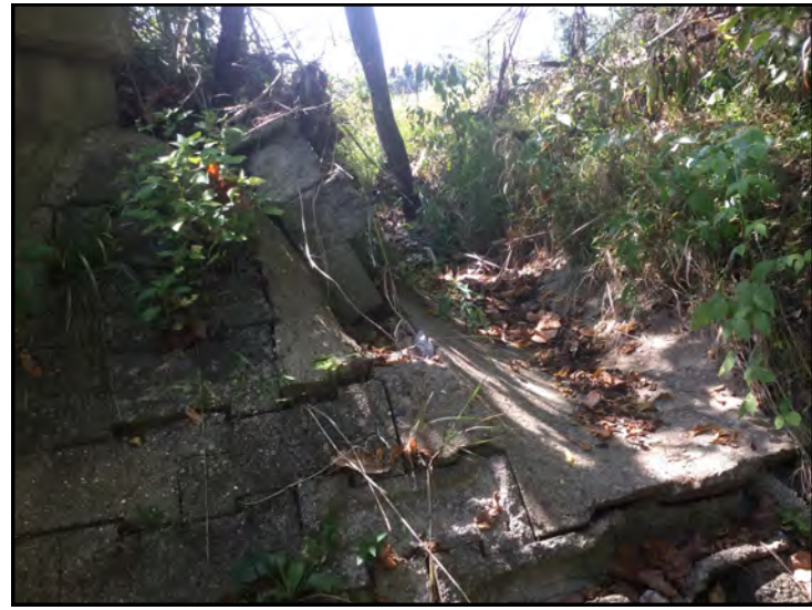
6. View of RSD 1, looking southwest.
