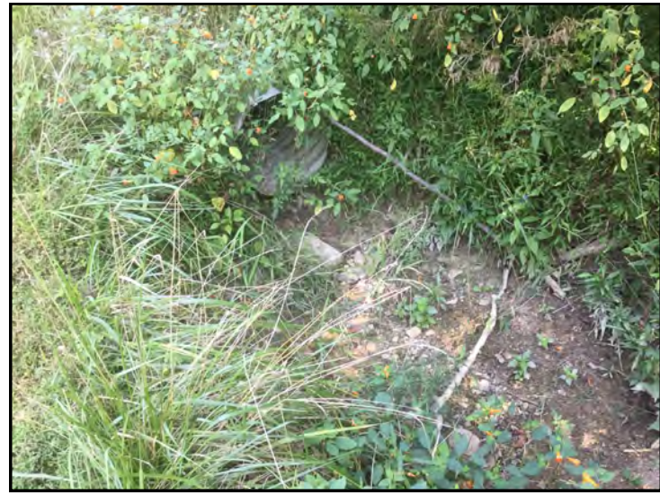
30. View of UNT 2 and Culvert 1 - outlet, looking east.
