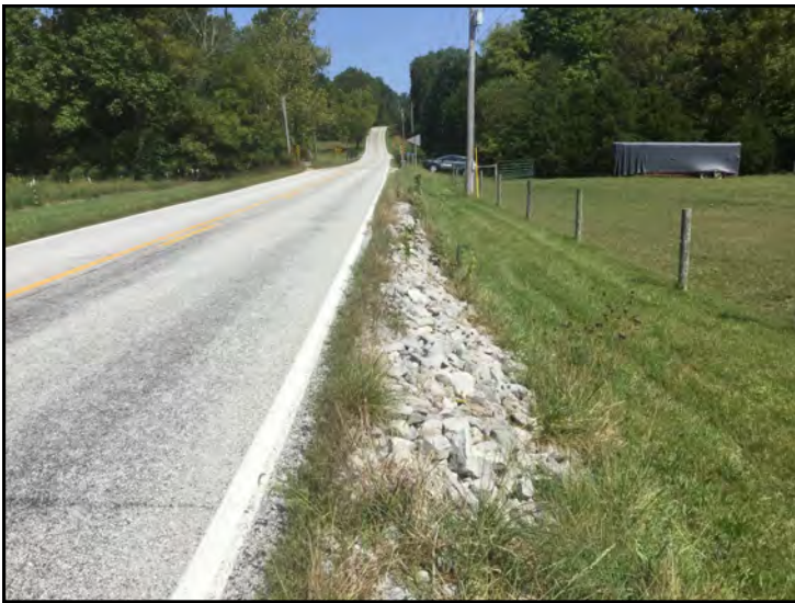
1. View of S.R. 58 Right-of-Way (ROW) from the project study limits (PSL), looking northeast.
