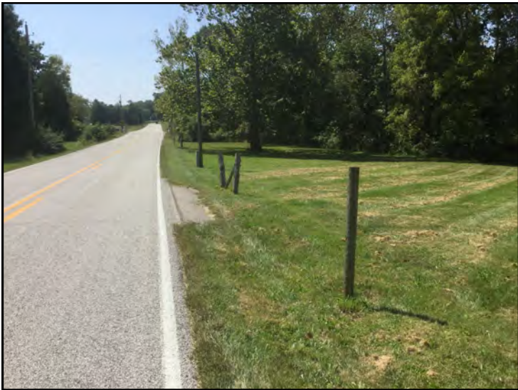
19. View of S.R. 58 ROW from the PSL, looking southwest.
