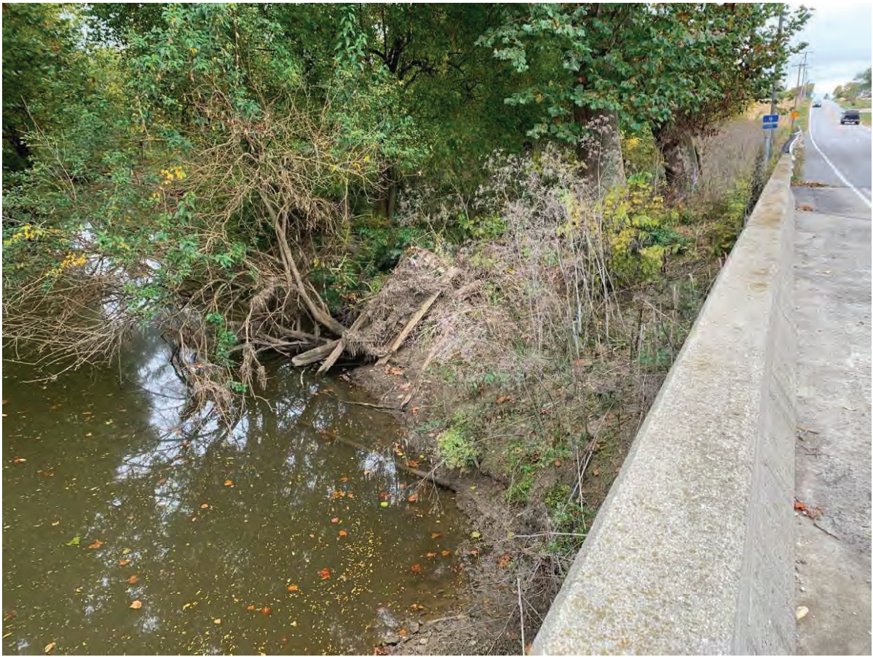
15. Looking at southwest quadrant from bridge
