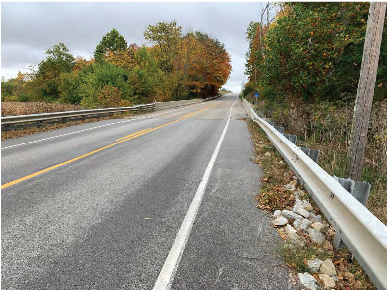
12. Looking east along SR 244
