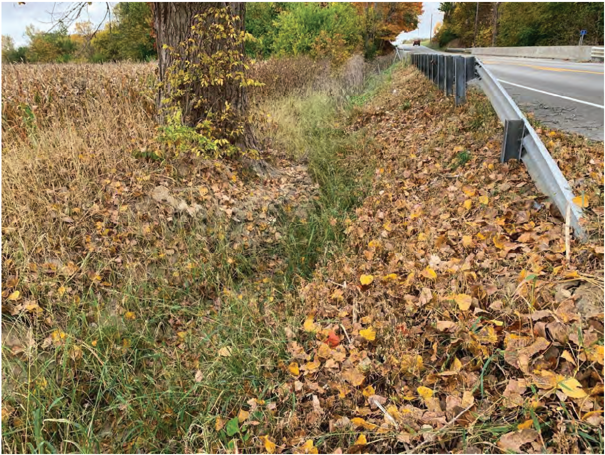
13. Looking east along roadside ditch
