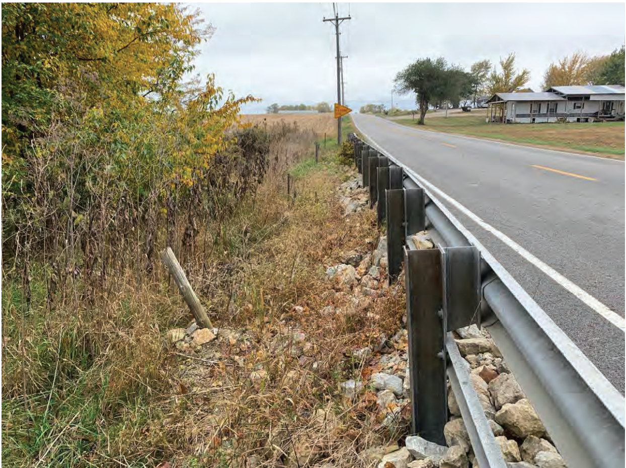
10. Looking west along roadside
