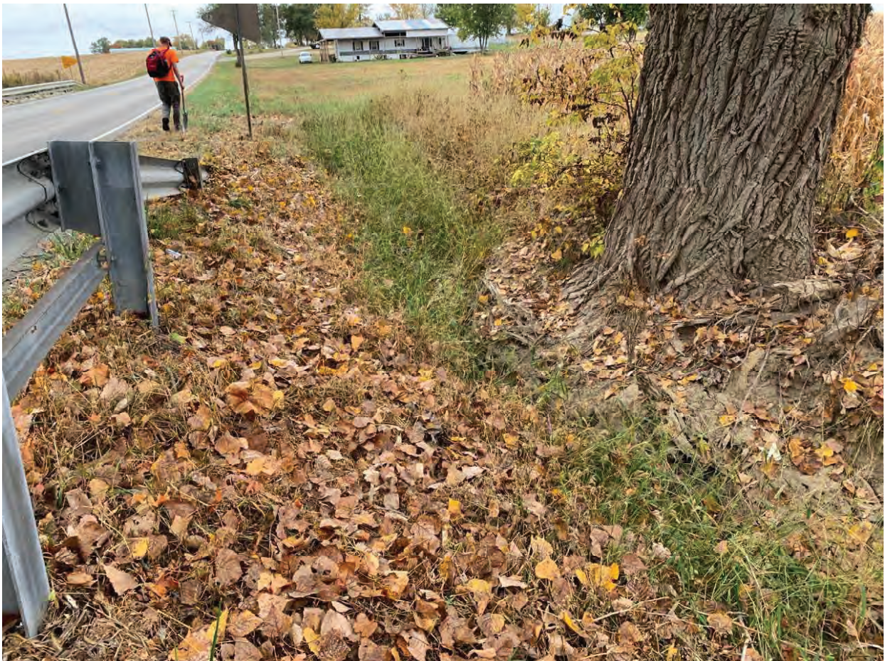
14. Looking west along roadside ditch
