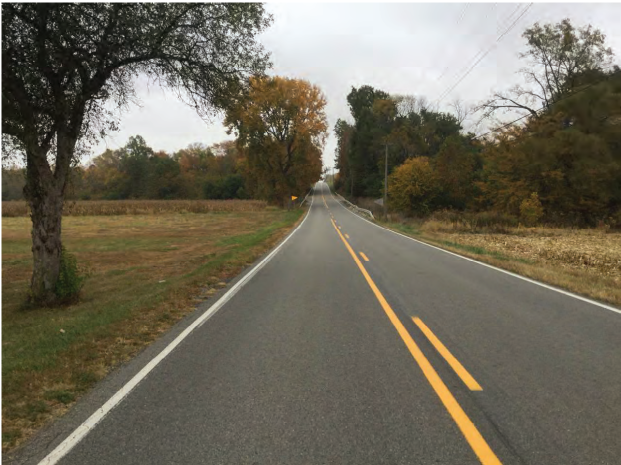
2. Looking east along SR 244
