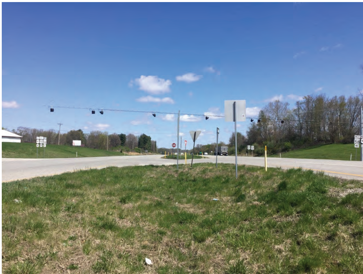
48. Looking north within US 41 median toward US 41 & SR 58 intersection
