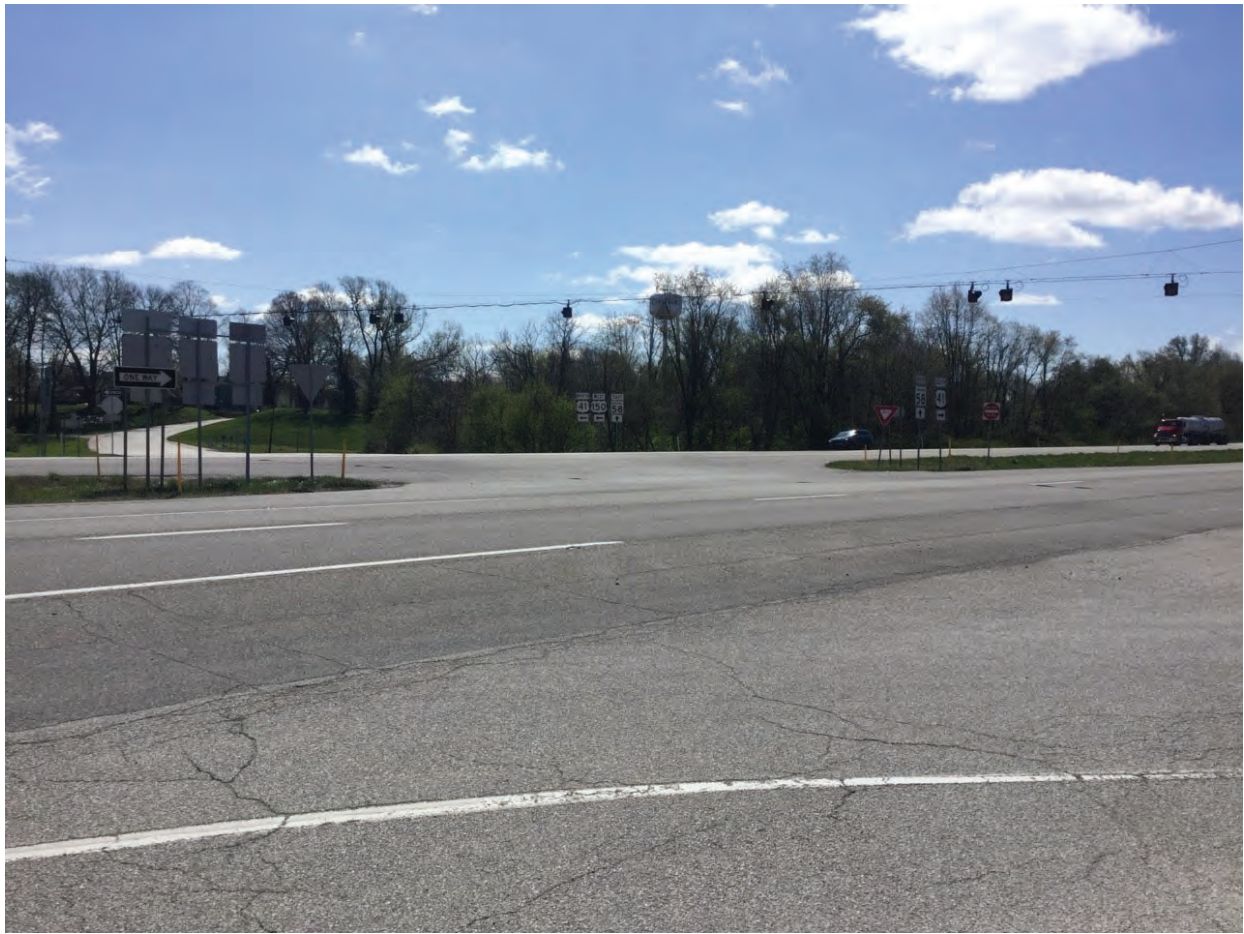
51. Looking south east at US 41 & SR 58 interchange
