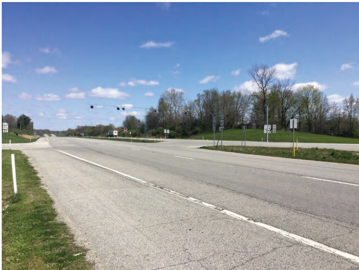
46. Looking north east at US 41 & SR 58 intersection
