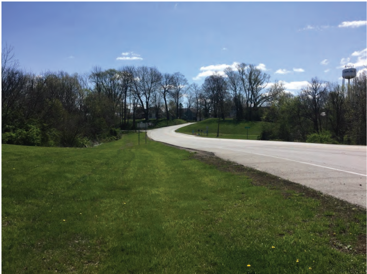
64. Looking east along SR 58
