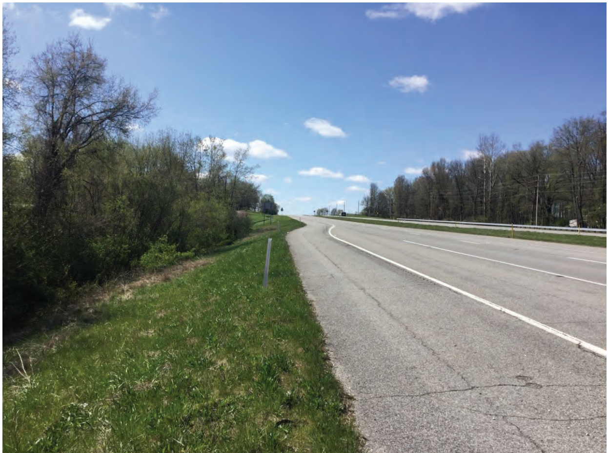
14. Looking south along US 41
