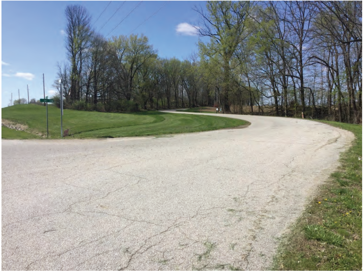
39. Looking south west along S Ledgerwood Street
