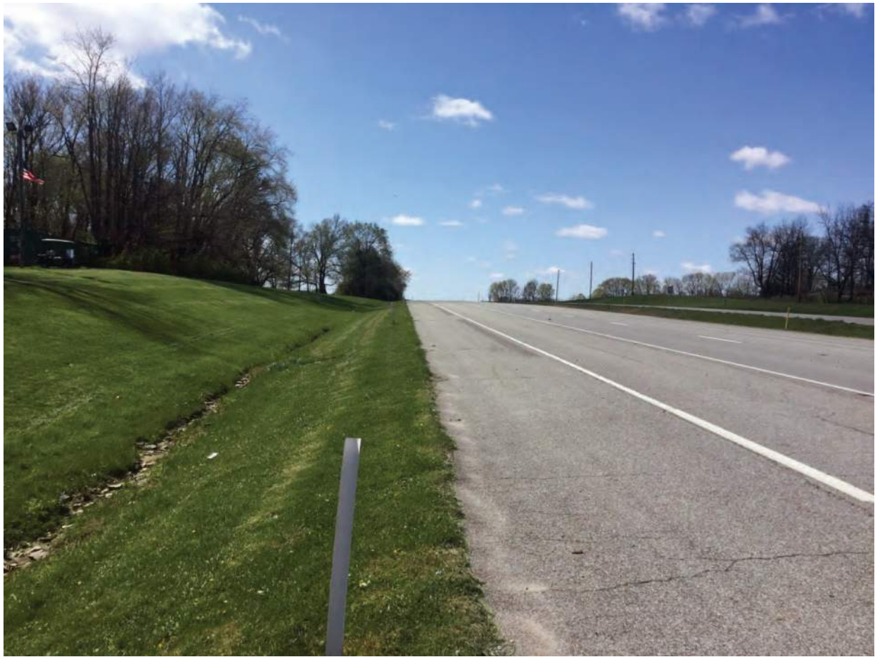
23. Looking south along US 41 at RSD3
