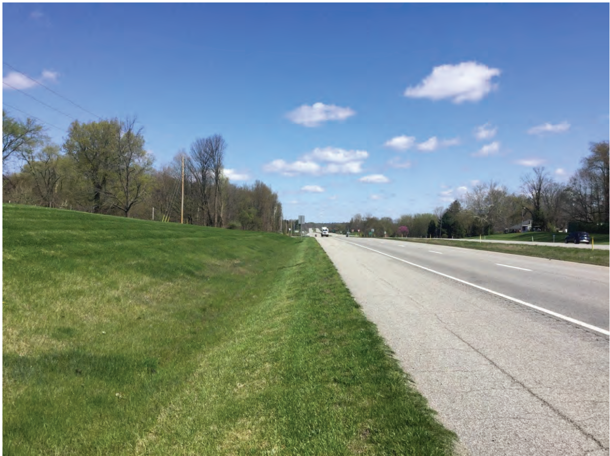
32. Looking north along US 41
