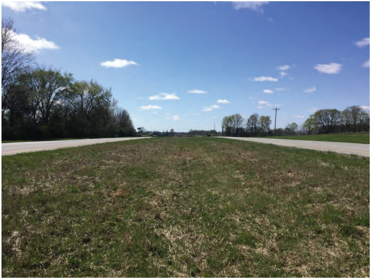
29. Looking south within US 41 median
