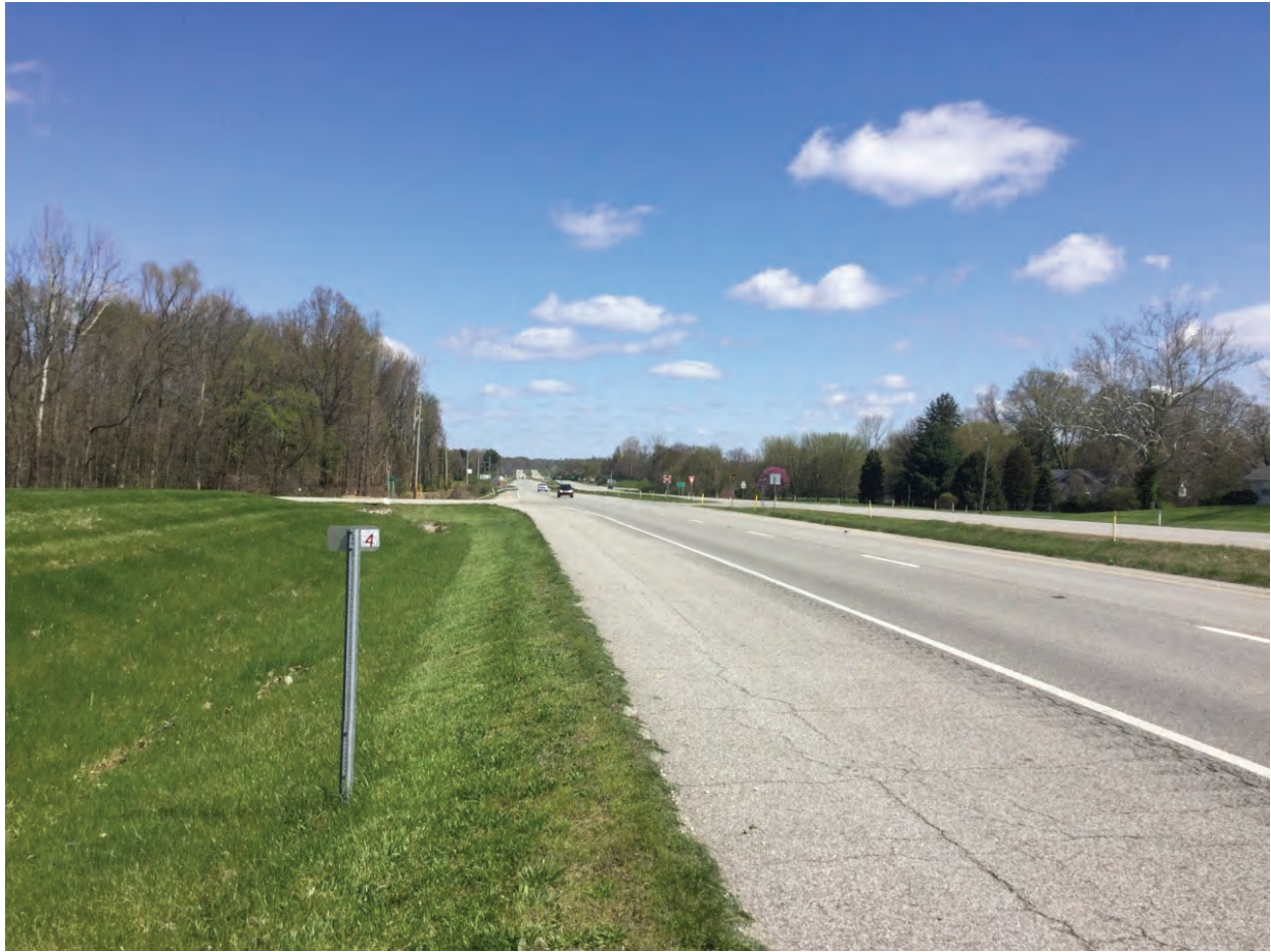
33. Looking north along US 41
