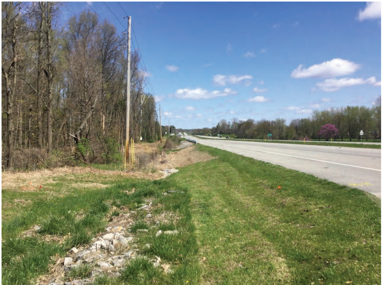
38. Looking north along US 41
