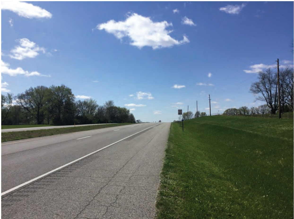
34. Looking south along US 41
