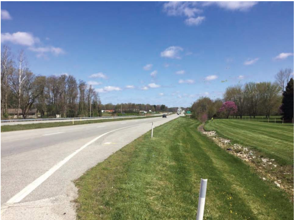
20. Looking north along US 41
