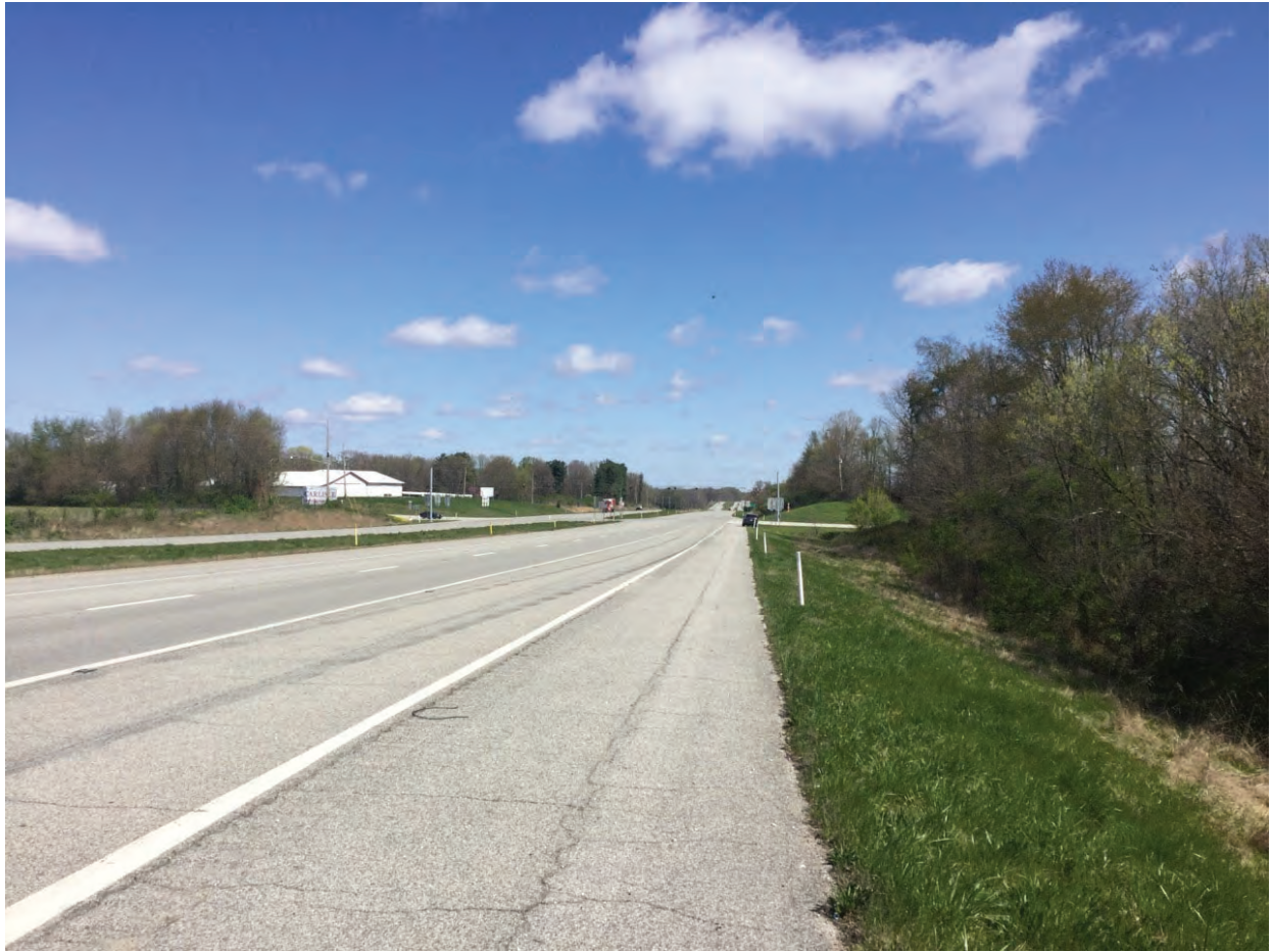
17. Looking north along US 41
