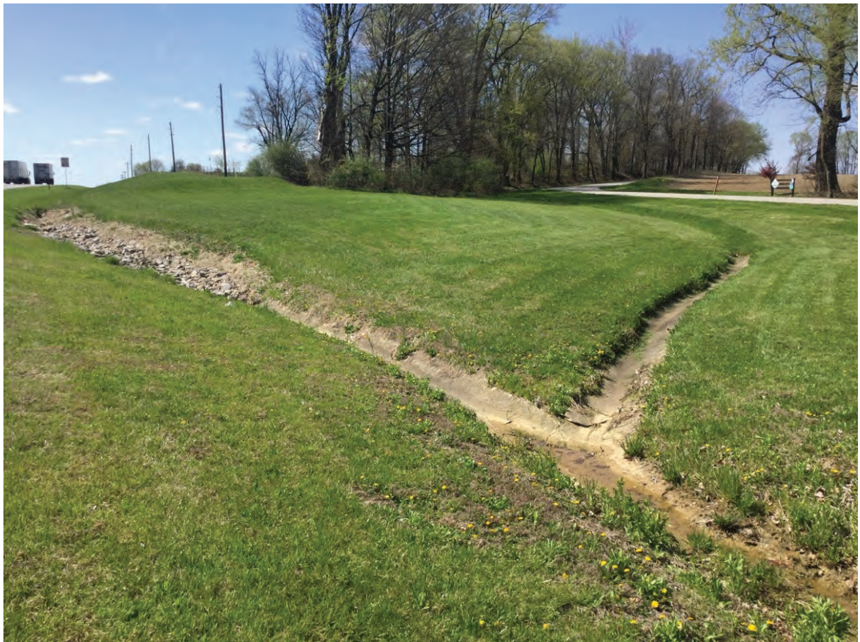
36. Looking south west at RSD 1 and RSD 2
