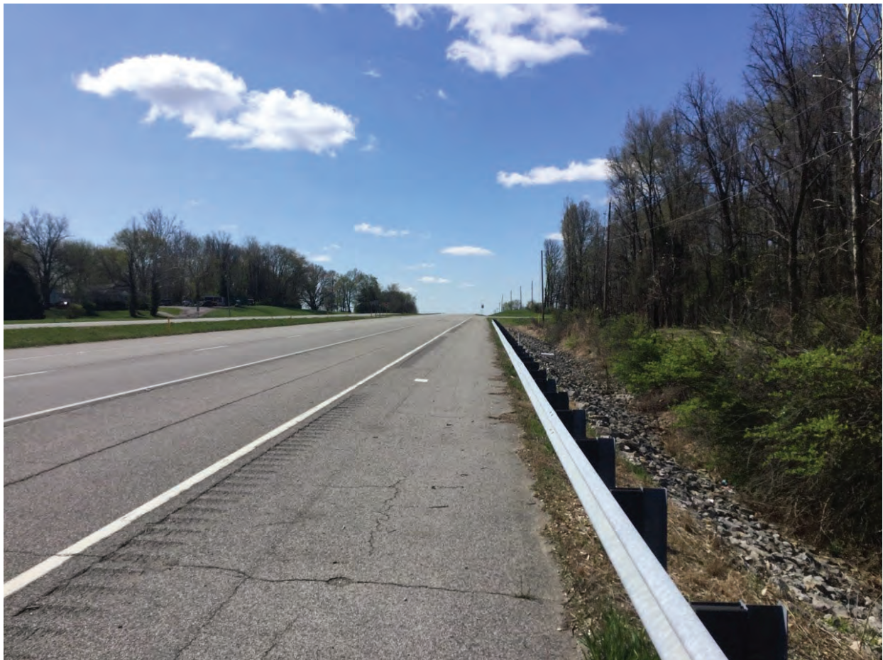
42. Looking south along US 41
