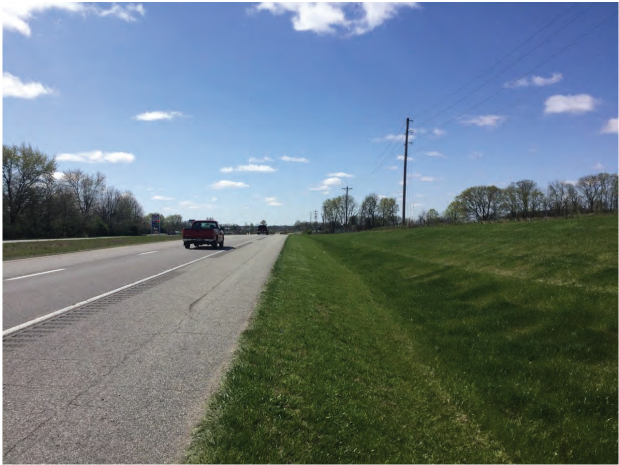
31. Looking south along US 41
