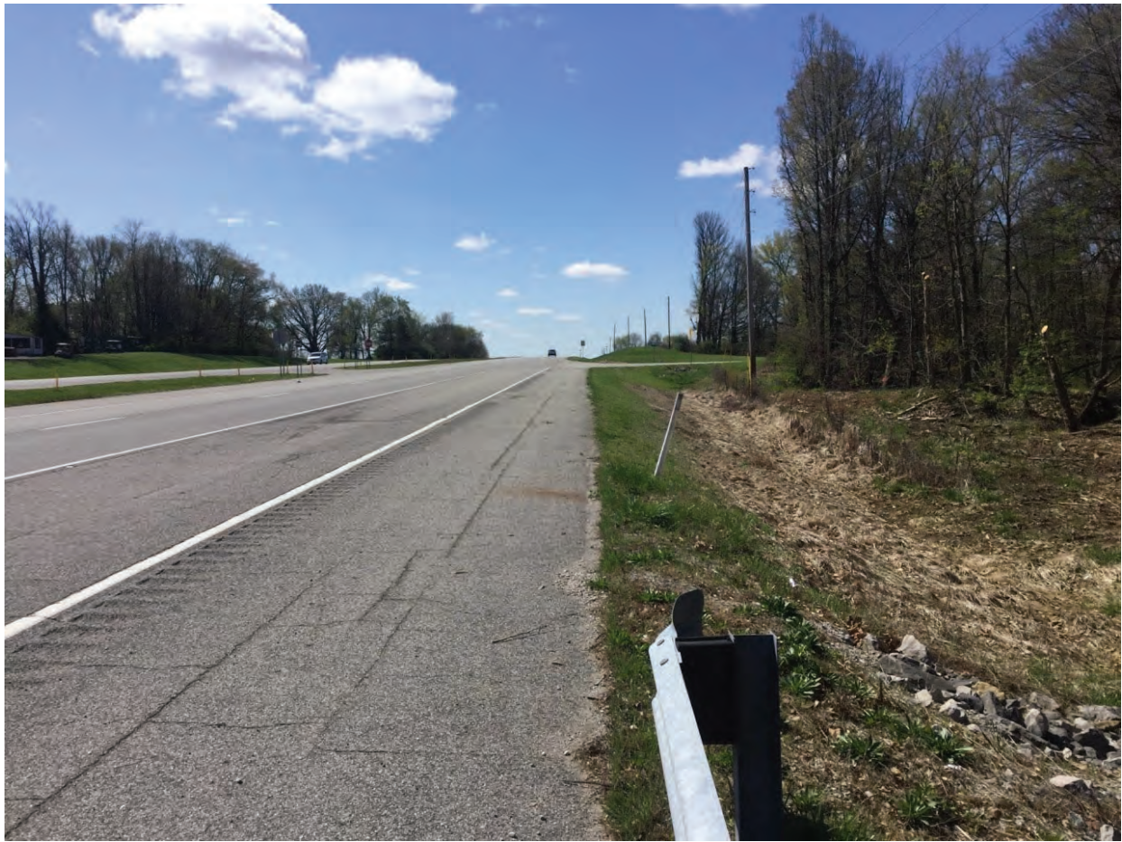
41. Looking south along US 41
