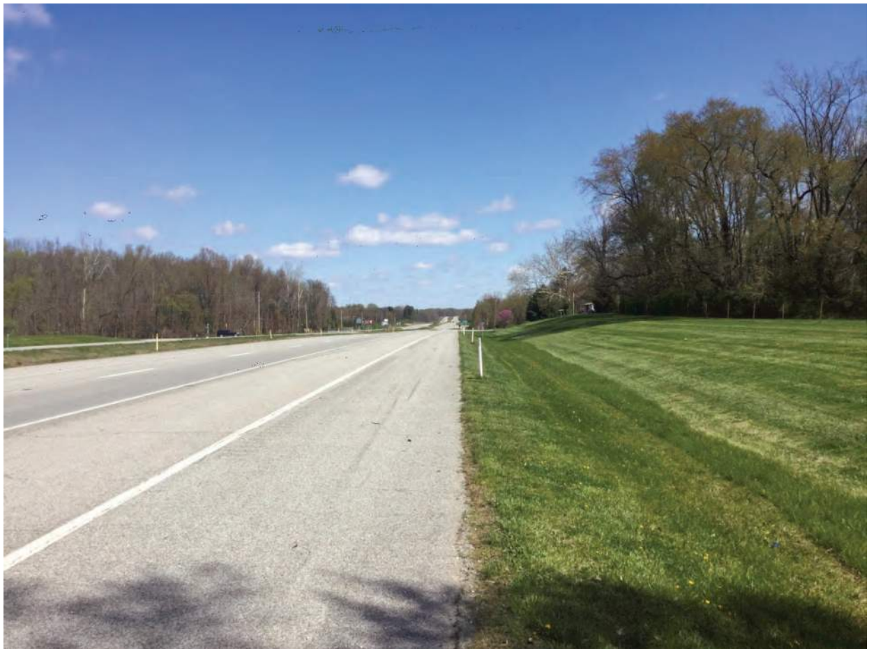
26. Looking north along US 41
