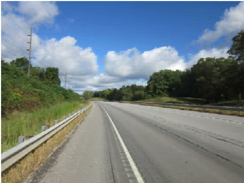
12. Looking north along US 231
