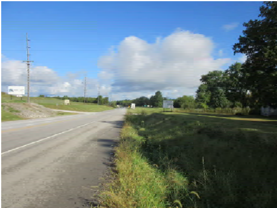
8. Facing northwest along US 231 towards CR 800 S
