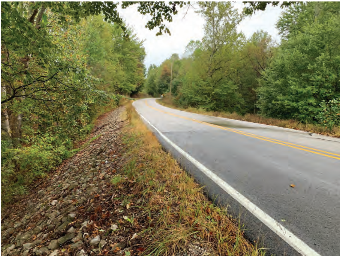
8. Slide correction area, north side of SR 62 facing east
