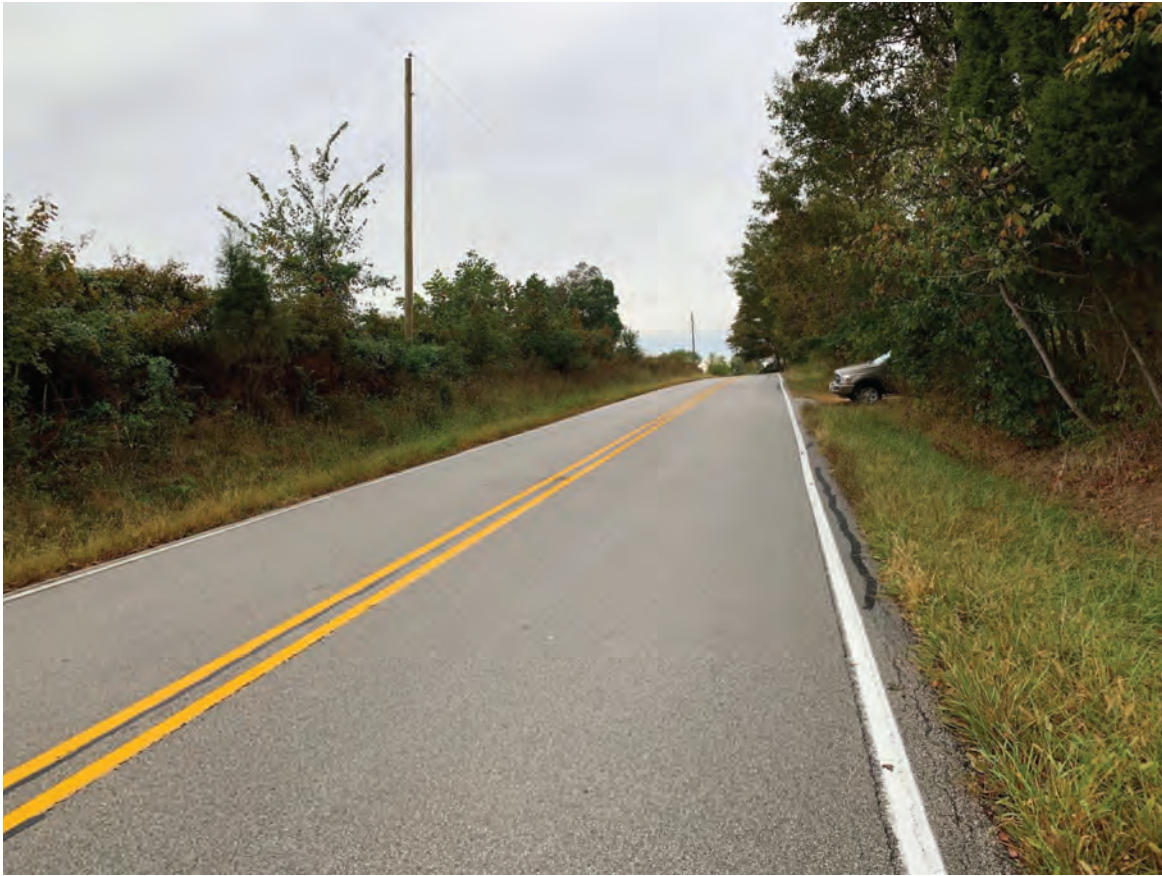
3. SR 62 facing east from west survey boundary
