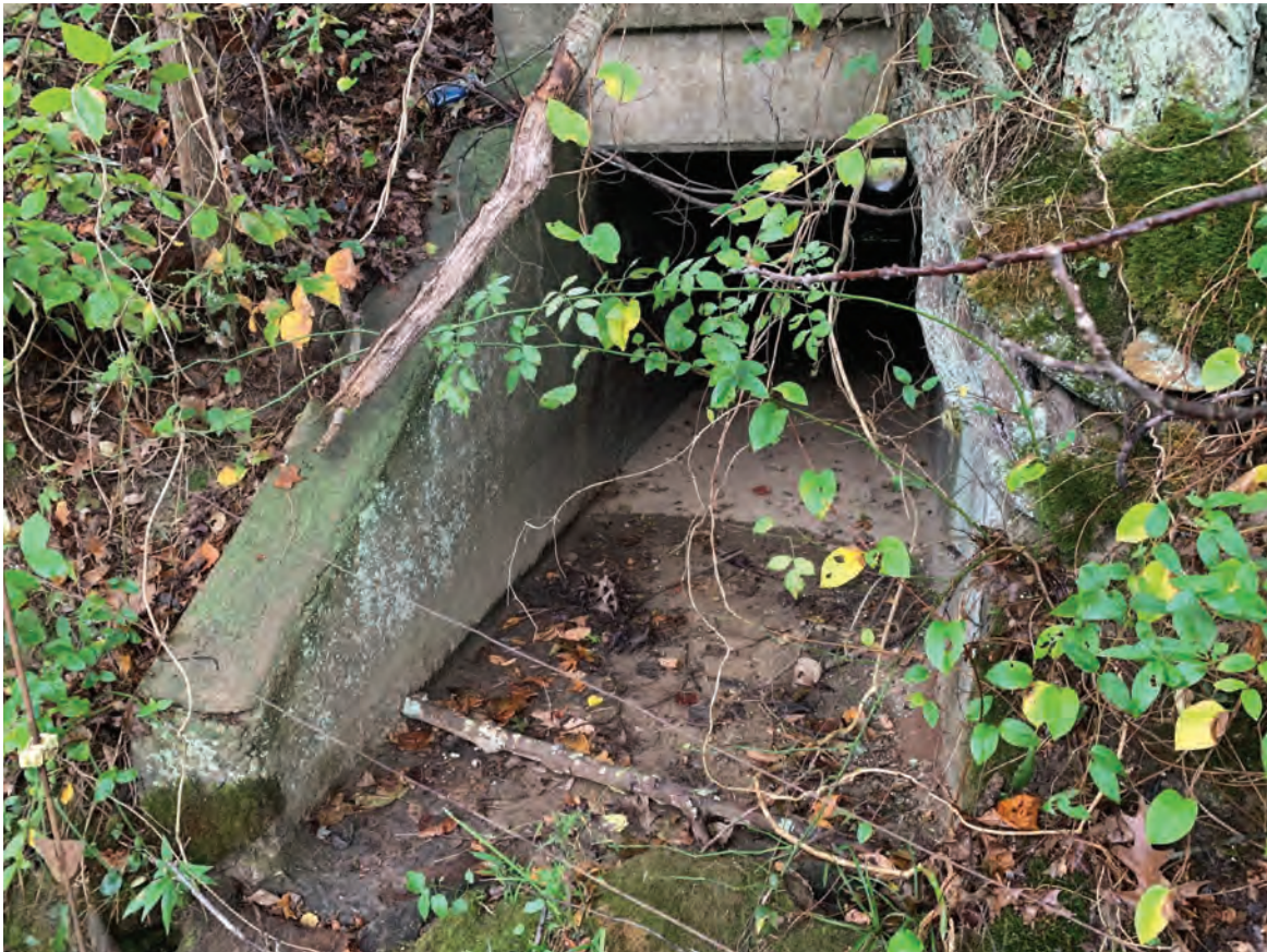
4. Culvert outlet under SR 62 facing south
