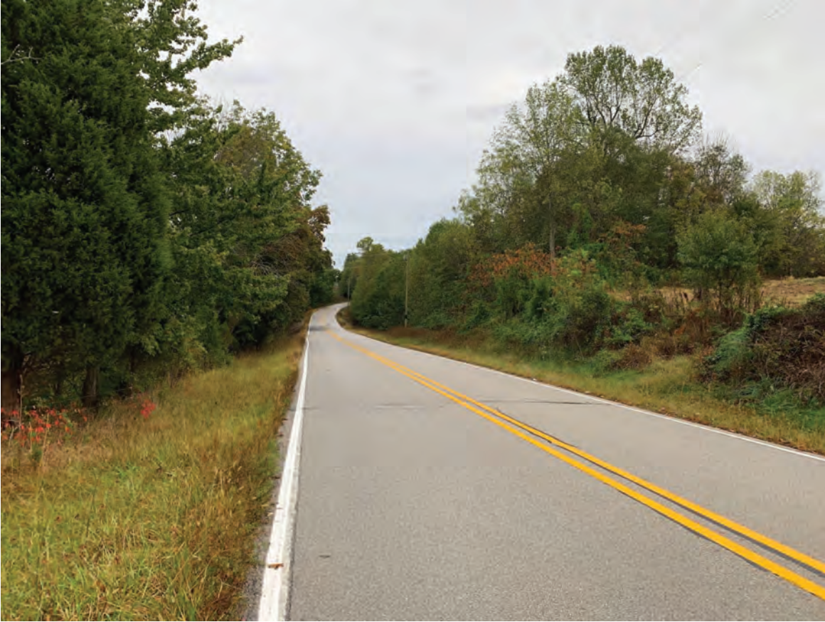
1. North side of SR 62 facing east from west survey boundary
