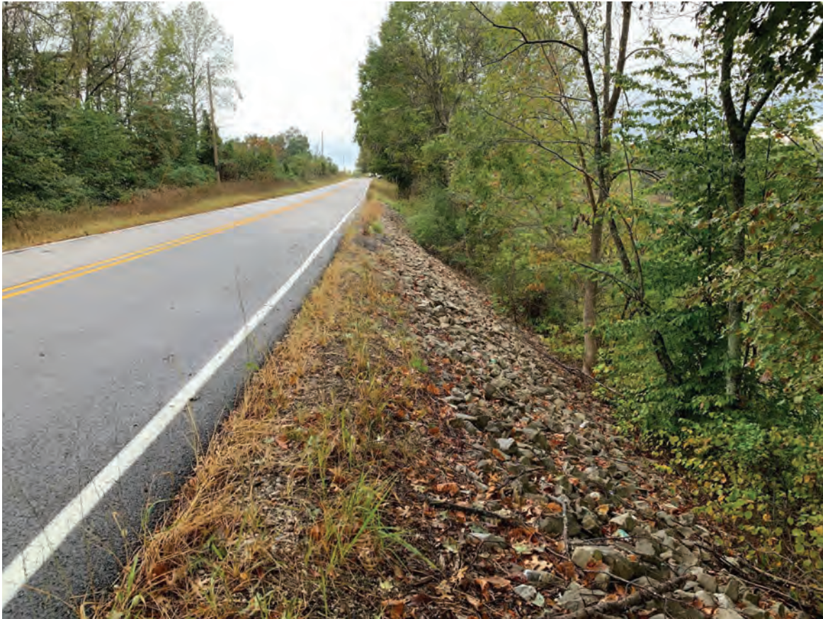
7. North side of SR 62 facing west
