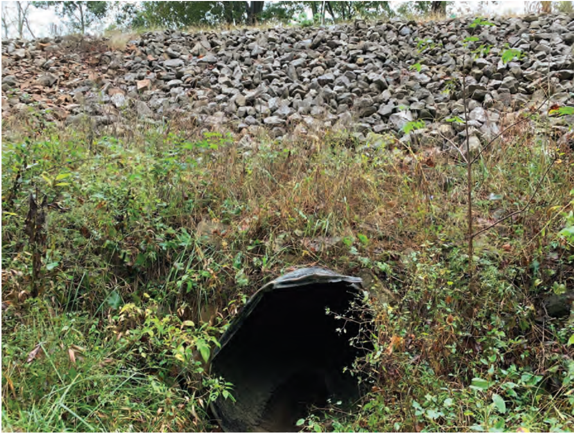
5. Culvert inlet under SR 62 facing north
