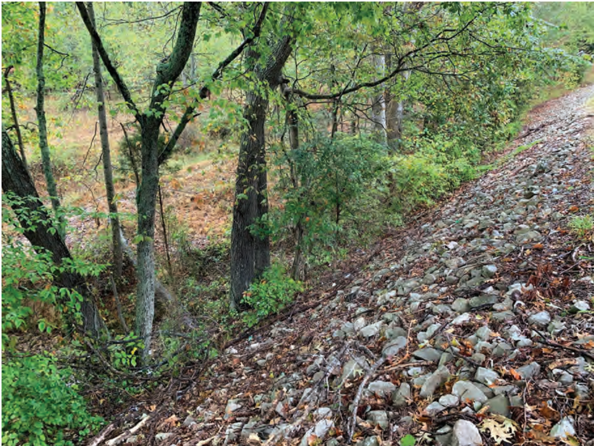
6. North side of SR 62 embankment facing northeast
