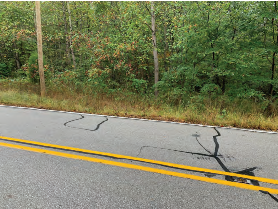
12. View of south side of SR 62 facing south
