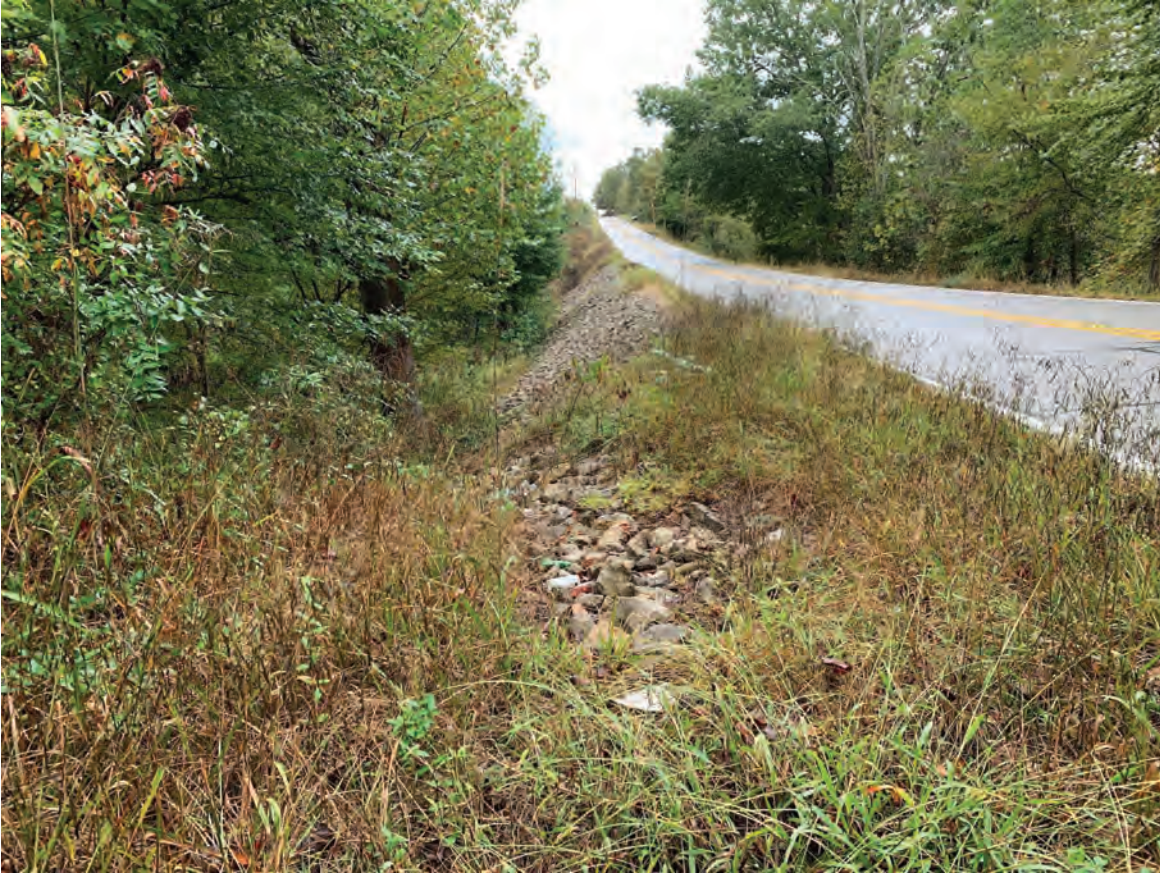
11. South side of SR 62 facing west
