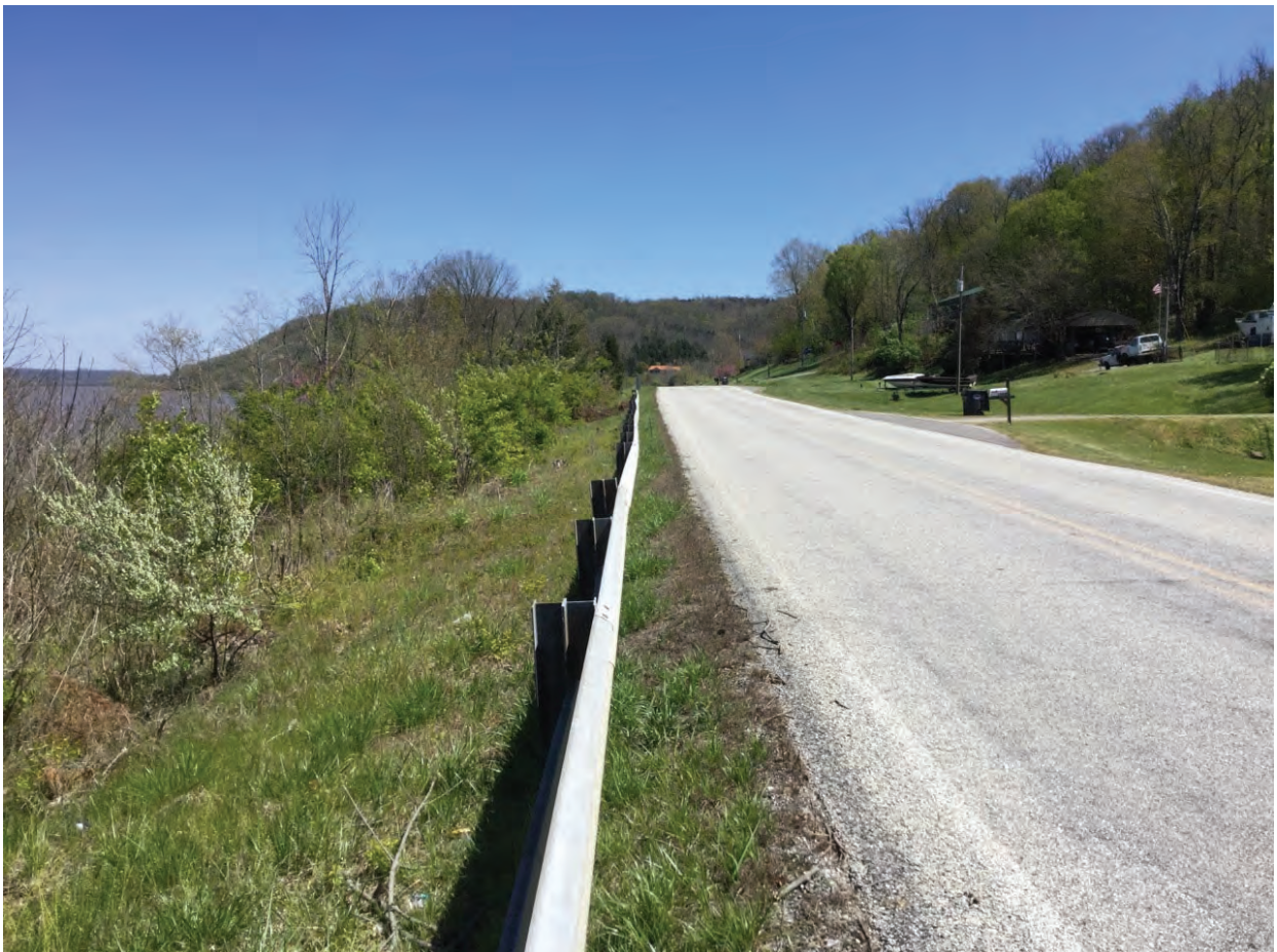
16. Looking southeast along State Road 156 – 4/22/2020
