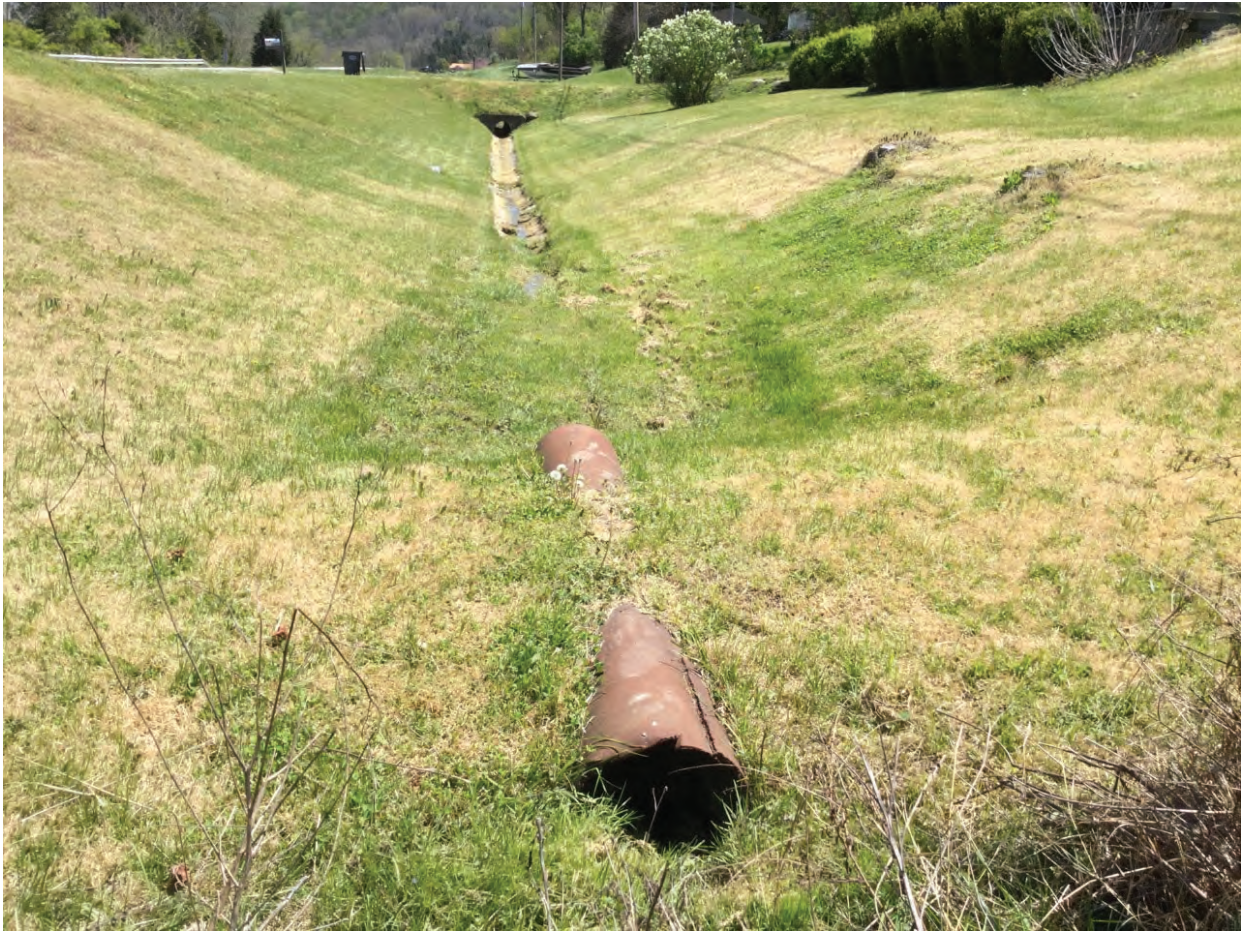
7. Looking southeast at metal pipe culverts and concrete lined drainage area – 4/21/2020
