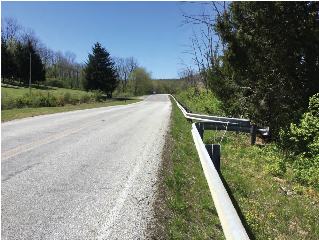
17. Looking northwest along State Road 156 – 4/21/2020
