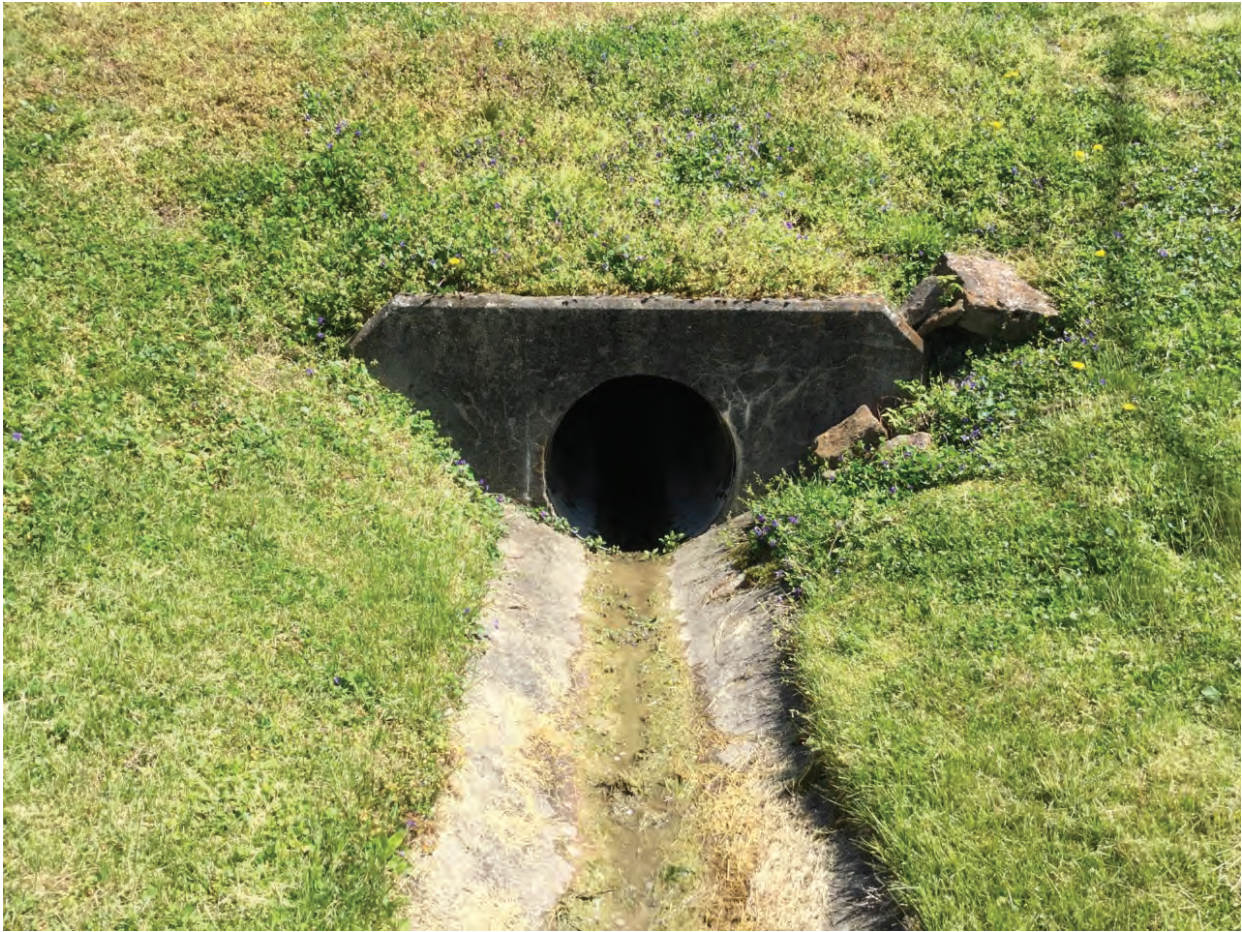
9. Looking southeast at culvert below residential driveway – 4/21/2020
