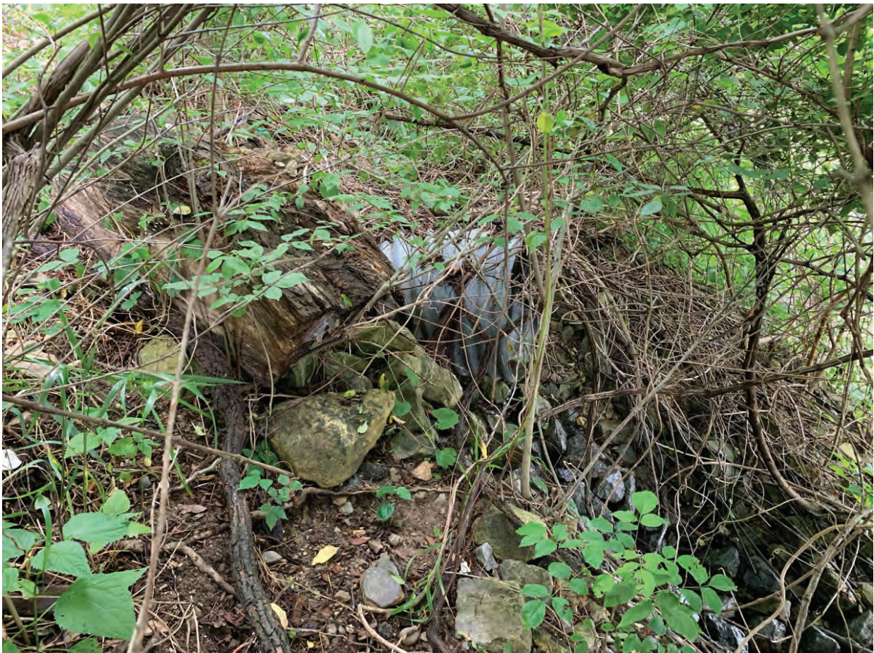
18. Looking northwest at culvert below State Road 156 – 6/22/2020
