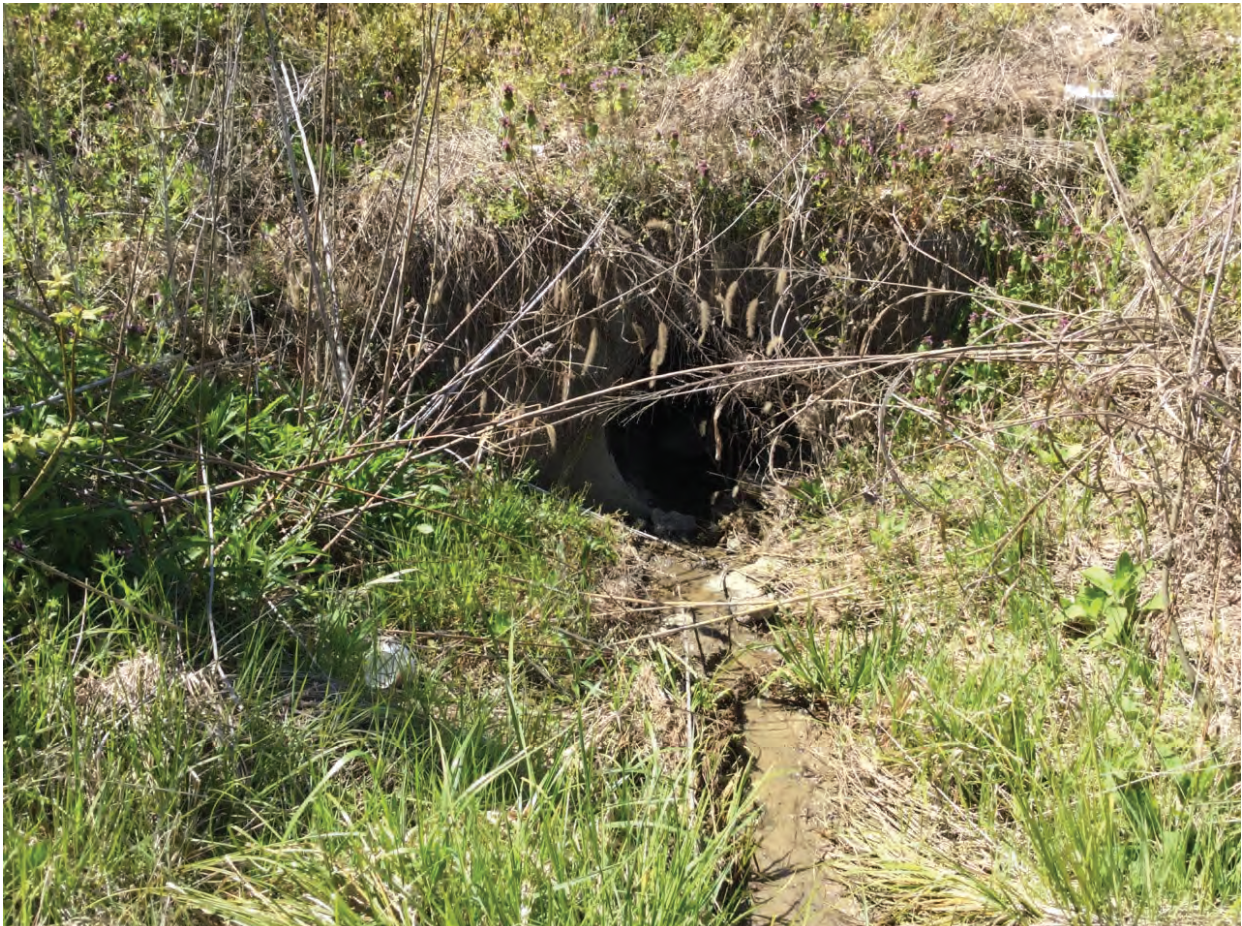
10. Looking southeast at culvert below residential driveway – 4/21/2020
