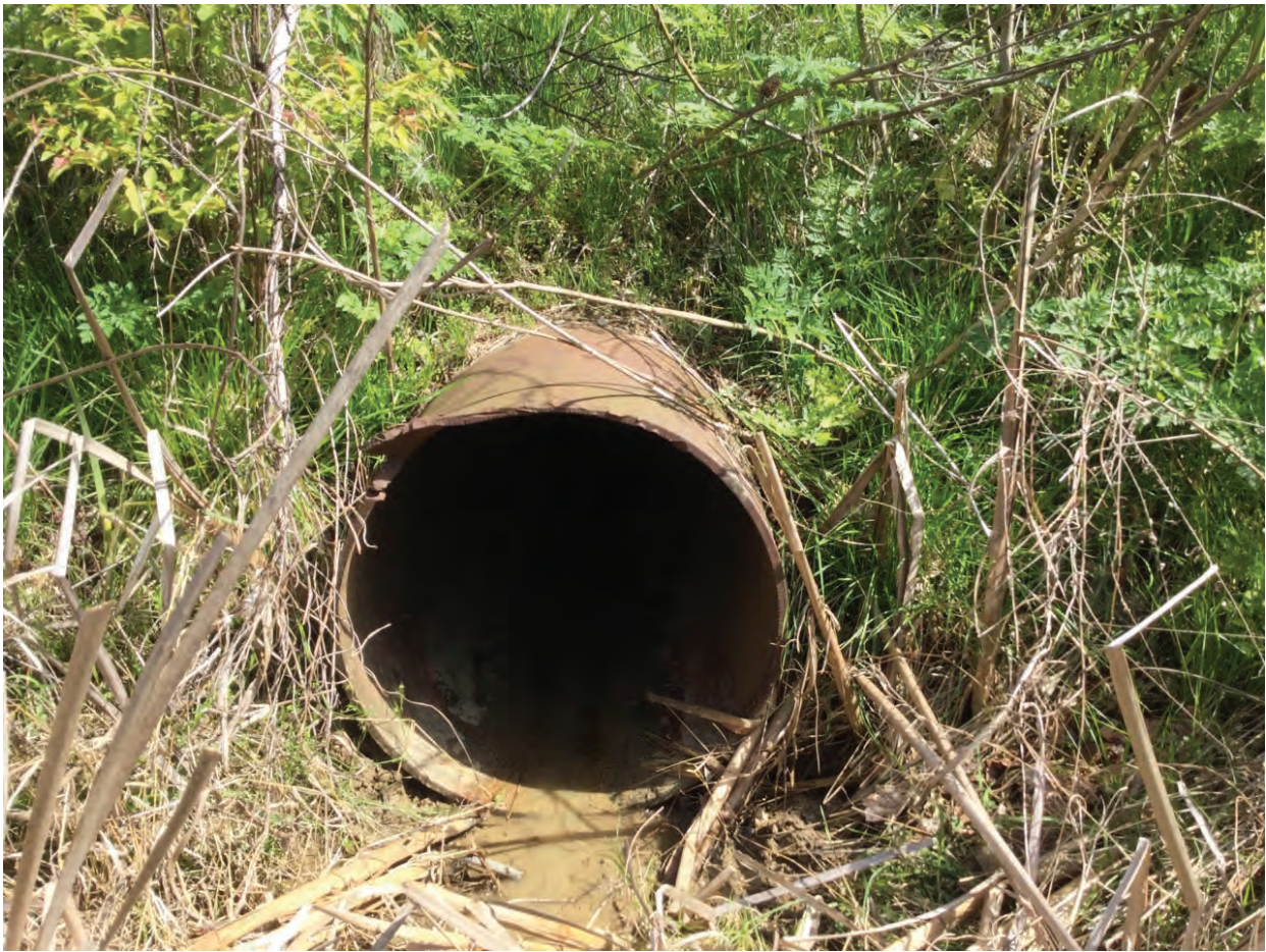
3. Looking northeast at culvert below State Road 156 – 4/21/2020
