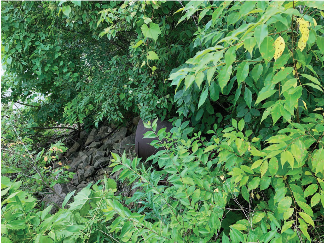
15. Looking northeast at culvert outlet below State Road 156 – 6/22/2020
