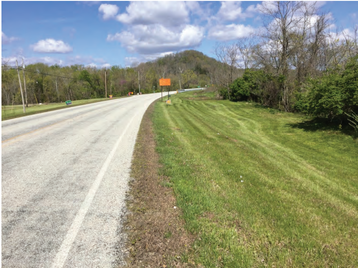
2. Looking northwest along State Road 156 – 4/21/2020
