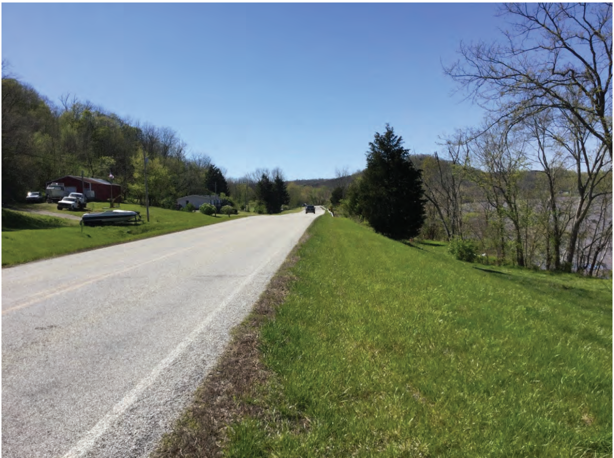
14. Looking northwest along State Road 156 – 4/21/2020
