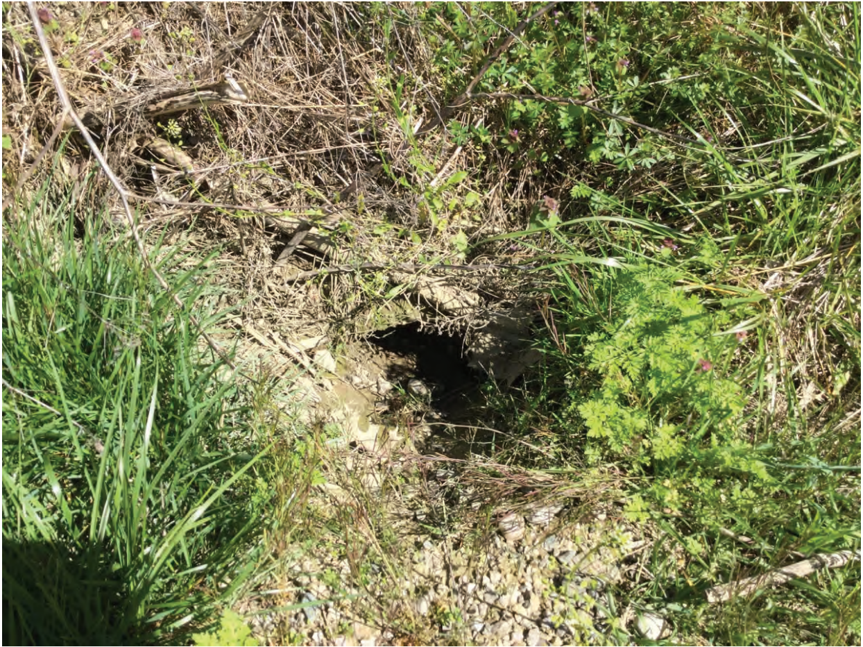
13. Looking southeast at culvert below residential driveway – 4/21/2020
