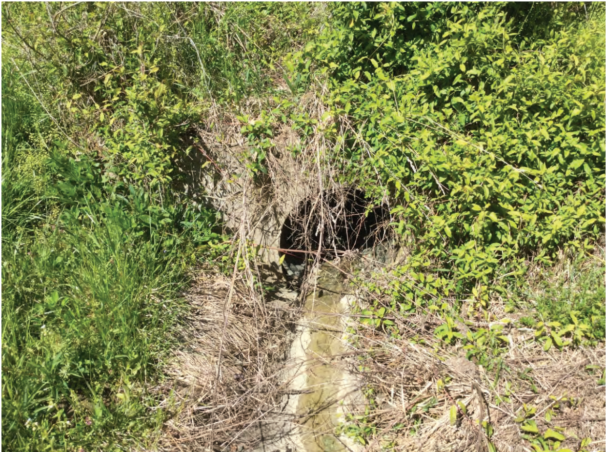
12. Looking northeast at culvert below State Road 156 – 4/21/2020
