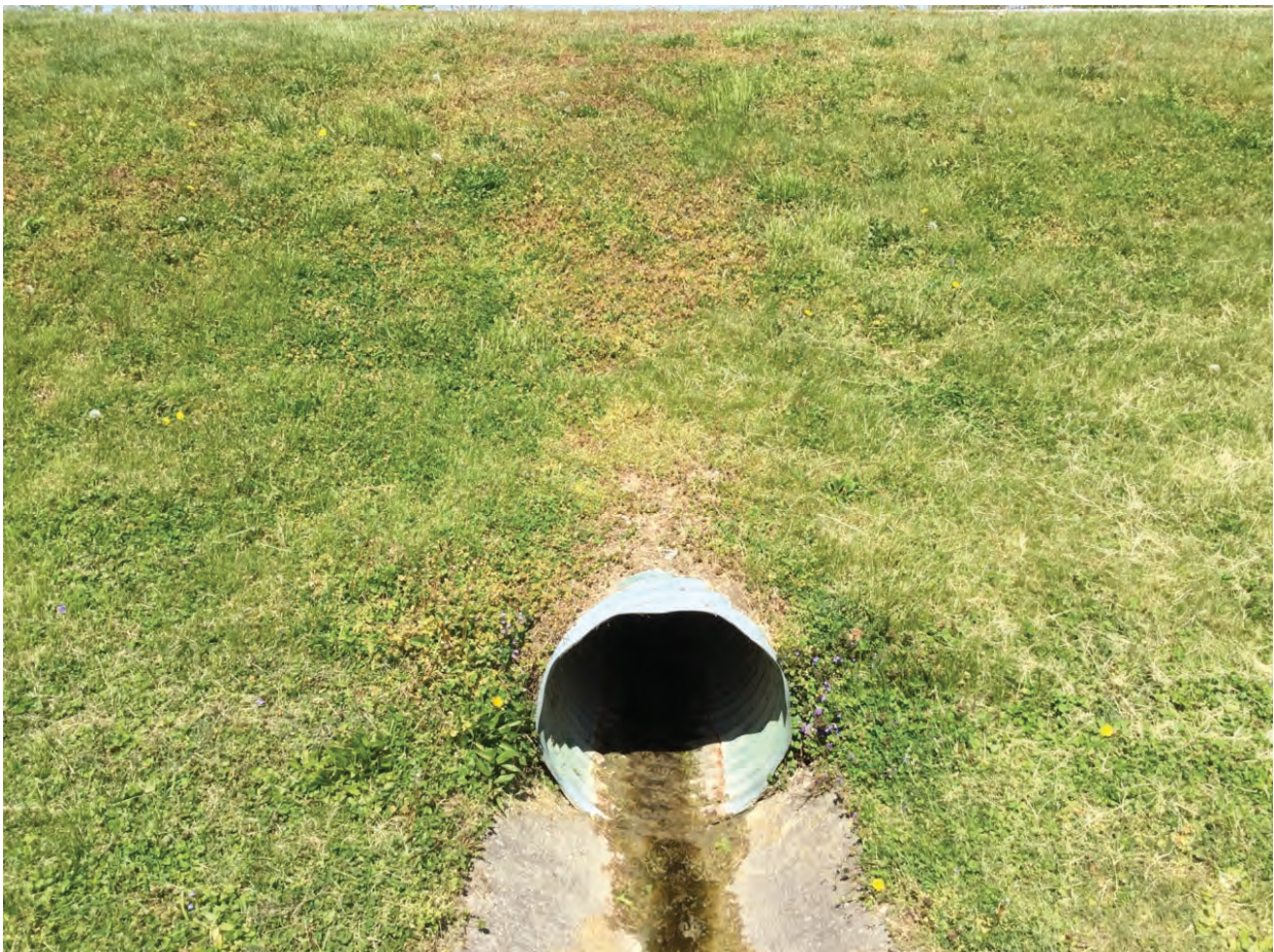
8. Looking northeast at culvert below State Road 156 – 4/21/2020
