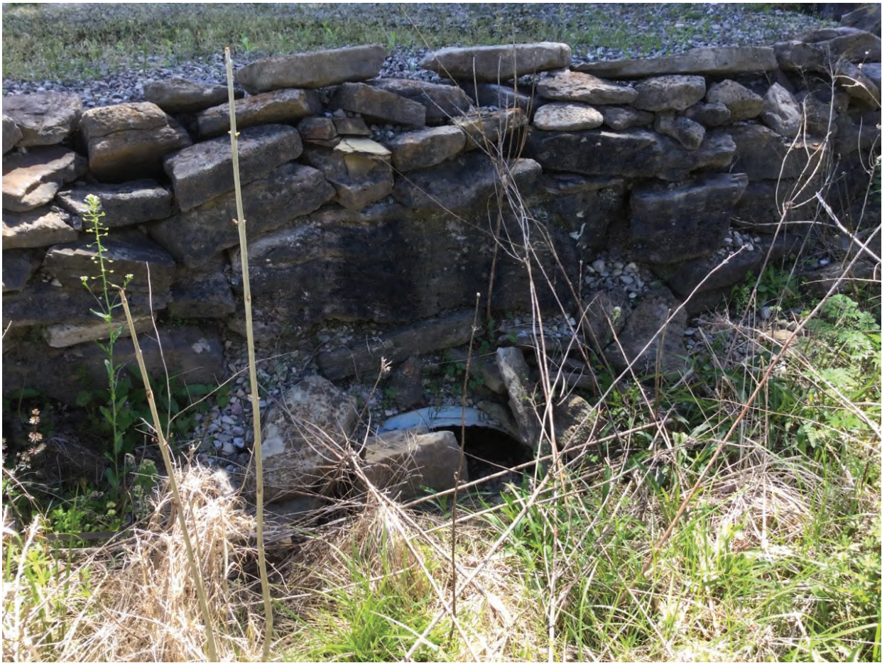
5. Looking south at culvert below residential drive – 4/21/2020
