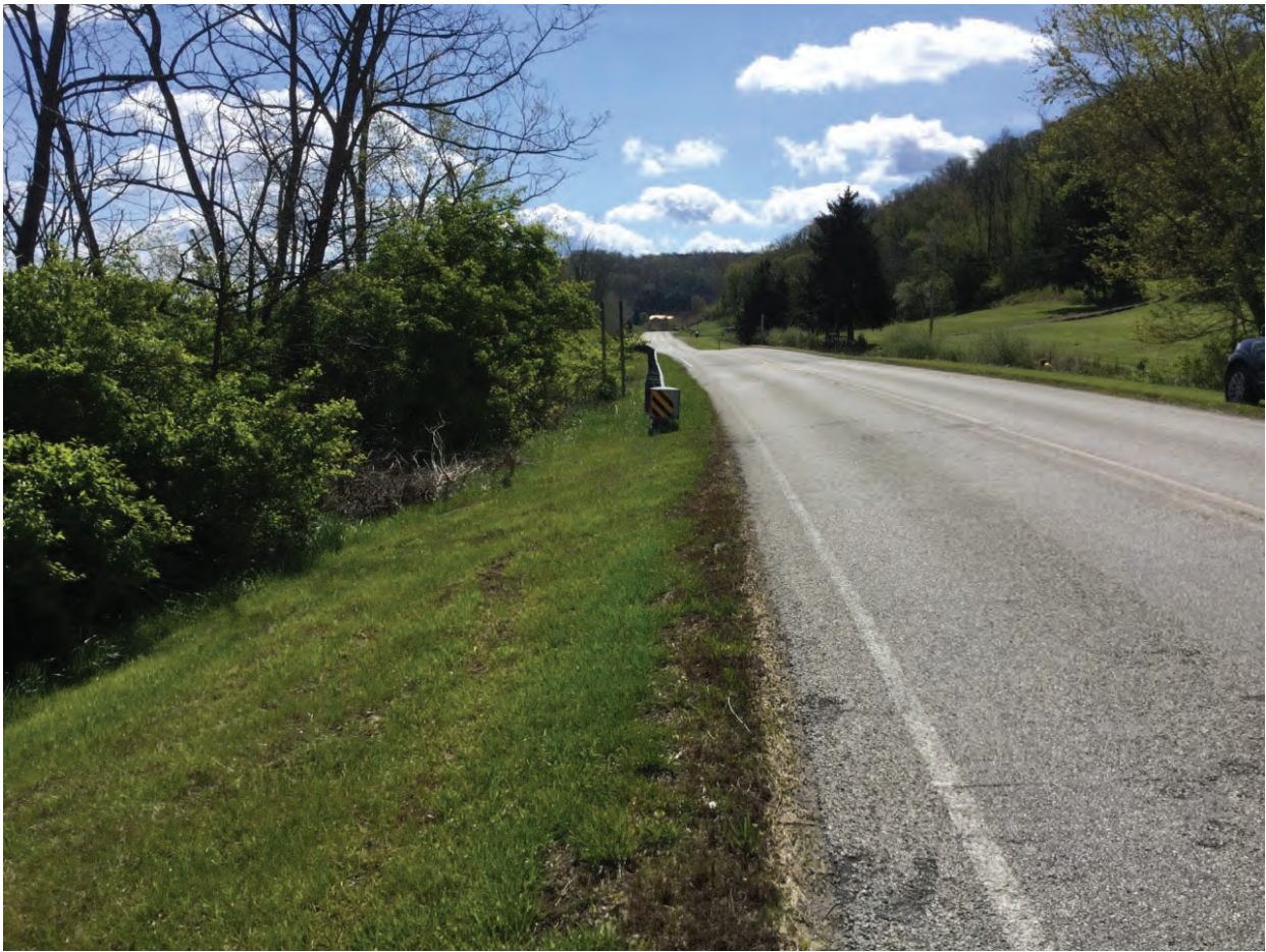
1. Looking southeast along State Road 156 – 4/21/2020
