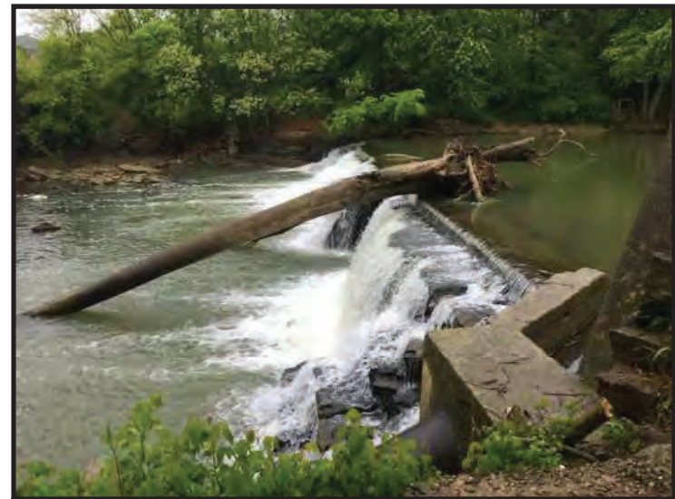
40. View of dam in Silver Creek from southern bank of Silver Creek, looking north. (Taken 5/14/2020)
