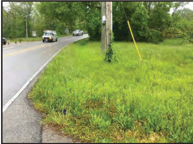
91. View of Blackiston Mill Rd ROW, looking northwest. (Taken 5/14/2020)
