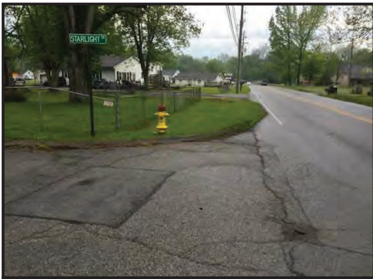
109. View of Blackiston Mill Rd ROW from intersection of Starlight Dr and Blackiston Mill Rd intersection, looking northwest.
