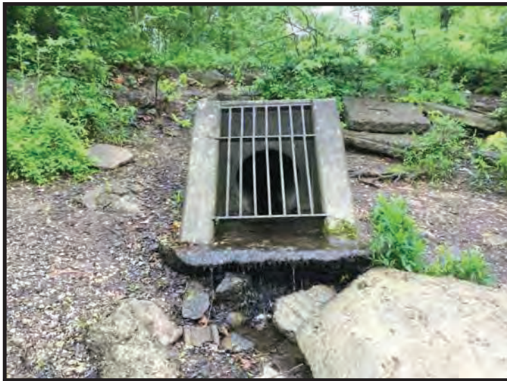
39. View of CV 3, looking southeast. (Taken 5/14/2020)
