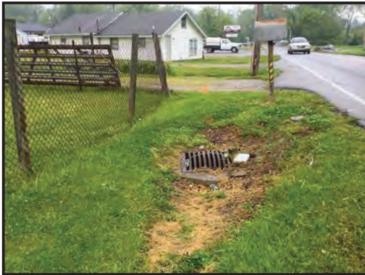
103. View of SD 5 and Blackiston Mill Rd ROW, looking northwest. (Taken 5/14/2020)
