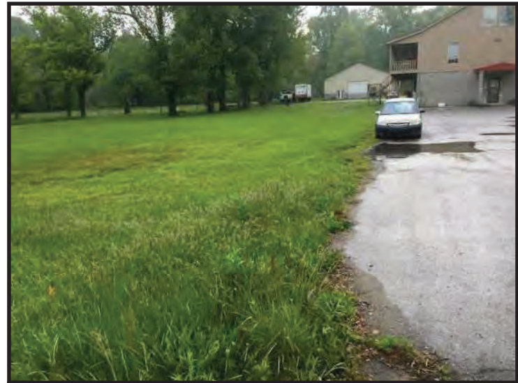
94. View of Blackiston Mill Rd ROW and upland area, looking east. (Taken 5/14/2020)
