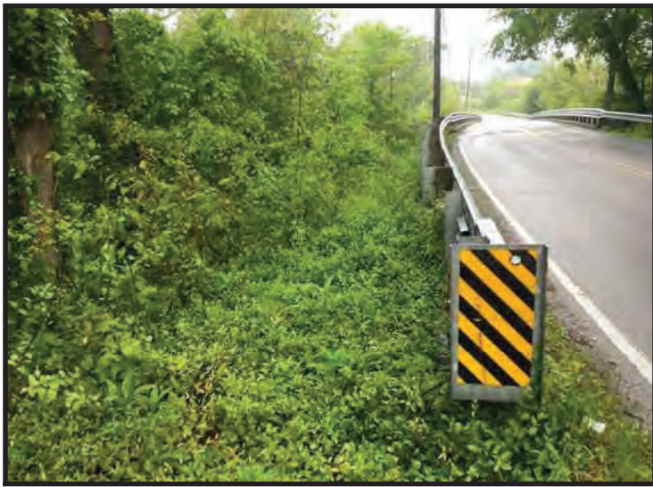
89. View of Blackiston Mill Rd ROW, looking northwest. (Taken 5/14/2020)
