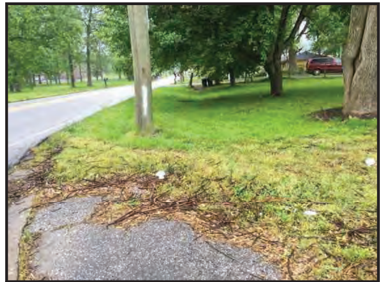
110. View of Blackiston Mill Rd ROW from intersection of Starlight Dr. and Blackiston Mill Rd intersection, looking southeast. (Taken 5/14/2020)
