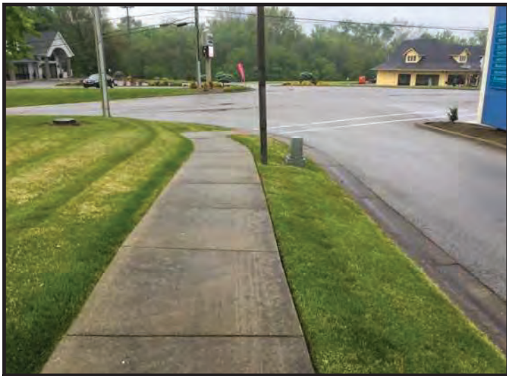
77. View of Blackiston Blvd ROW from northern PSL, looking southwest. (Taken 5/14/2020)
