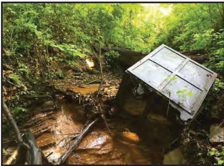
53. View of UNT 1 to Silver Creek, looking northwest (upstream). (Taken 5/14/2020)
