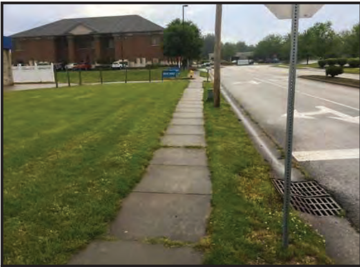
73. View of Blackiston Blvd ROW from intersection of Blackiston Mill Rd and Blackiston Blvd, looking northeast. (Taken 5/14/2020)
