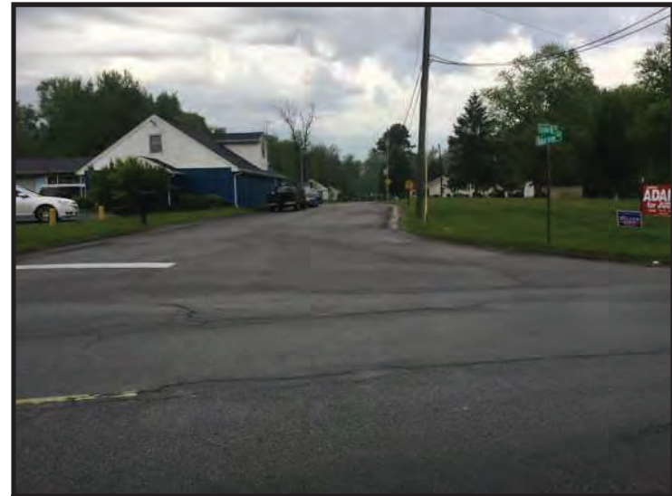
96. View of intersection of Walnut Grove and Blackiston Mill Rd, looking southwest. (Taken 5/14/2020)
