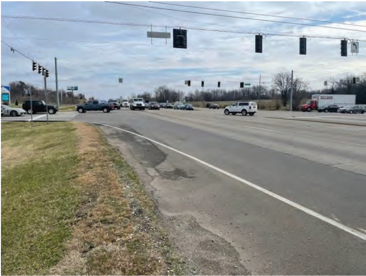
5. Looking east at SR 66/Epworth Rd intersection (12/29/21)
