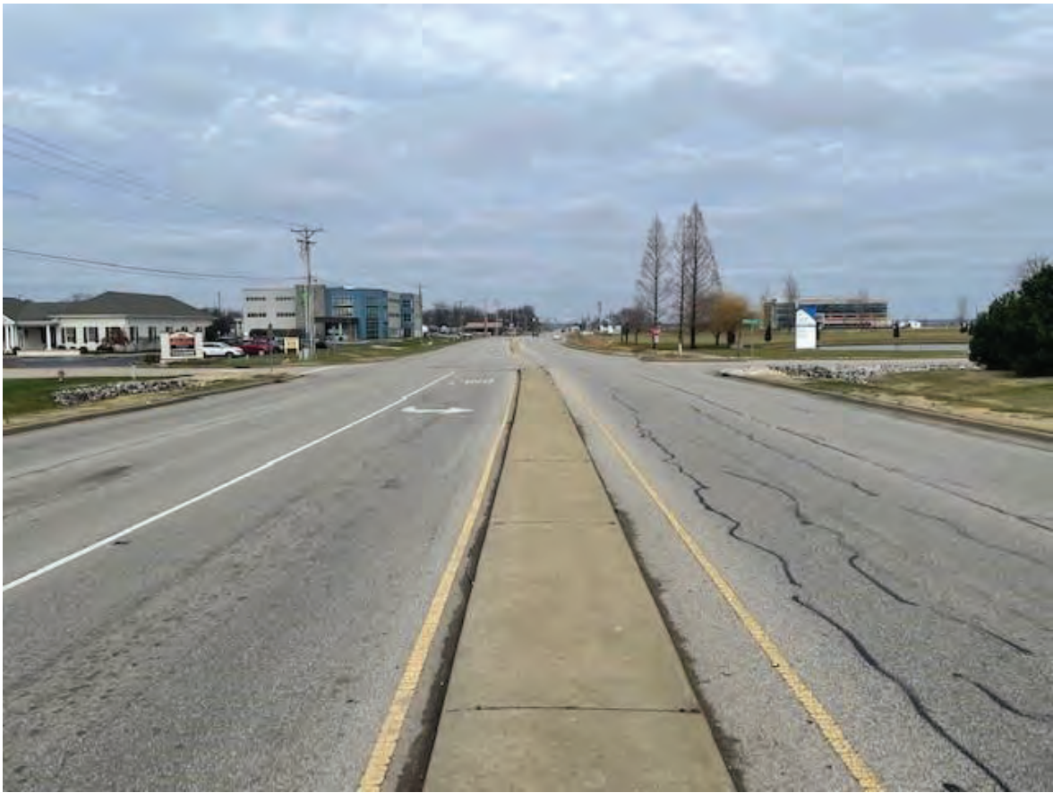
11. Looking north along Epworth Rd (12/29/21)
