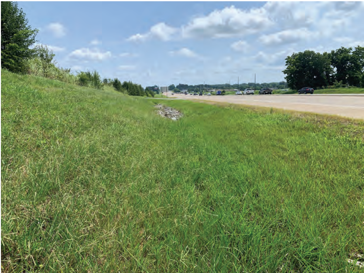
18. Looking east along westbound SR 66 (08/10/21)
