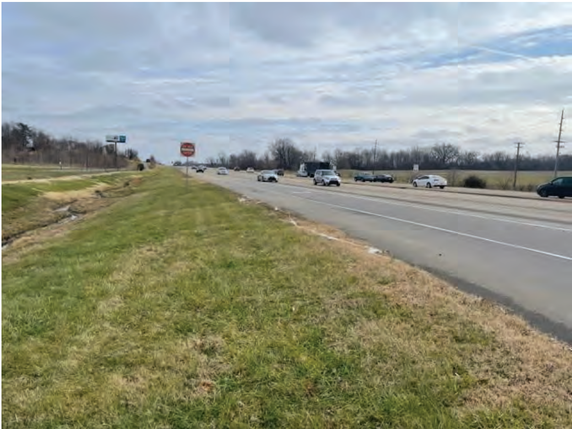
16. Looking east along westbound SR 66 (12/29/21)
