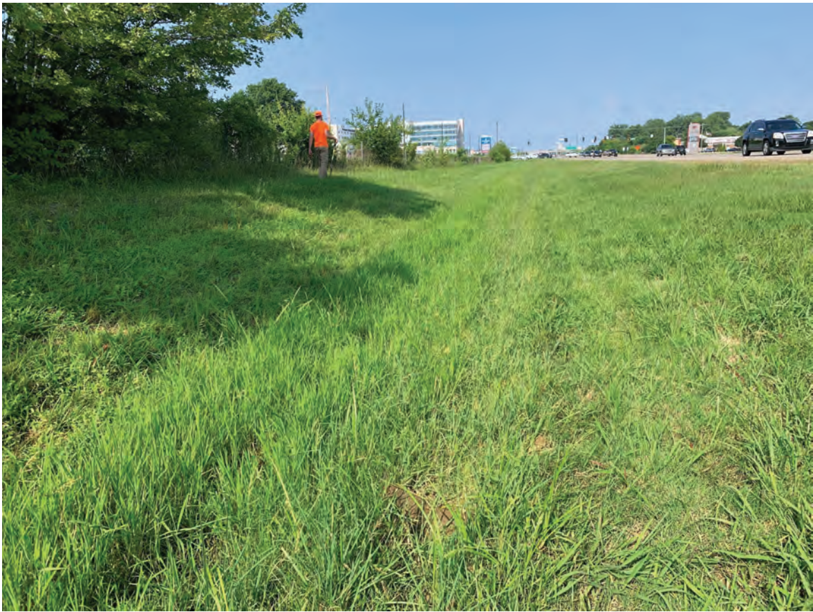
17. Looking west along eastbound SR 66 (08/10/21)
