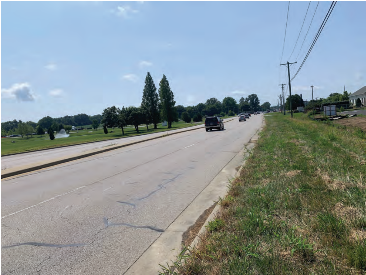
12. Looking southeast along Epworth Rd from northern project limits (08/10/21)
