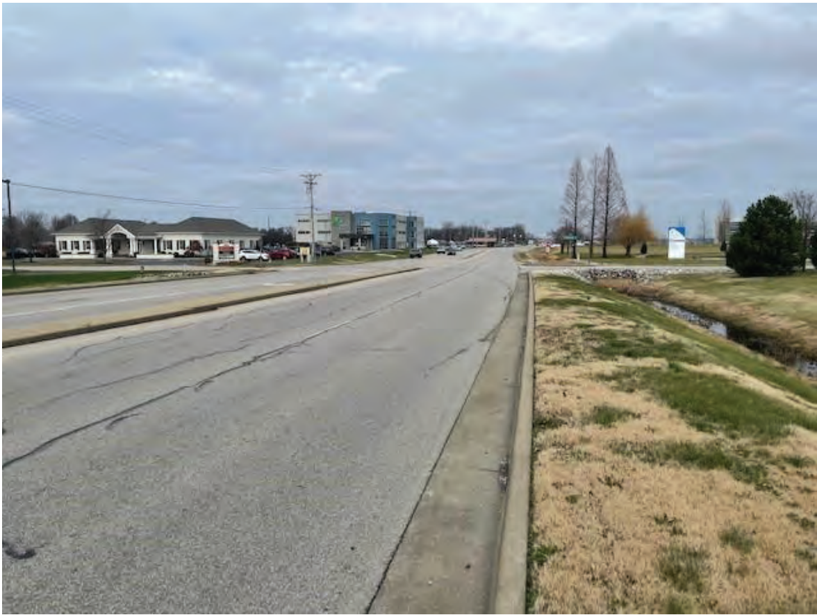
9. Looking north along Epworth Rd (12/29/21)
