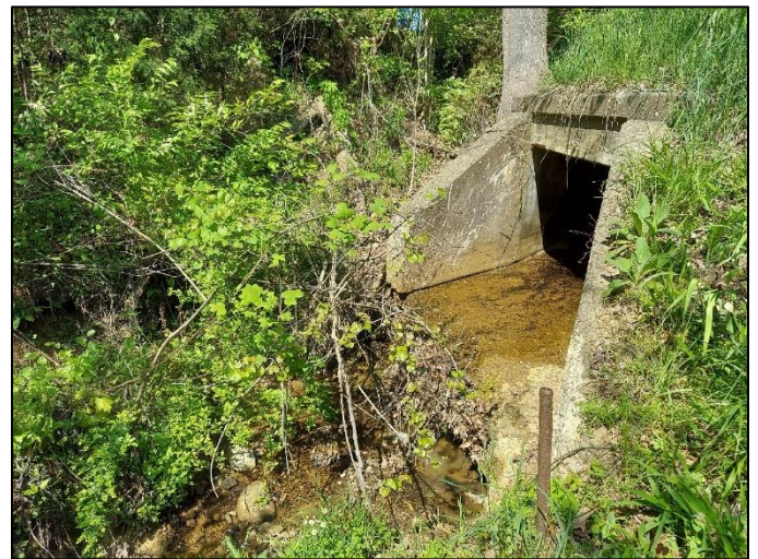
Photo 12. Outlet of culvert (CV 445-28-000.52) and UNT to Beech Creek, viewing west, 5/13/2022
