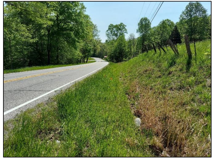
Photo 6. Roadside ditch on south side of SR 445, viewing east, 5/13/2022
