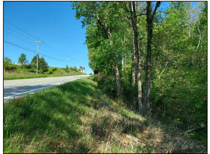
Photo 4. Roadside slope on north side of SR 445, viewing west, 5/13/2022
