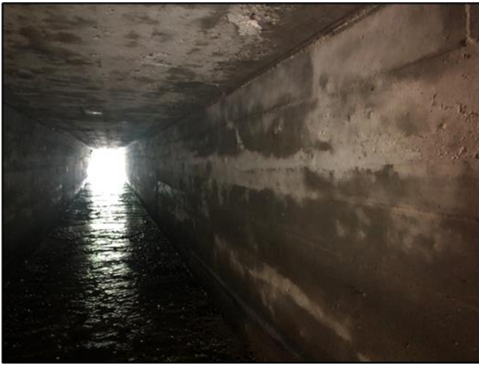
Photo 13. Inside of culvert (CV 445-28-000.52) at outlet facing upstream, viewing northwest, 5/13/2022
