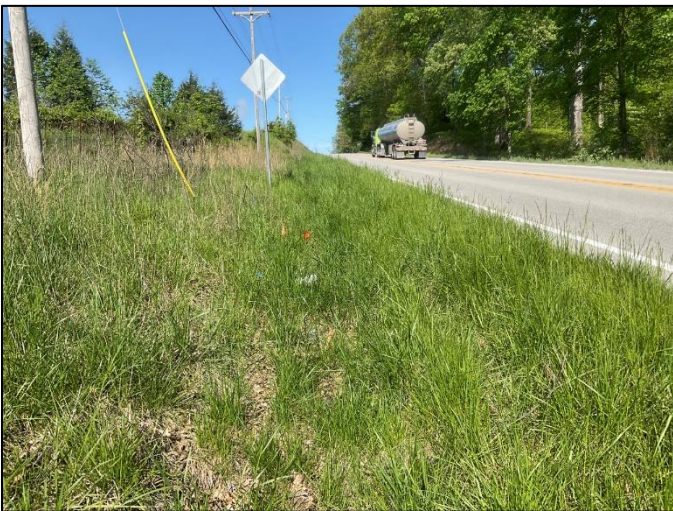
Photo 3. Roadside ditch on south side of SR 445, viewing west, 5/13/2022
