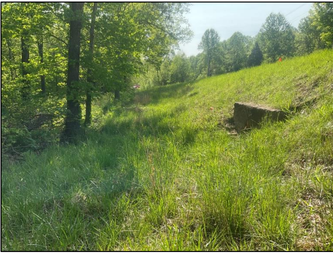
Photo 5. Roadside slope on north side of SR 445, viewing southeast, 5/13/2022
