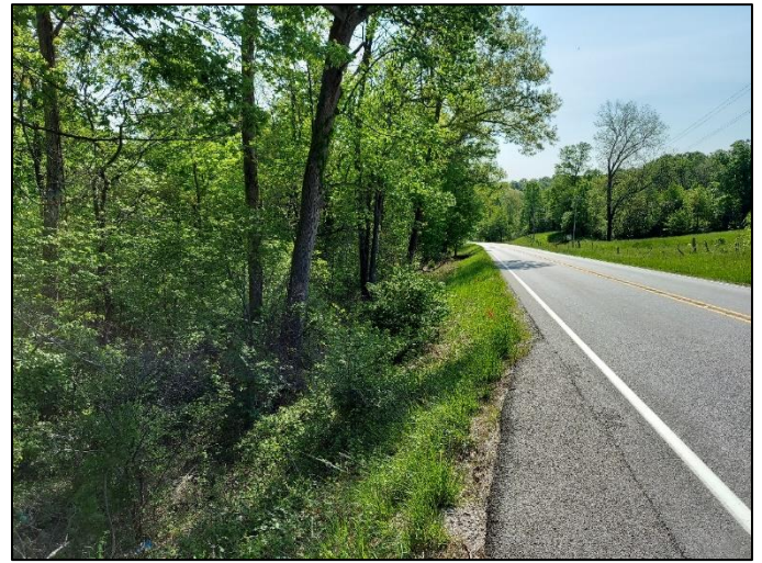
Photo 2. Roadside slope on north side of SR 445, viewing east, 5/13/2022
