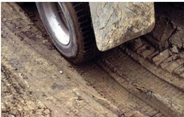
Figure 10-3 Unacceptable Compaction
