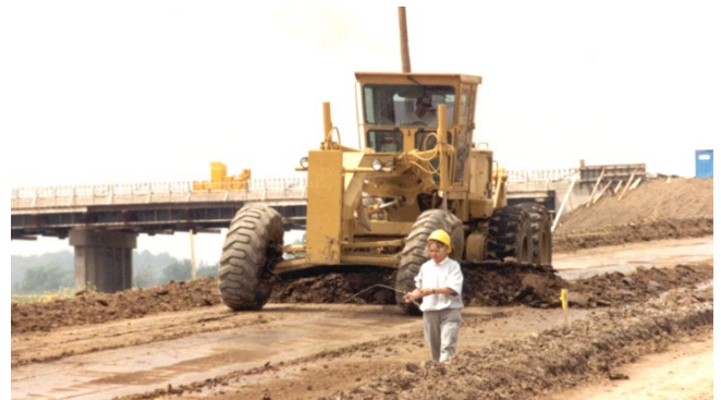
Figure 7-2 Fine Grading
