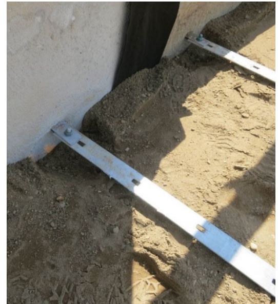
Figure 10-7 Proper Strap Attachment
