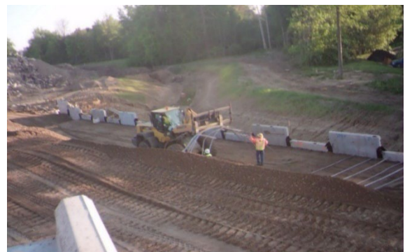
Figure 10-8 Reinforcement Strap Installation
