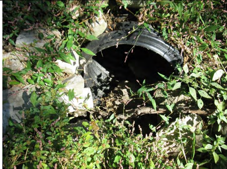
16. Culvert inlet under SR 65 draining to RSD 4. (10-9-19)
