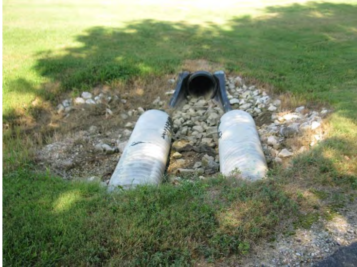
43. Looking northwest at culverts draining RSD 7 located on cemetery property. (9/17/19)
