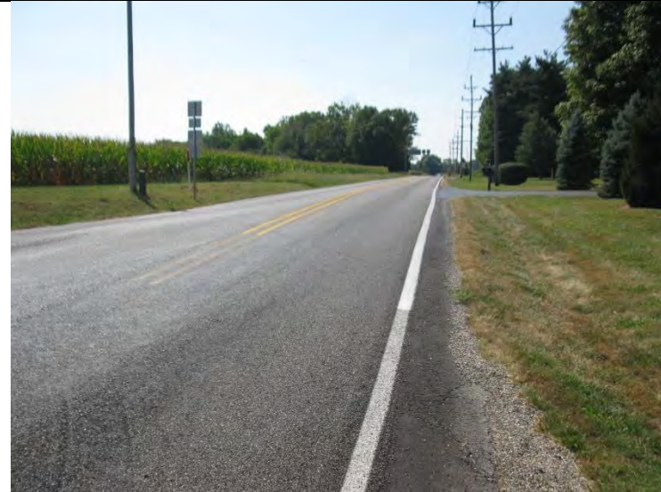
52. Looking south along SR 65/68 from north terminus. (9/17/19)
