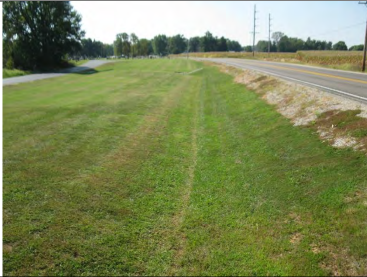
45. Looking south along SR 65/68 and RSD 8 on east side of SR 65/68 near cemetery exit. (9/17/19)
