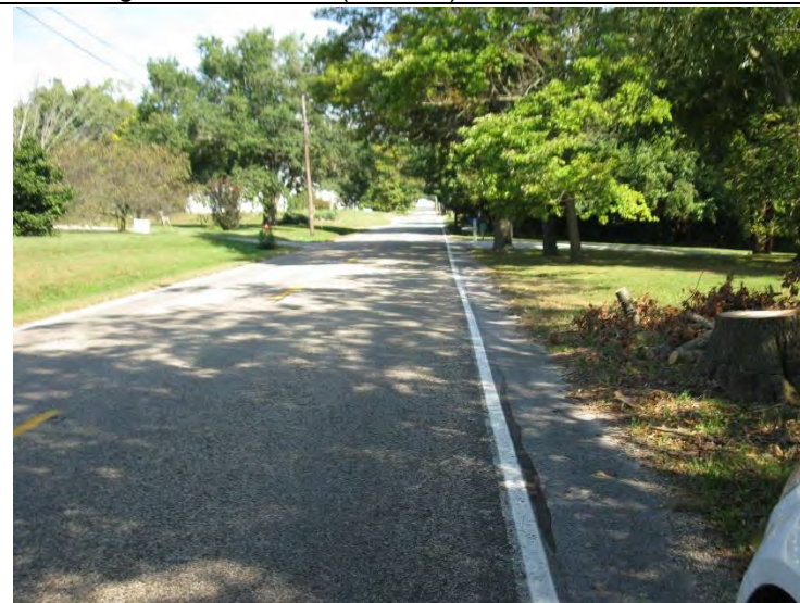
20. Looking north along SR 65, just south of the 9925 Evansville Street driveway. (9/17/19)
