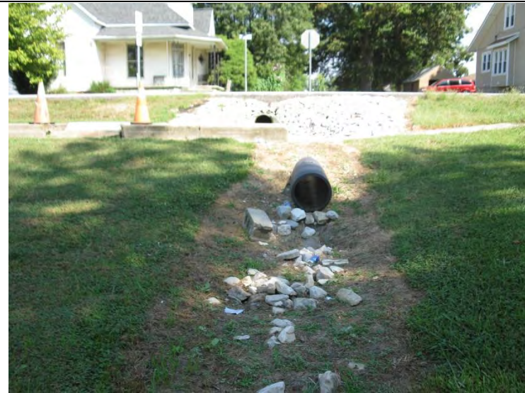
34. Looking north in RSD 5 near Green Street. (9/17/19)
