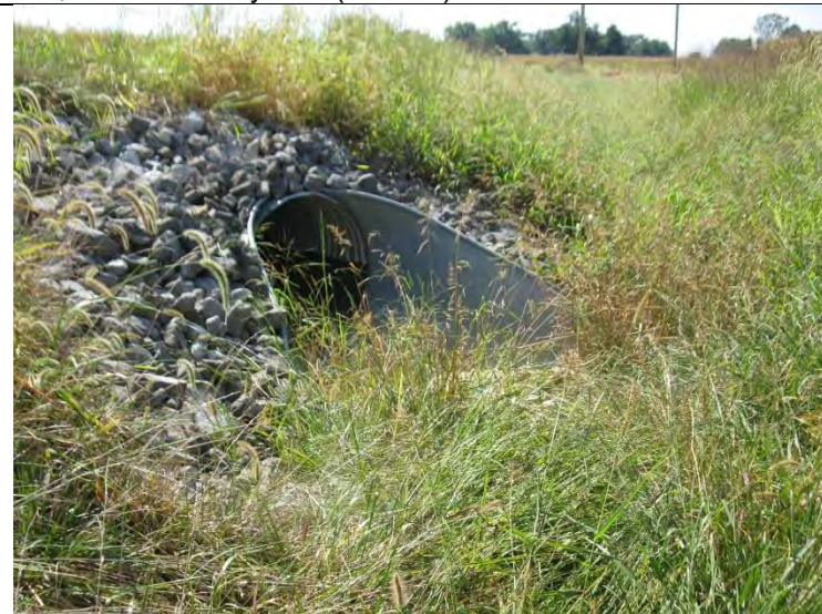
48. Looking at culvert along west side of SR 65/68 and RSD 7. (9/17/19)
