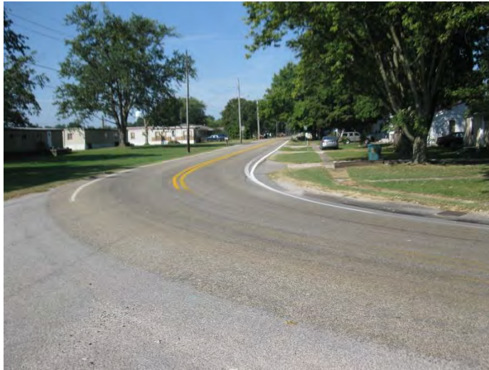
37. Looking west along SR 65/68, near the intersection of SR 65/68 and North Street. (9/17/19)
