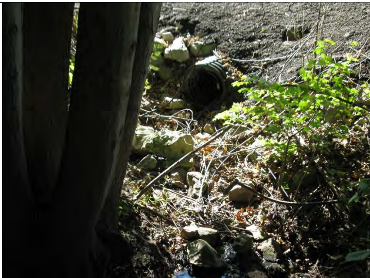
17. Culvert outlet from under SR 65 draining to RSD 4. (10-9-19)
