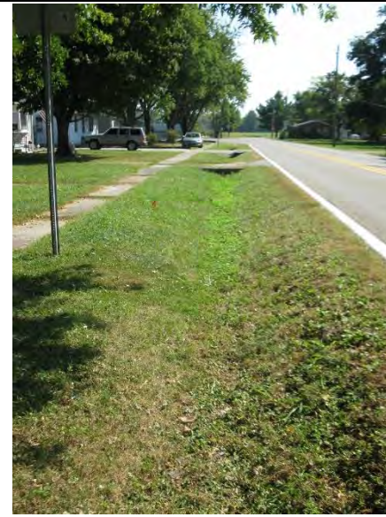
36. Looking east along SR 65/68, and RSD 6 east of Garfield Street. (9/17/19)
