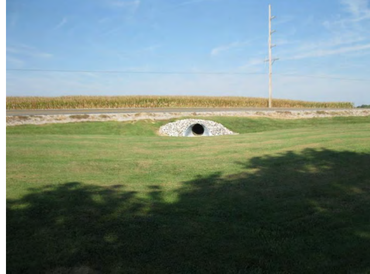
44. Looking northwest from cemetery at culvert draining RSD 7 located under the SR 65/68. (9/17/19)
