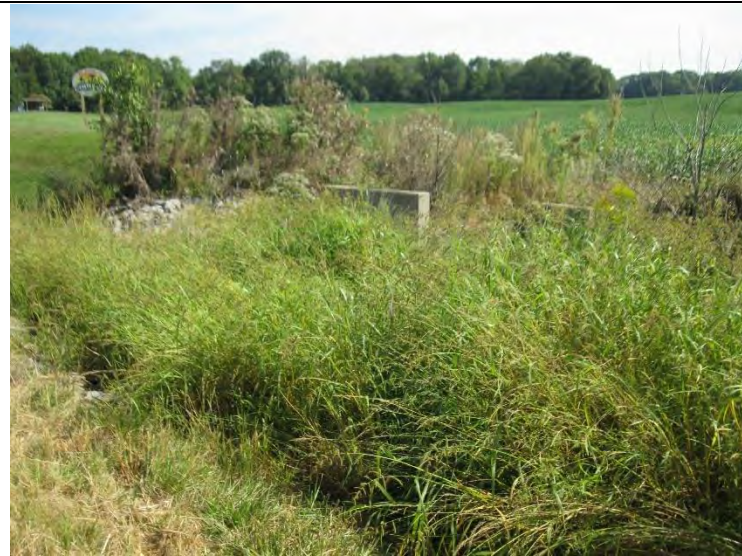
6. Looking northeast at culvert and Wetland 1, east of SR 65, near south terminus. (9/17/19)
