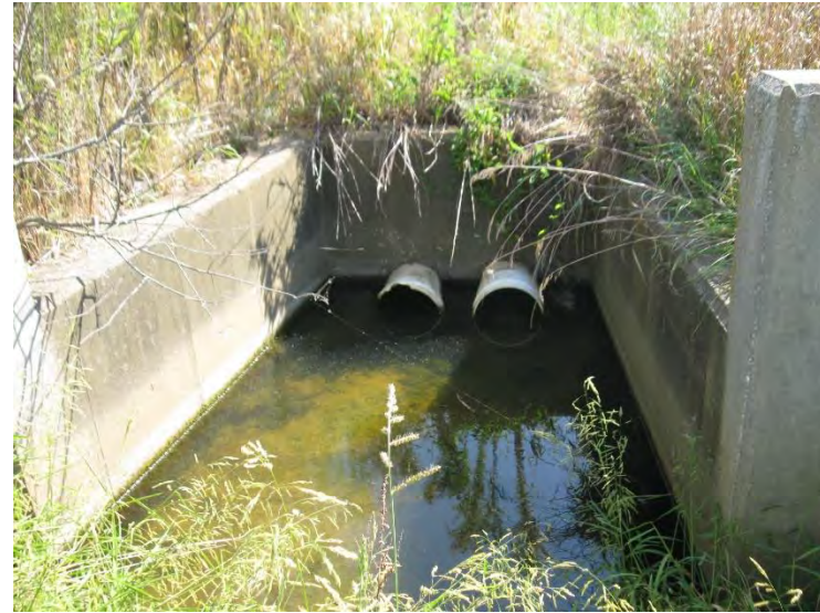
2. Looking east at culverts draining agricultural field near Wetland 1, east of SR 65, near south terminus. (9/17/19)
