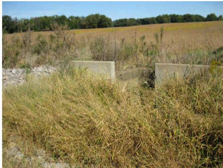
3. Looking east, east of SR 65, culvert outlet near Wetland 1 at edge of agricultural field near south terminus. (10-9-19)
