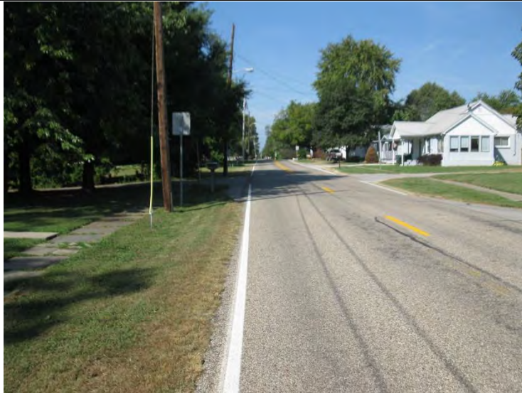
31. Looking west down SR 65/68 at the intersection of East Street. (9/17/19)
