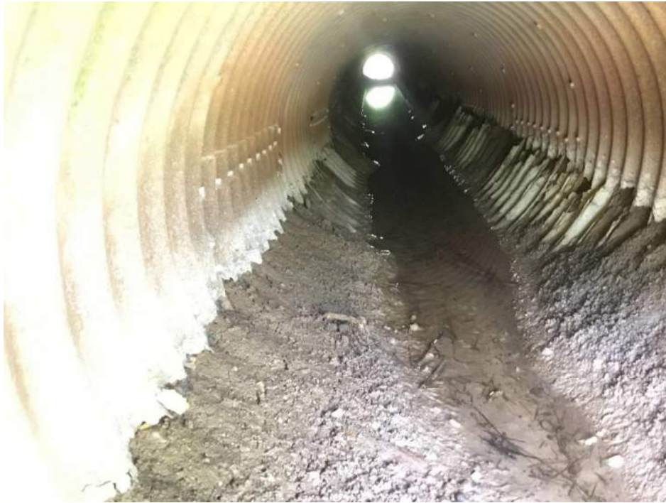
PHOTO 7 Condition Description Looking south through west pipe
