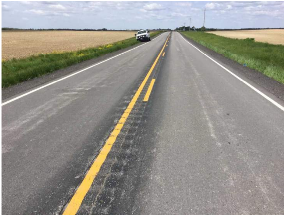
PHOTO 2 Condition Description Road alignment looking west
