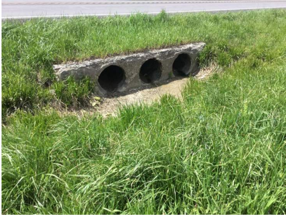
PHOTO 5 Elevation, Condition Description Profile looking south
