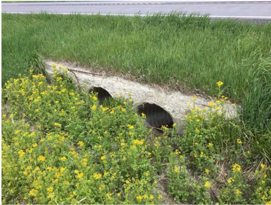
PHOTO 4 Elevation, Condition Description Profile looking North
