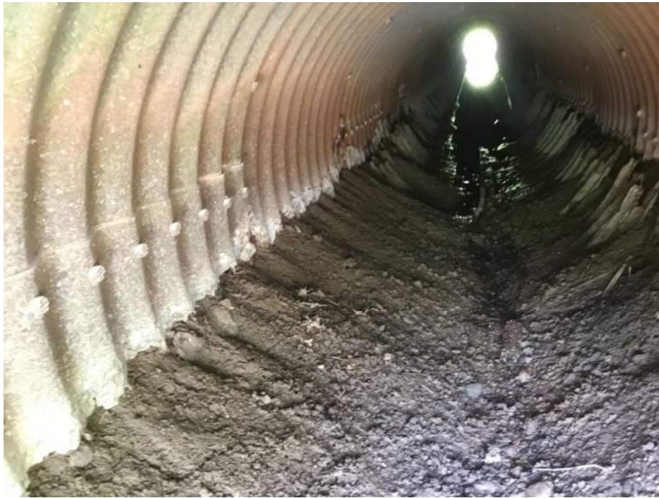
PHOTO 8 Condition Description Looking South through East pipe
