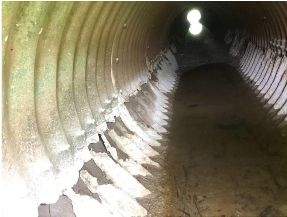
PHOTO 10 Condition Description Looking North through West pipe
