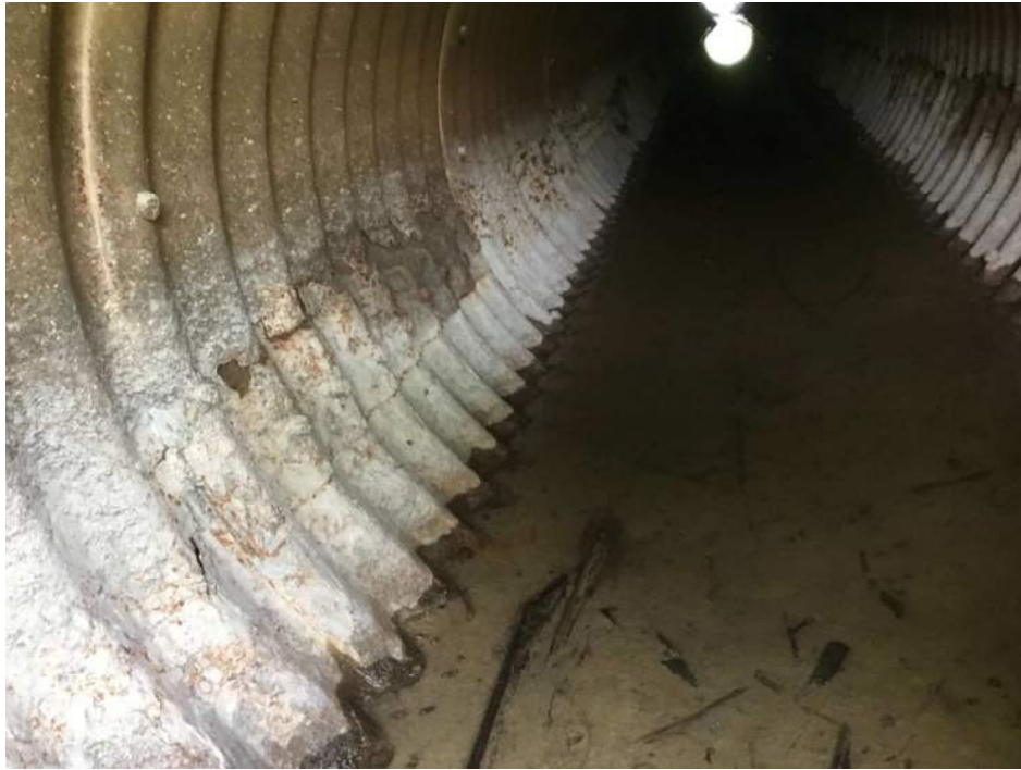
PHOTO 11 Condition Description Looking North through East pipe
