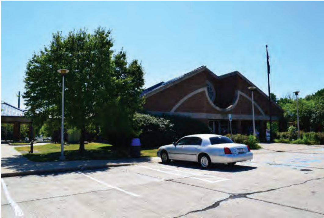
Photo 14. View of the Clear Creek Rest Area west facade facing southeast from the Clear Creek Rest Area parking lot
