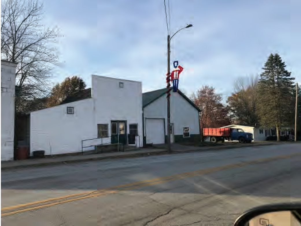
21. Looking north on SR 26 at intersection of SR 26 and SR 55
