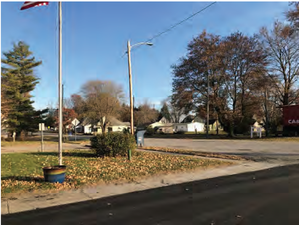
18. Looking east at SR 26 from Jefferson Street
