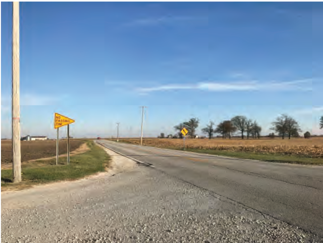
14. Looking east on SR 26 from 450 E
