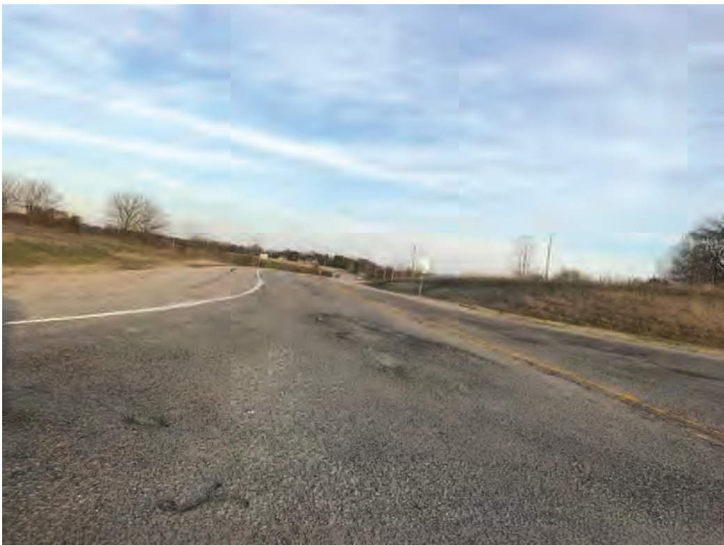
28. Looking west at SR 26 from US 41
