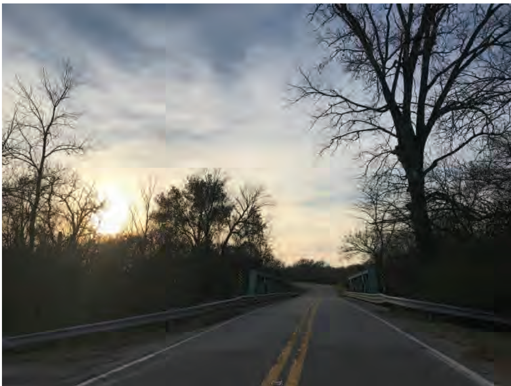
26. Looking west at State Highway Bridge 026-85-1572
