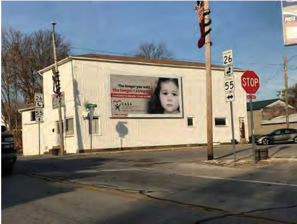
19. NC building at intersection of SR 26 and SR 55
